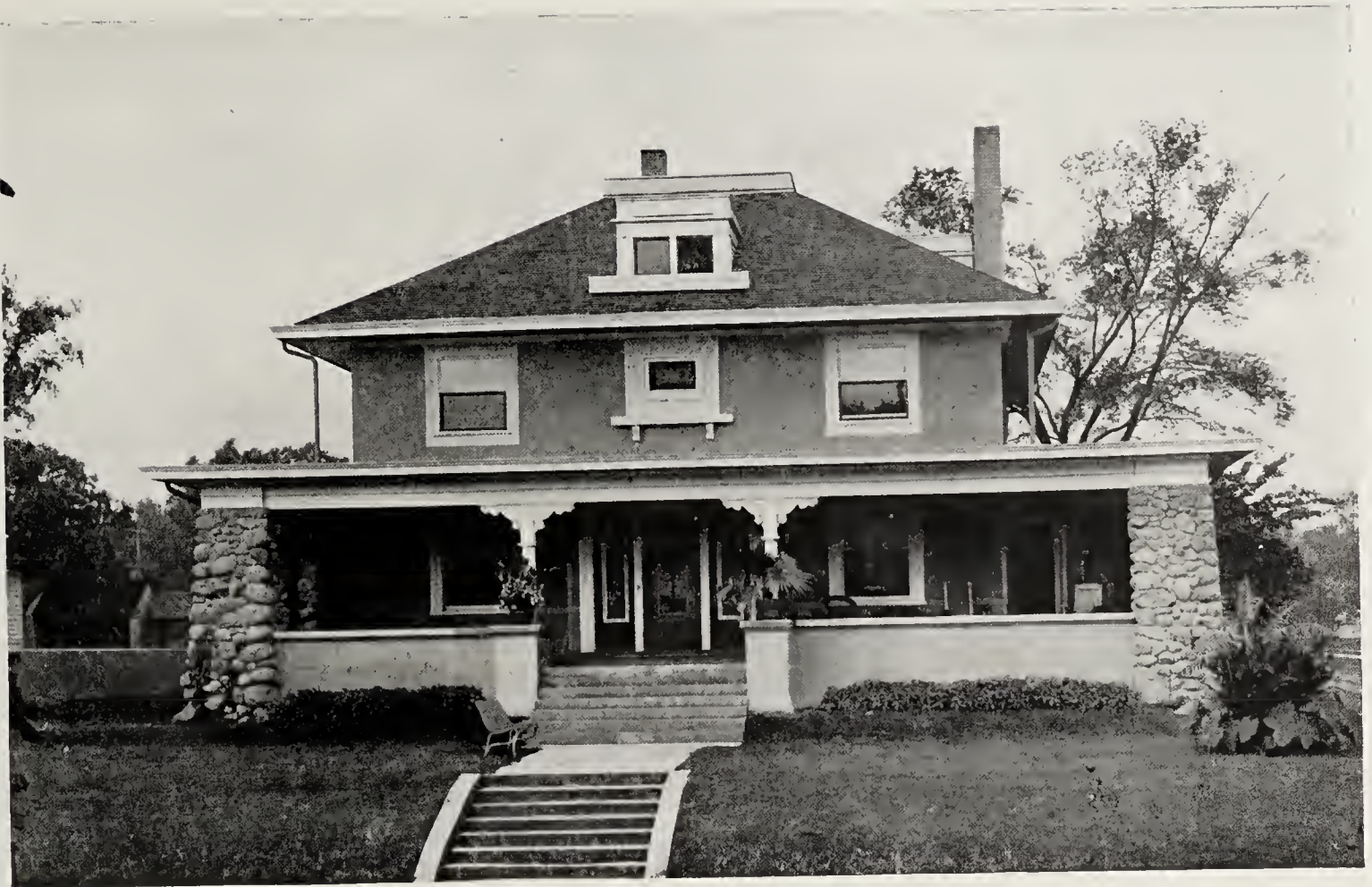
CHANCELLOR'S RESIDENCE, DRAKE UNIVERSITY, DES MOINES, IOWA—See Floor Plans. The C. E. Eastman Co., Architects, Des Moines.
