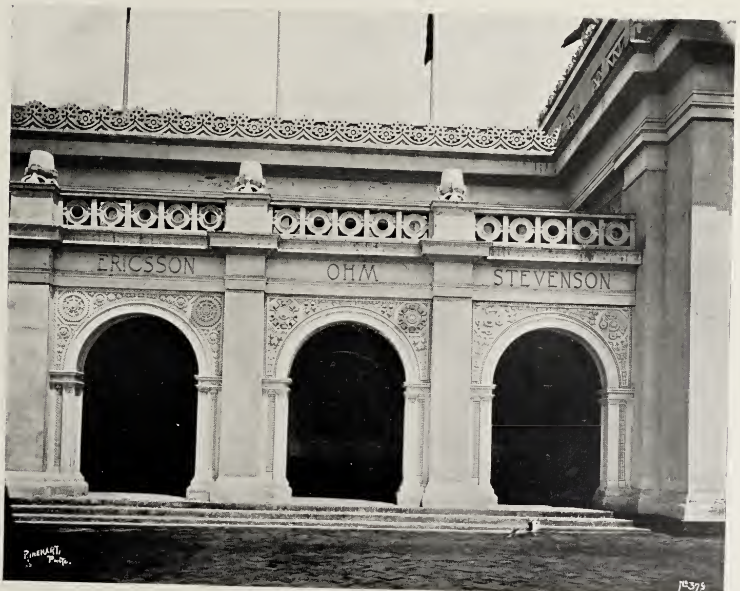
DETAIL OF PORTICO, MACHINERY AND ELECTRICAL BUILDING,
