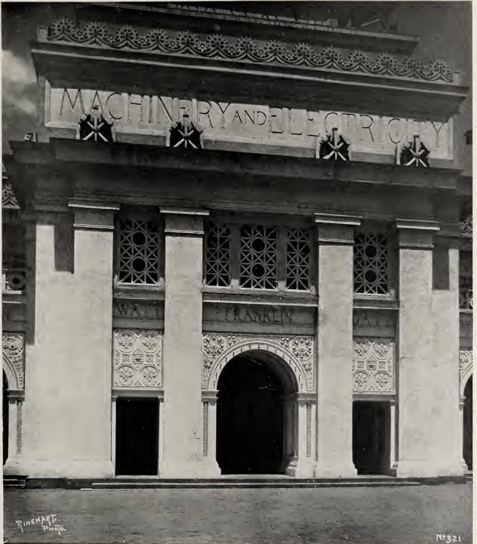
MAIN ENTRANCE TO MACHINERY AND ELECTRICAL BUILDING, Trans Mississippi Exposition, Omaha, Neb., 1900-01 Dwight Heald Perkins, Architect, Chicago.
