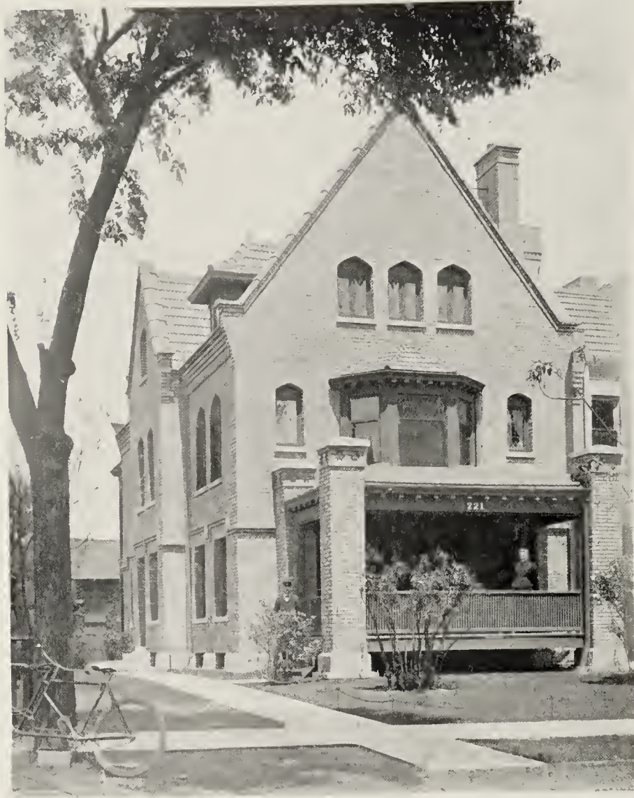
FRONT VIEW OF JAMES J. WAIT ESQ'S RESIDENCE, CHICAGO, ILL. Dwight Heald Perkins, Architect, Chicago.
