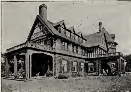
Shepley, Rutan & Coolidge, Arch'ts, Boston.
