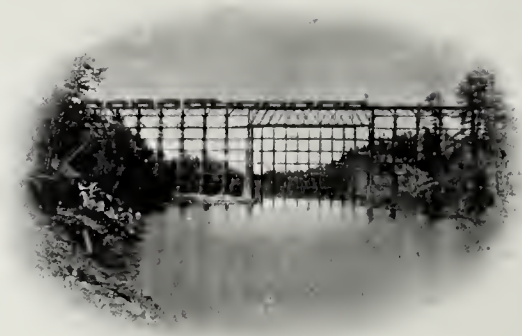
RAILROAD BRIDGE, Piers Built of Kettle River Sandstone.
