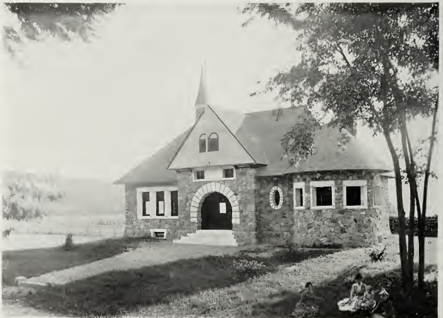
FARWELL SCHOOL HOUSE, Charlestown, N. H. (See Description on Page 21.)
