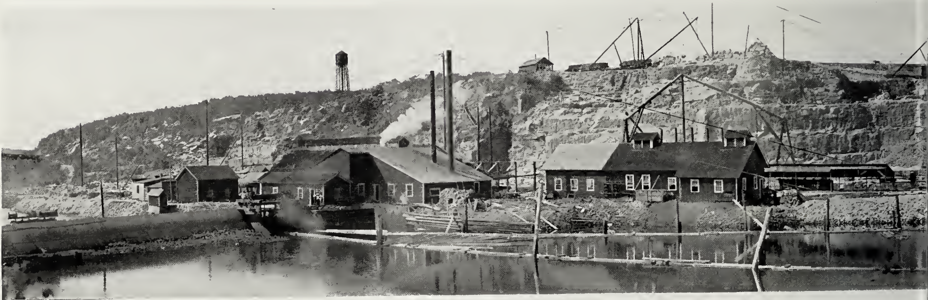
GENERAL VIEW OF KETTLE RIVER
