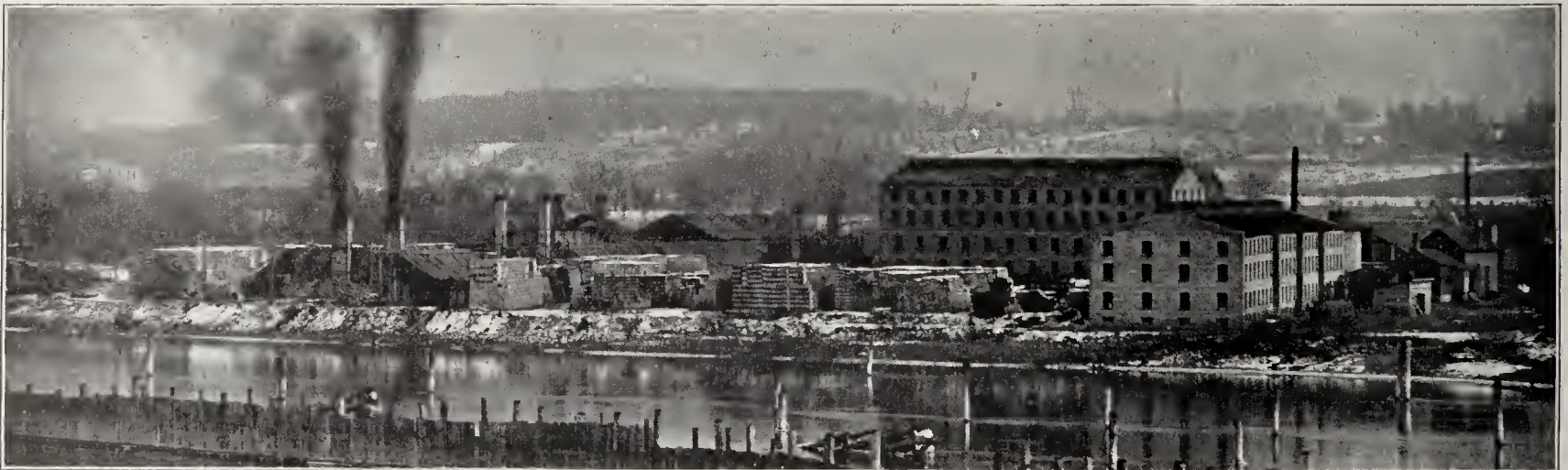
VIEW OF NORTHWESTERN FIRE PROOFING WORKS, MINNEAPOLIS.
