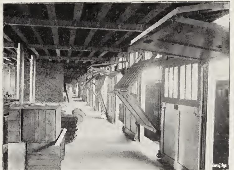
In the Lake Shore & Michigan Southern Freight House there are 129 door openings, 9 ft. wide by 10 ft. high.
