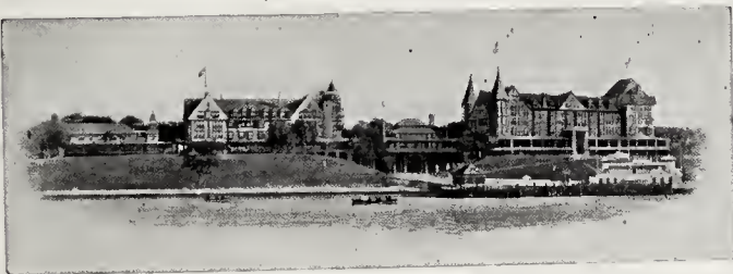
Manhasset House, Shelter Island, N. Y. using 1000-light plant.
