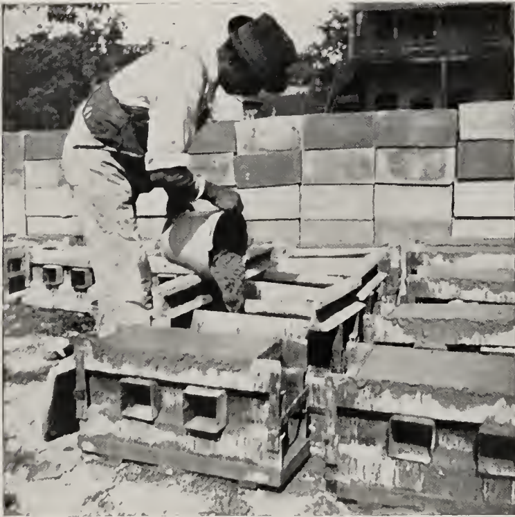
POURING THE STONE.
