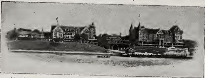
Manhasset House, Shelter Island, N. Y. using 1000-light plant.
