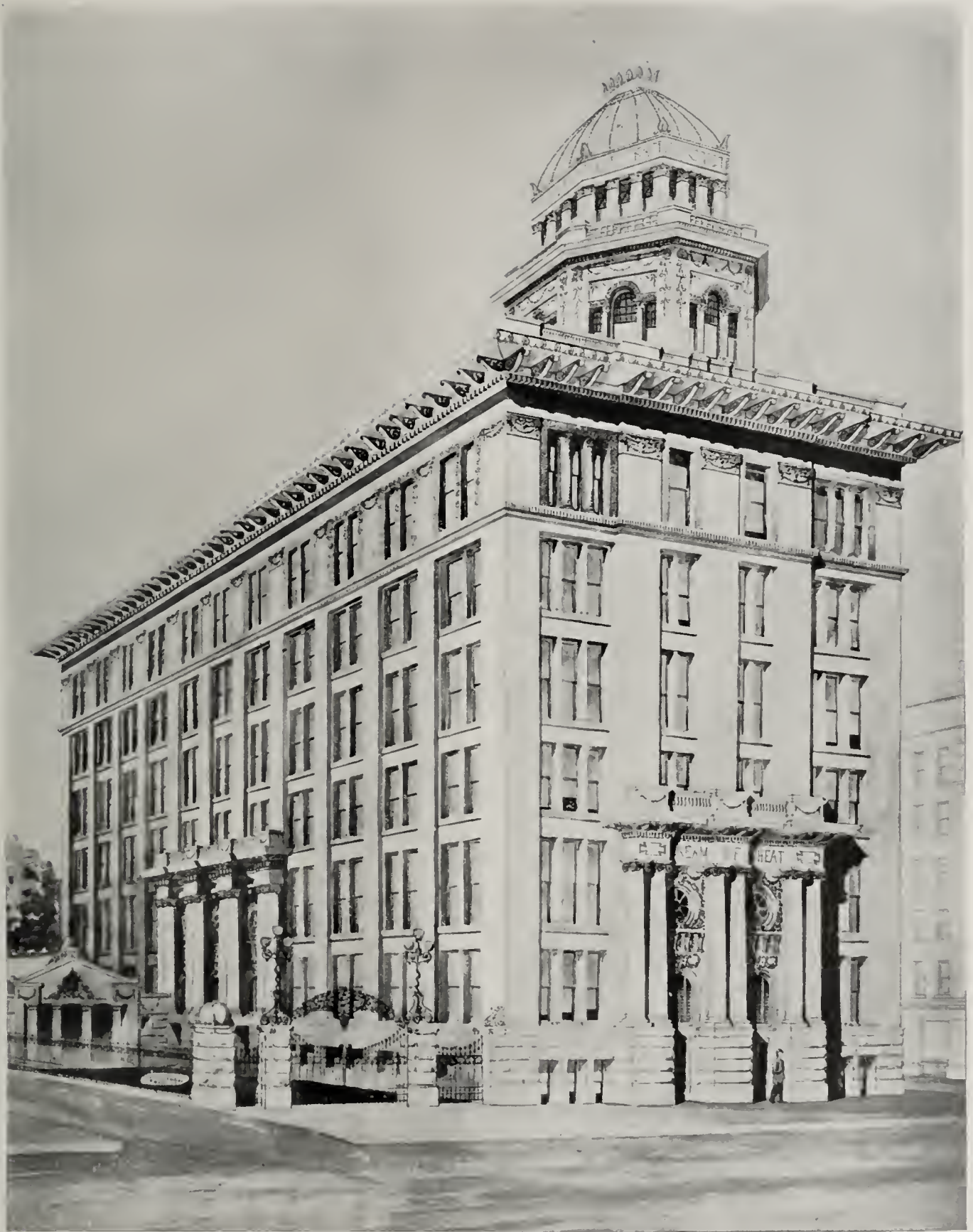
A COMPETITIVE DESIGN FOR THE "CREAM OF WHEAT" BUILDING, MINNEAPOLIS. Sedgwick & Saxton, Architects, Minneapolis.
