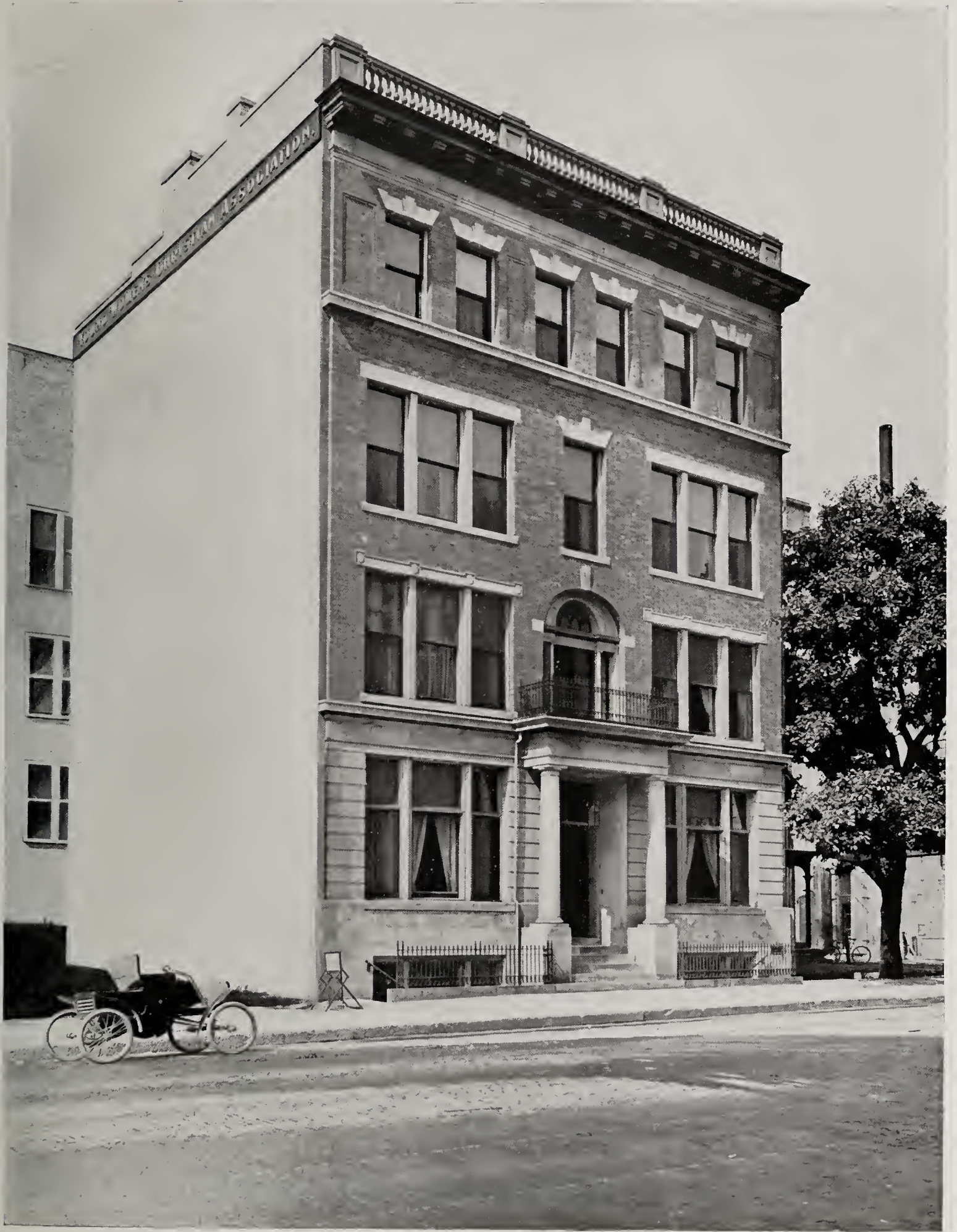
YOUNG WOMEN'S CHRISTIAN ASSOCIATION BUILDING, MINNEAPOLIS, MINN. Wm. Channing Whitney, Architect, Minneapolis.
