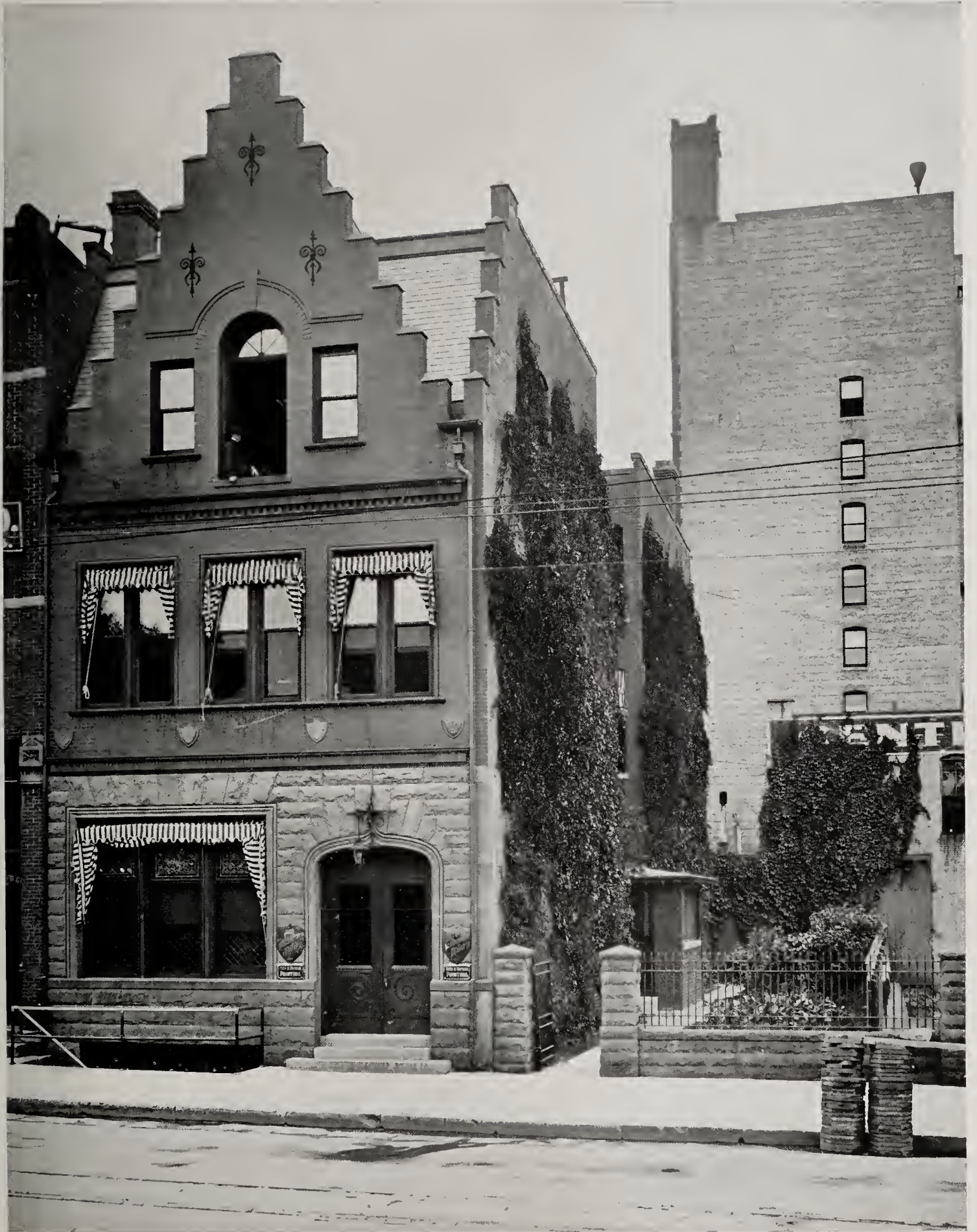
THE NORTHWESTERN MILLER BUILDING, MINNEAPOLIS, MINN. Wm. Channing Whitney, Architect, Minneapolis.
