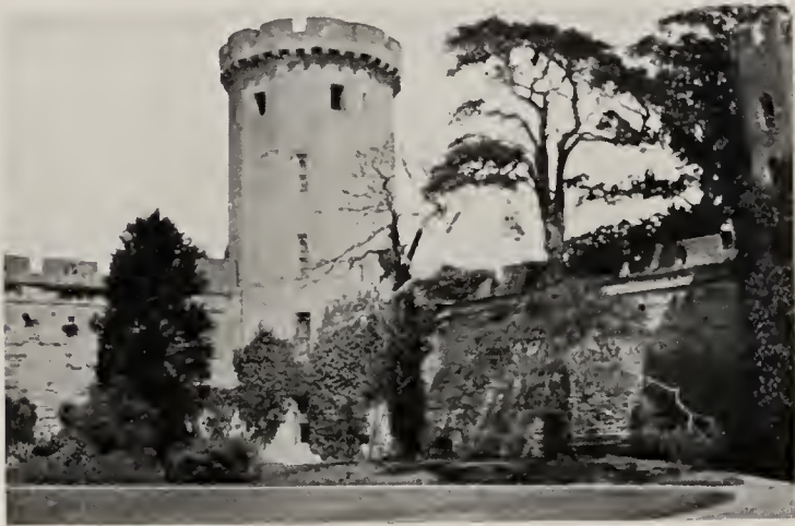
*GUY'S TOWER, WARWICK CASTLE.
