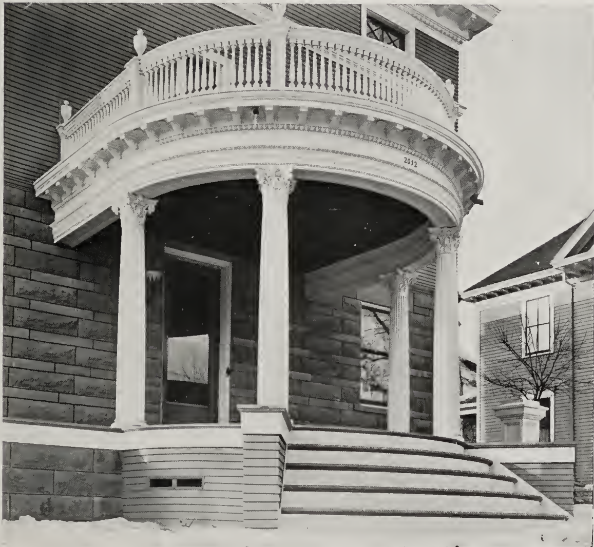
DETAIL OF FRONT PORCH TO RESIDENCE OF HAROLD JOHNSON, MINNEAPOLIS, MINN. F. D. Orff, Architect, Minneapolis.
