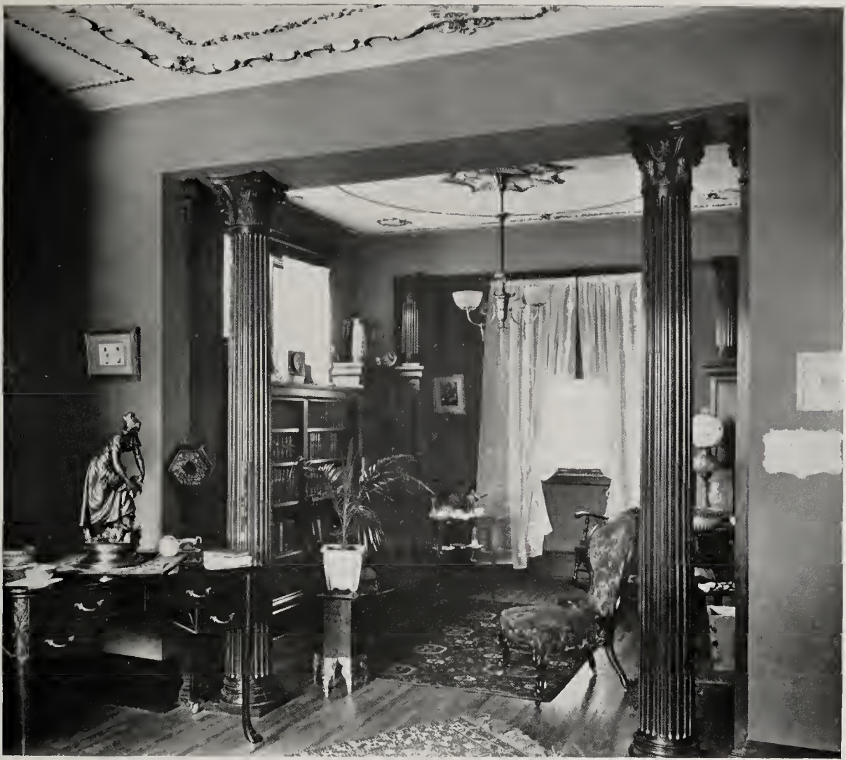
PARLOR IN RESIDENCE OF HAROLD JOHNSON, MINNEAPOLIS, MINN. F. D. Orff, Architect, Minneapolis.
