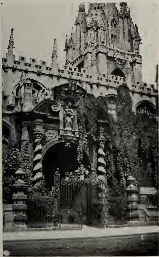
*VIRGIN'S PORCH—ENTRANCE TO ST. MARY'S CH., HIGH ST., OXFORD.
