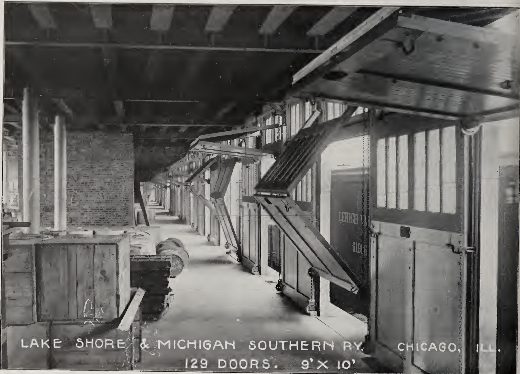
VIEW OF THE CROSS HORIZONTAL FOLDING DOORS In the Lake Shore & Michigan Southern Freight House, Chicago, Ill. Manufactured by the Variety Mfg. Co., Chicago.
