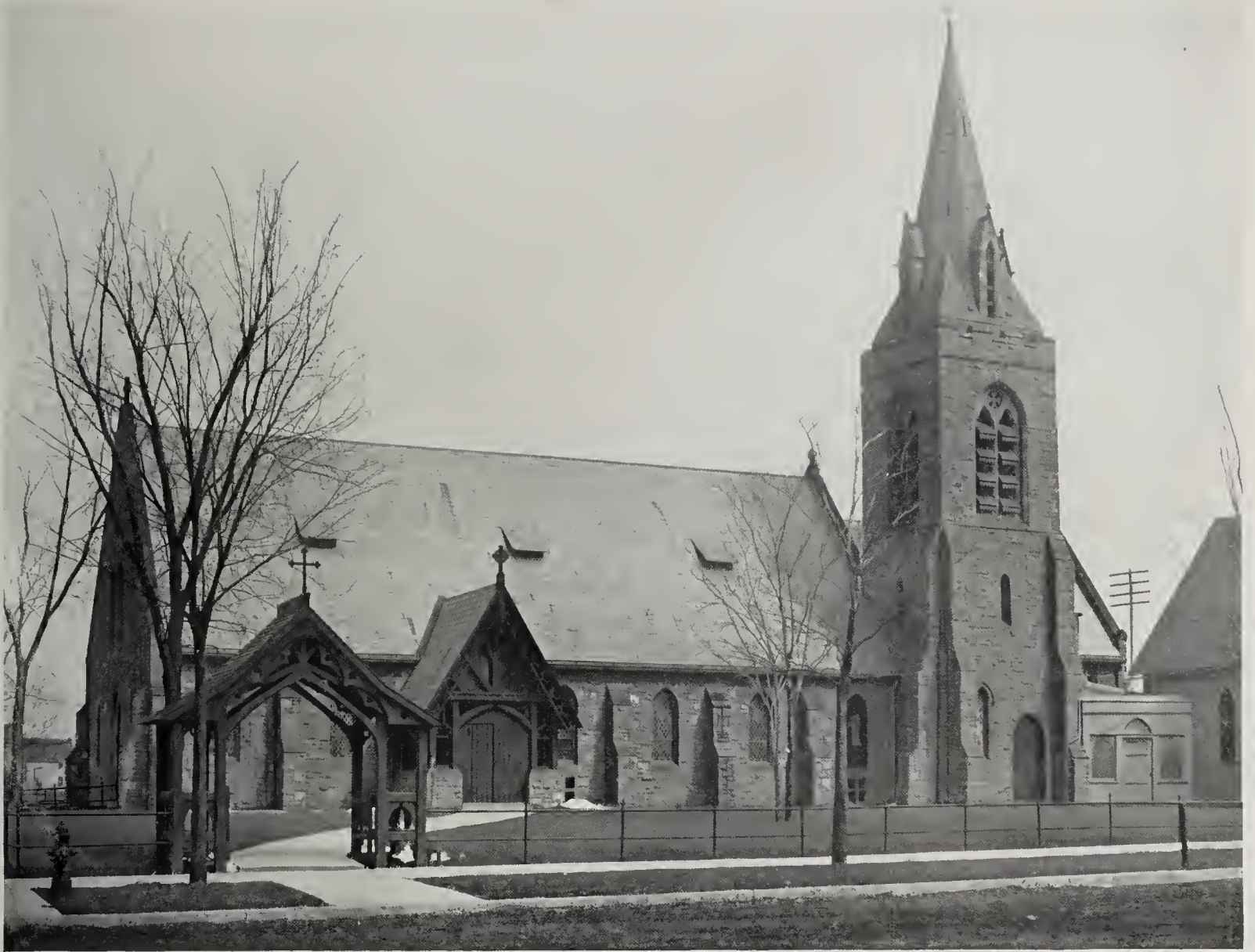
Fig. 3 - ST. CLEMENT'S EPISCOPAL CHURCH, ST. PAUL, MINN. Cass Gilbert, Architect, New York and St. Paul.
