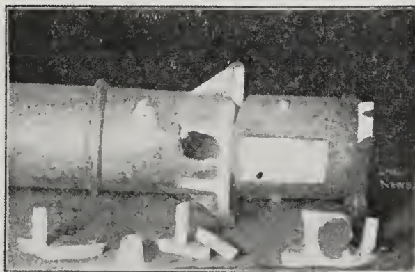
Fig. 14.—Fracture of Brackets, 14-in. Columns, No. 6.
