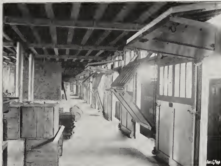
In the Lake Shore & Michigan Southern Freight House there are 129 door openings, 9 ft. wide by 10 ft. high.
