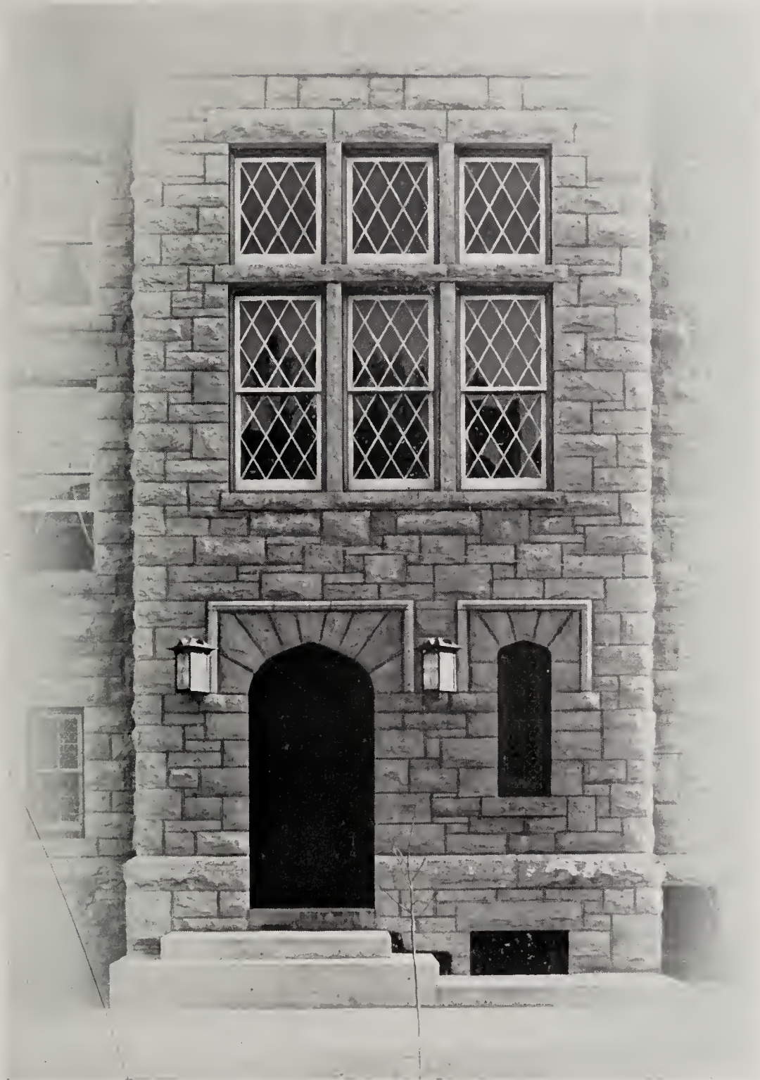
NORTH ENTRANCE TO FRANK T. HEFFELFINGER'S RESIDENCE, MINNEAPOLIS, MINN. Wm. Channing Whitney, Architect, Minneapolis
