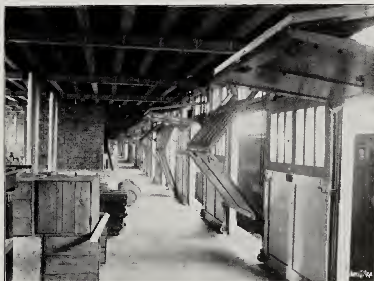
In the Lake Shore & Michigan Southern Freight House there are 129 door openings, 9 ft. wide by 10 ft. high.
