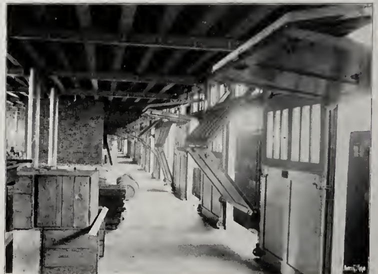
In the Lake Shore & Michigan Southern Freight House there are 129 door openings, 9 ft. wide by 10 ft. high.
