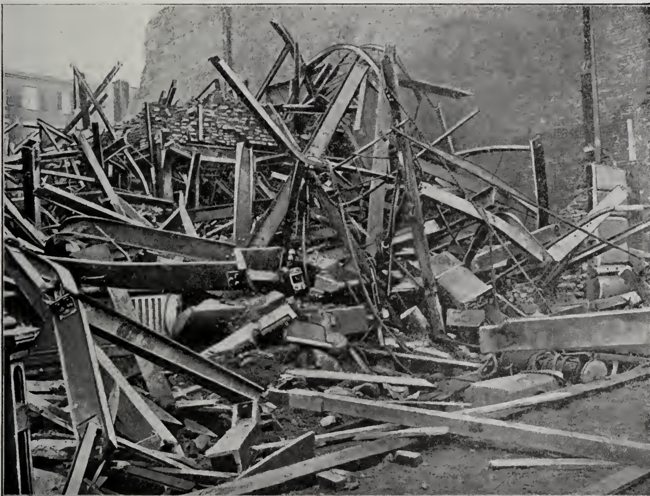
RUINS OF DARLINGTON BUILDING, SHOWING BROKEN CAST IRON COLUMNS. From Carpentry and Building.
