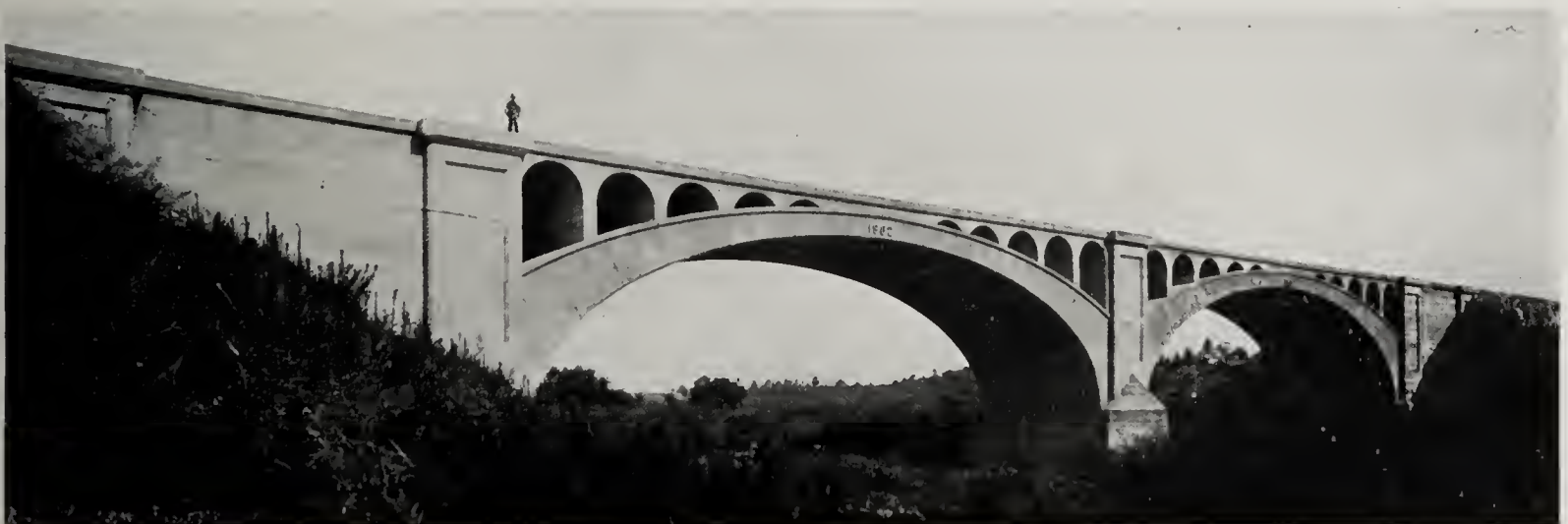
DOUBLE TRACK CONCRETE BRIDGE, ILLINOIS CENTRAL RY. Built with Universal Portland Cement.
