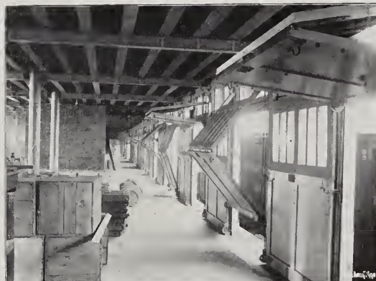
In the Lake Shore & Michigan Southern Freight House there are 129 door openings, 9 ft. wide by 10 ft. high.
