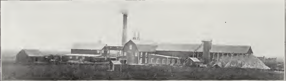
This Cut Represents THE FORT DODGE PLASTER COMPANY'S MILL
