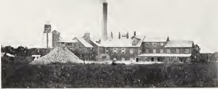
NEW GYPSUM MILL.
