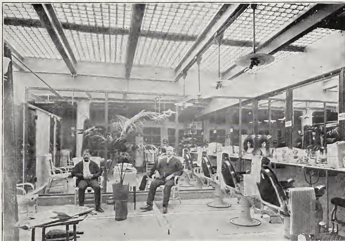
Showing underground Barber Shop of Hotel Wolcott, New York city where no artificial light is ever burned during the day, as same is thoroughly illuminated with natural light through the medium of “Bar-Lock construction and “3-Point” Prisms.
