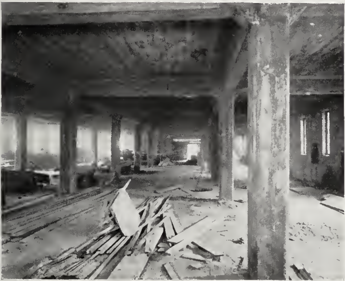
Concrete After Removal of Forms
