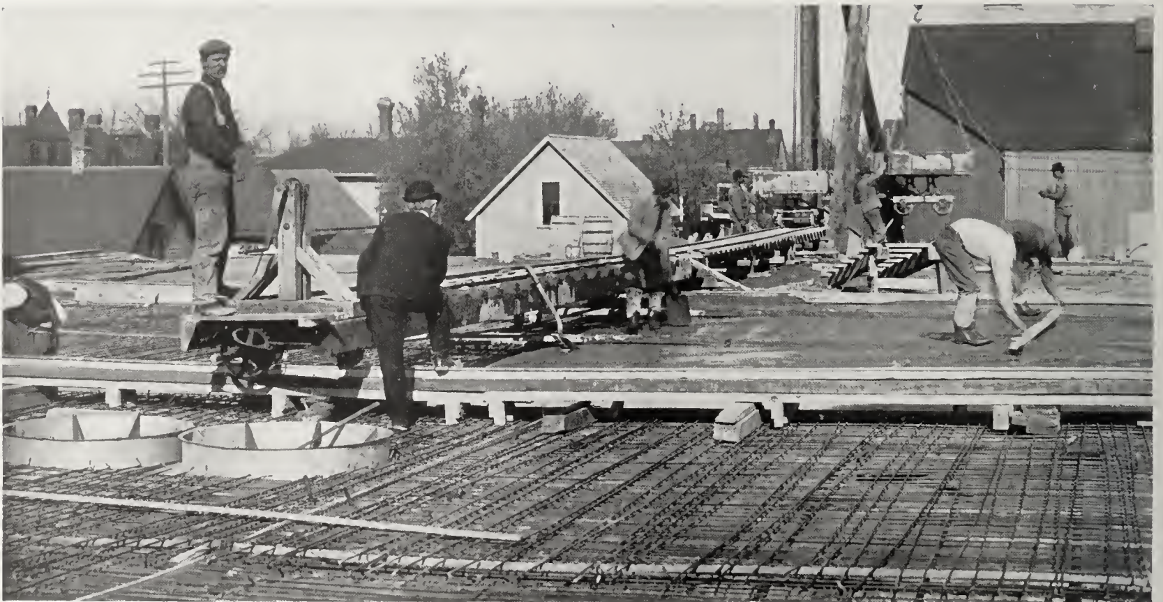
VIEW SHOWING METHOD OF HANDLING CONCRETE
