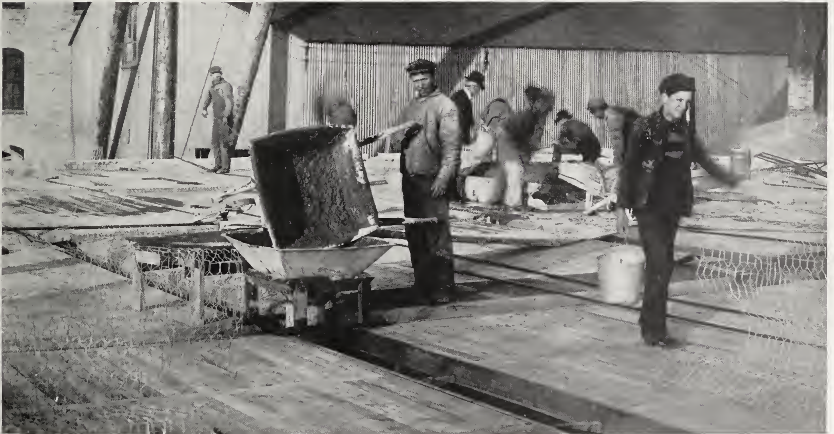
SHOWING FILLING OF COLUMNS
