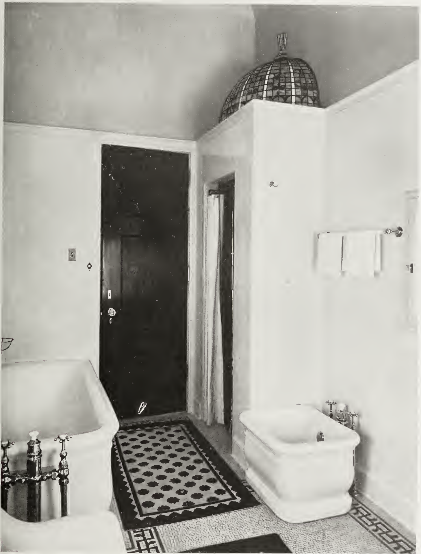
MODERN BATH ROOM—RESIDENCE FREDERICK ROBINSON, ESQ., RACINE, WIS. H. R. Wilson, Architect, Chicago, Ill. Fixtures Supplied by The J. L. Mott Iron Works, New York and Chicago
