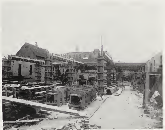
Method of Erection - One Floor in Place
