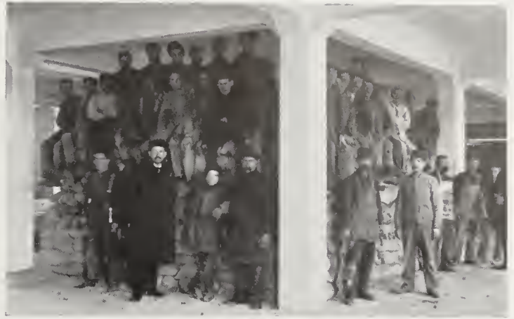
Test 100 Tons on Panel 16-ft. Square - N-W. Knitting Mill Warehouse Plate 4
