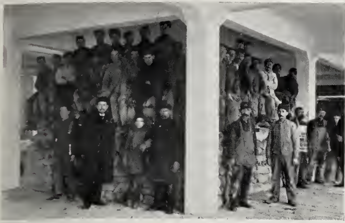
Te is 100 Tons on Panel 16 ft. Square—N.W. Knitting Mill Warehouse, Minneapolis
