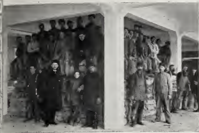
Test 100 Tons on Panel 16-ft. Square—N-W. Knitting Mill Warehouse, Minneapolis
