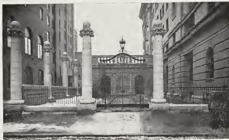
COURT ENTRANCE GATES
