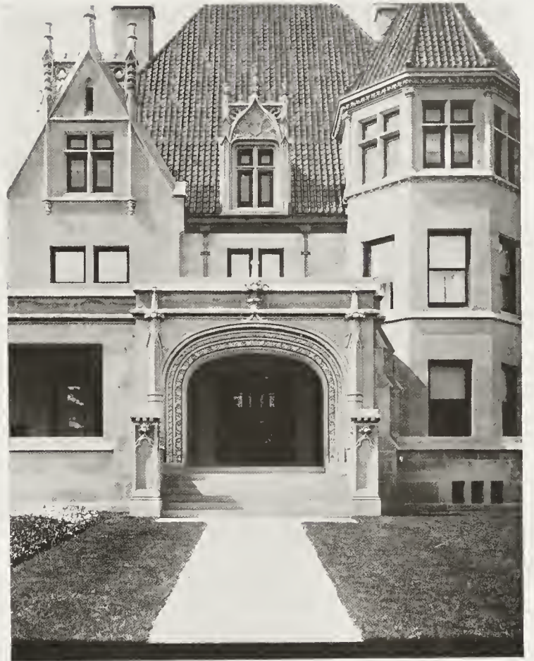
DETAIL OF RESIDENCE FOR J. J. WILLIAMS, SCRANTON, PA. E. H. Davis, Architect
