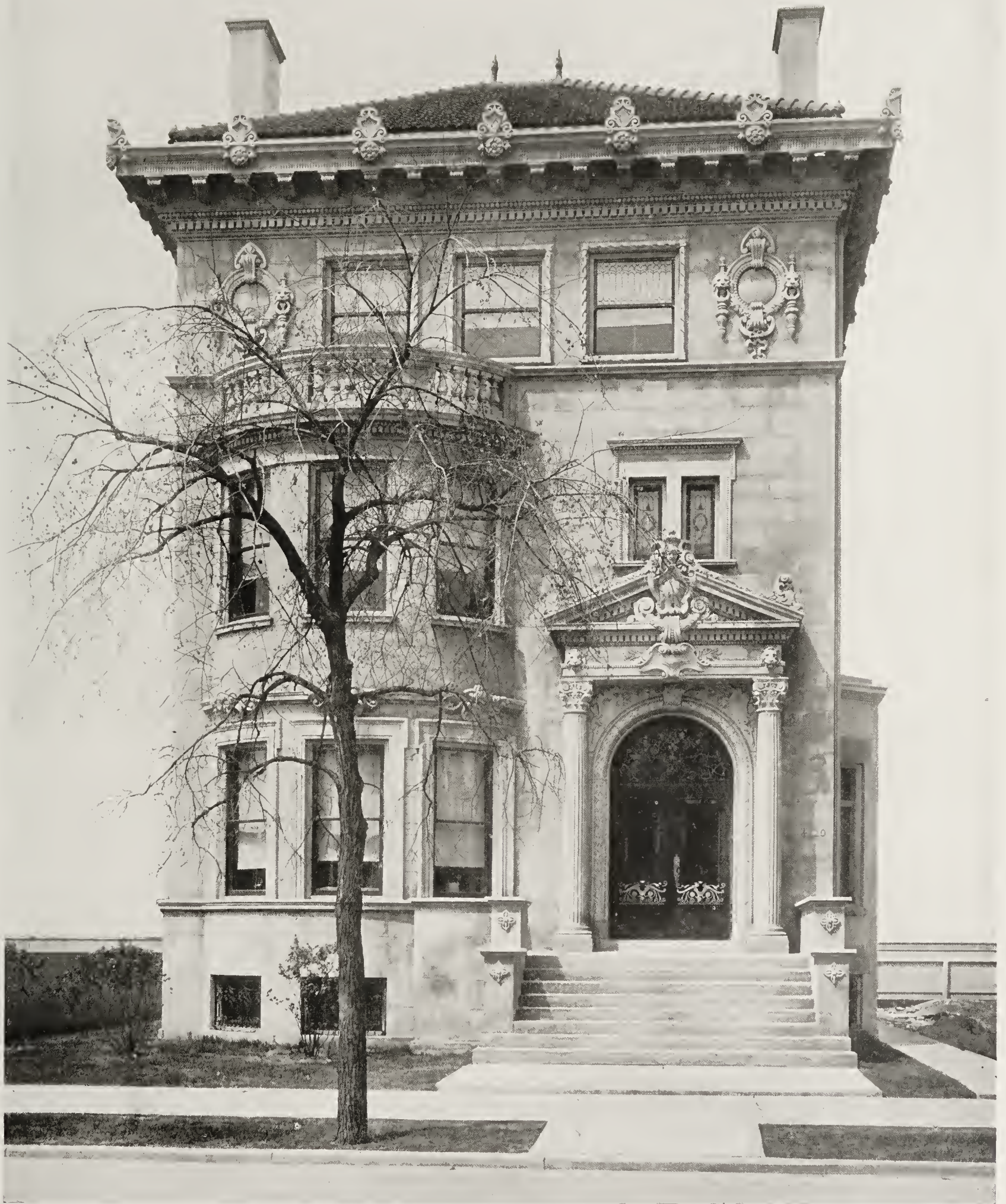
RESIDENCE OF M. LEO HARTMAN, GRAND BOULEVARD, CHICAGO, ILL. Henry L. Ottenheimer, Architect
