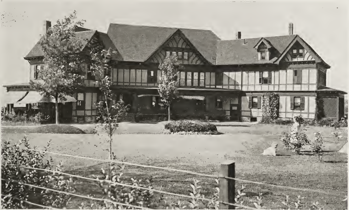
RESIDENCE OF C. D. SIMPSON, DALTON, PA. (Rear View) Herman C. Rutherford, Architect, Scranton, Pa.
