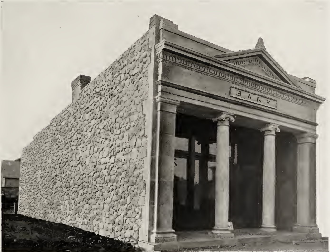
BANK OF WHEATON, WHEATON, MINN. A. F. Gauger, Architect, St. Paul, Minn.
