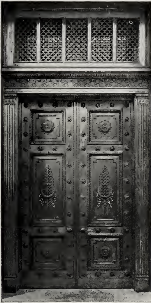
Bronze Doors of Northwestern National Bank, Minneapolis, Minn. Kees & Colburn, Architects
