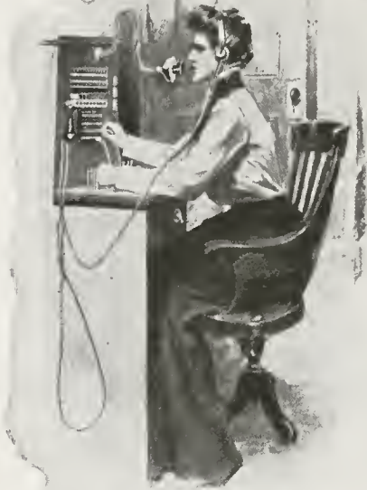
BRANCH EXCHANGE SWITCHBOARD
