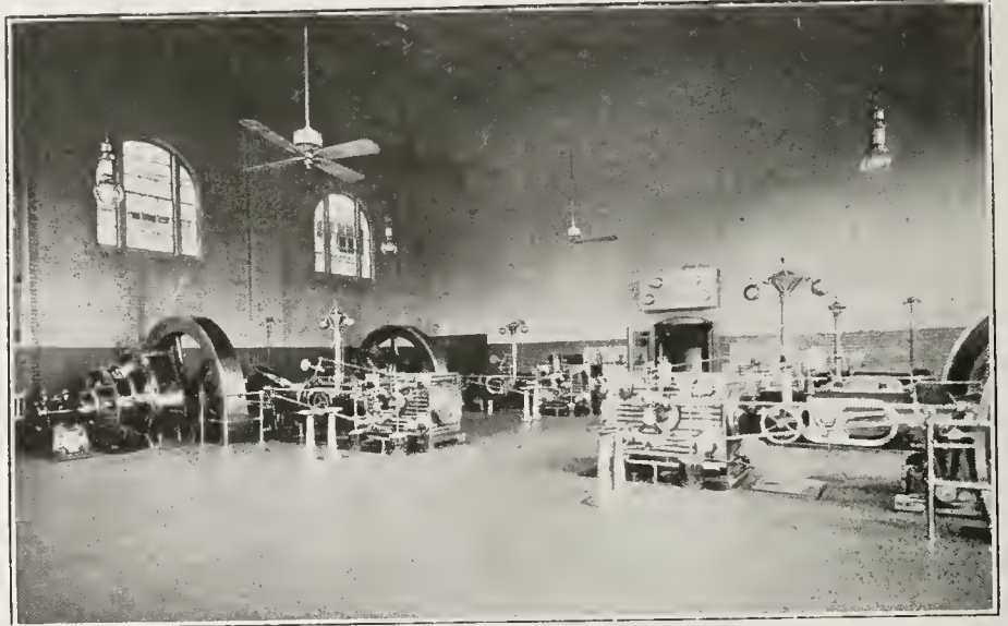
Engine Room of State Capitol.
