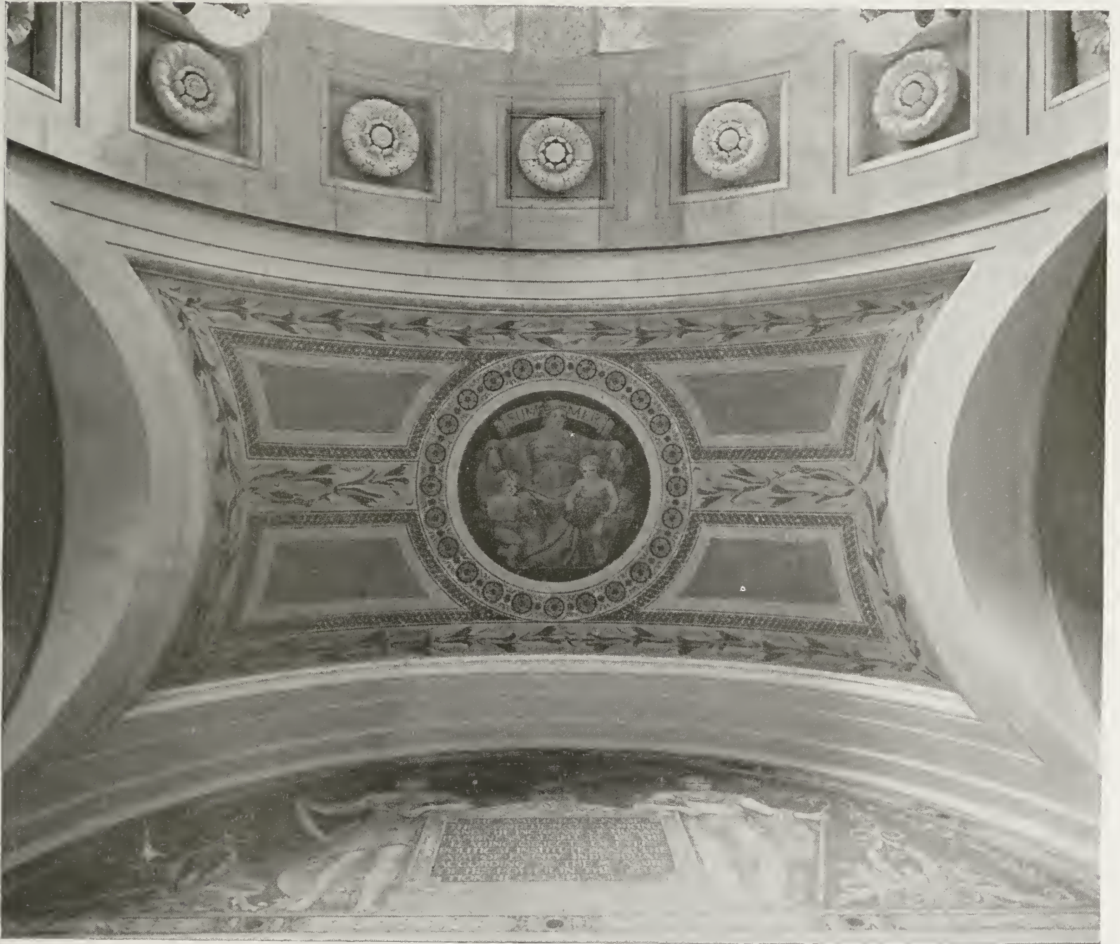
DETAIL OF CEILING DECORATION IN SECOND STORY ROTUNDA CORRIDOR.
