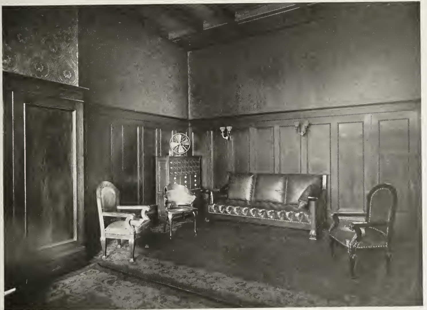
PRIVATE OFFICES PILLSBURY--WASHBURN COMPANY, MINNEAPOLIS, MINNESOTA.
