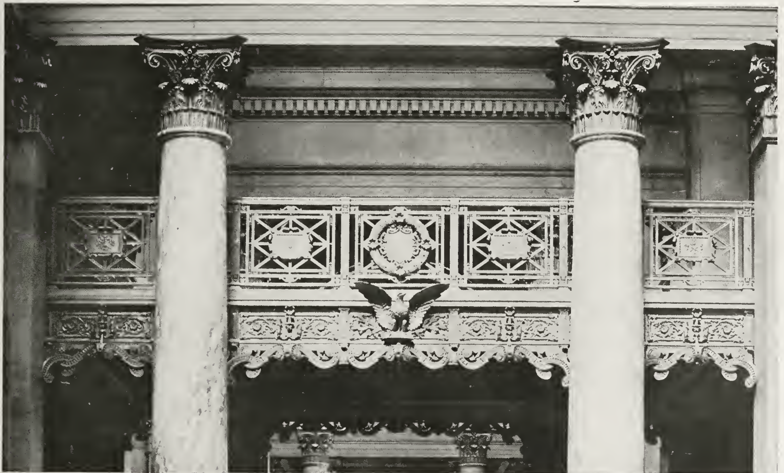
Cast Iron Railing and Facia Third Floor Corridor—Minnesota State Capitol Building
