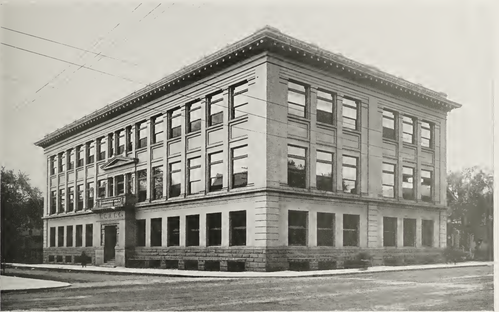
EXTERIOR VIEW OF MINNNEAPOLIS SUB-STATION AND OFFICE BUILDING.
