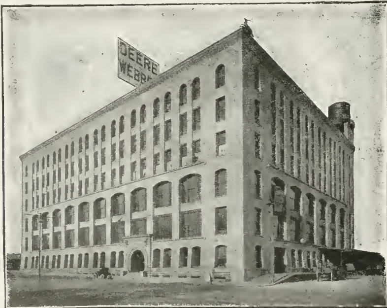
DEERE & WEBBER BUILDING Finest Office and Warehouse in the Northwest 21,300 Square Feet Roofing Used
