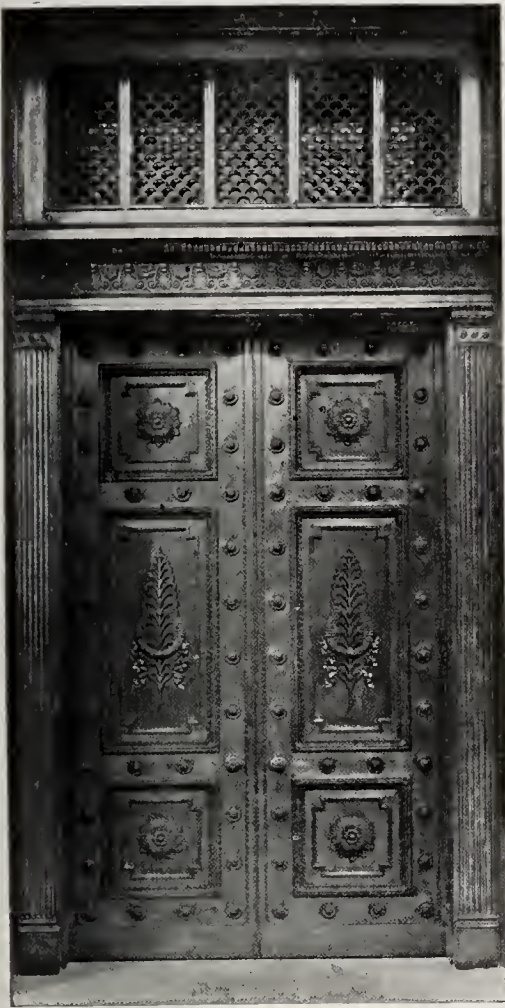
Bronze Doors of Northwestern National Bank, Minneapolis, Minn. Kees & Colbrn, Architects.
