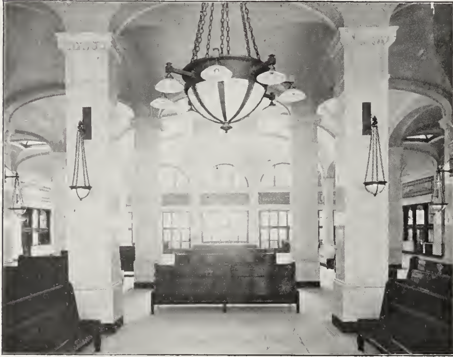
Figure 5—La Salle Station, Chicago—Waiting Room
