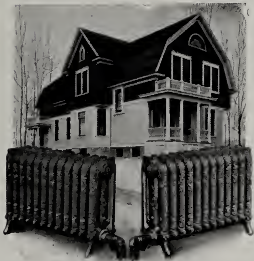
Fenced in against discomfort on all sides of the building.
