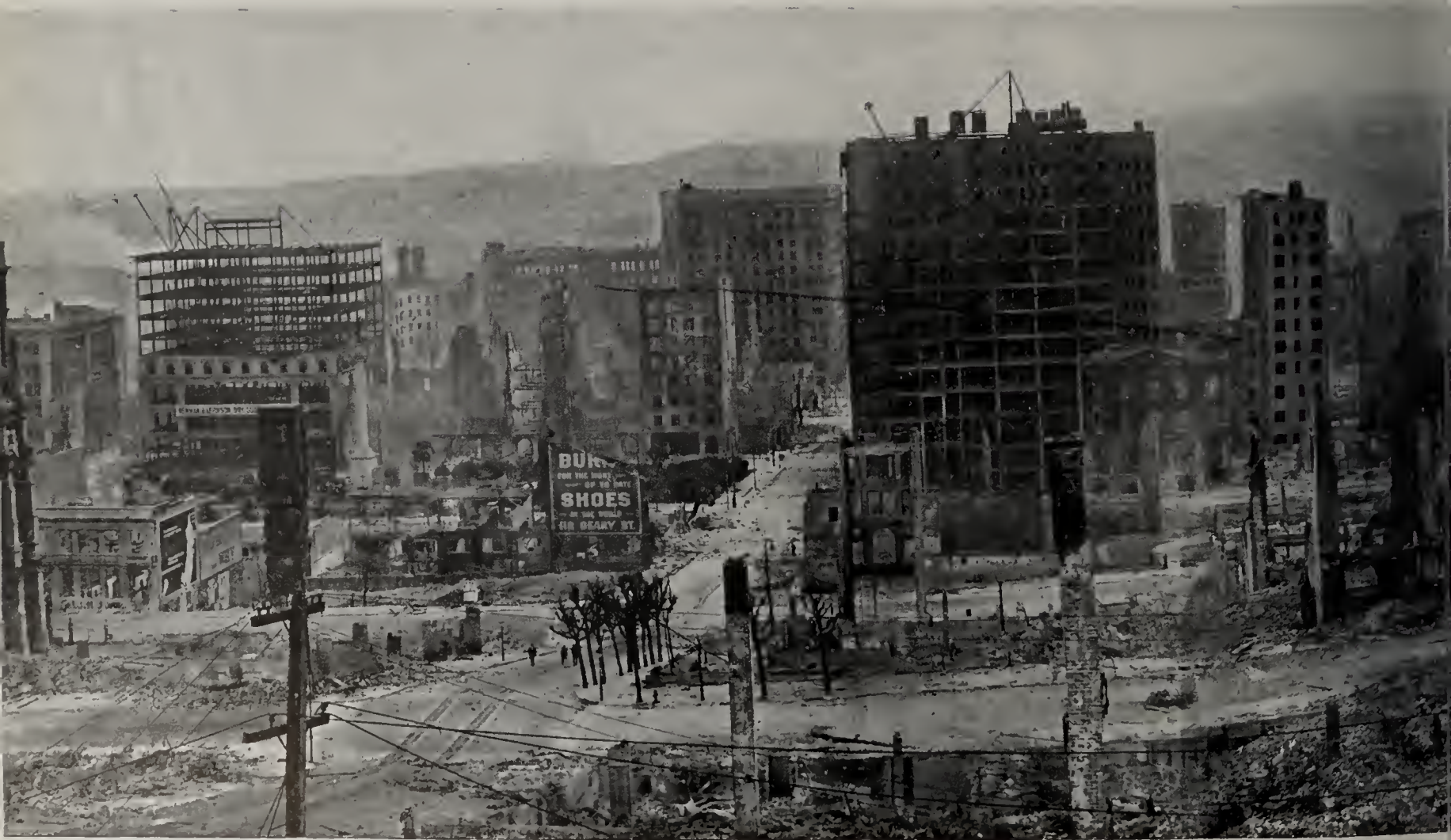
TAKEN DIRECTLY AFTER THE EARTHQUAKE AND FIRE OF APRIL 18, 1906.
