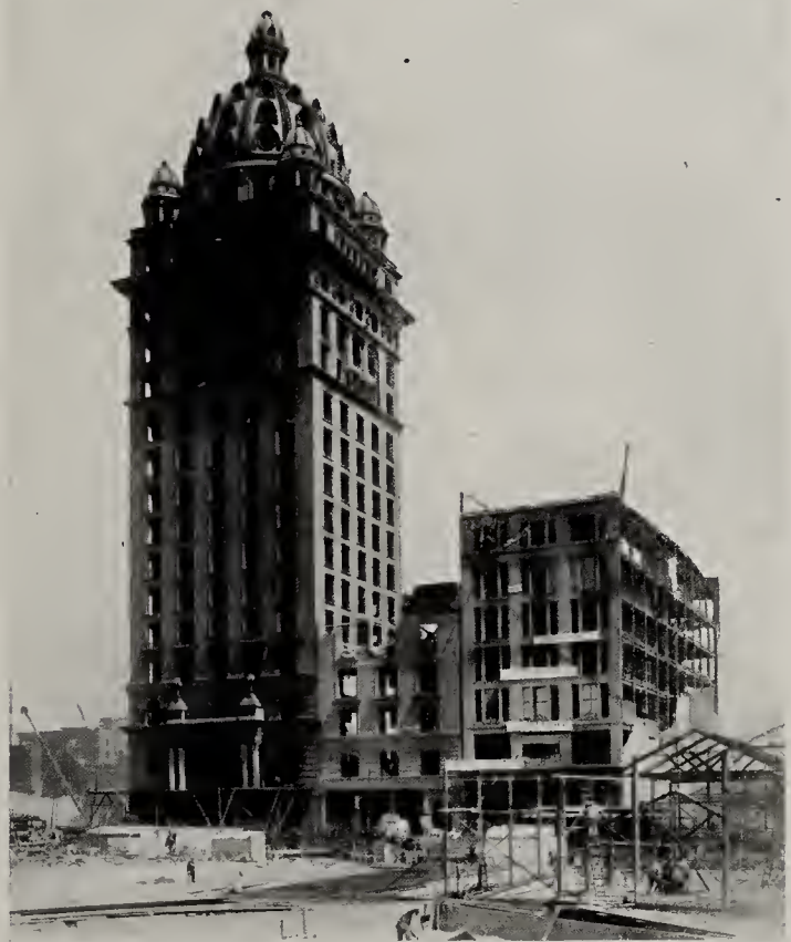
The only thing that went through the experience more or less intact was the steel building
