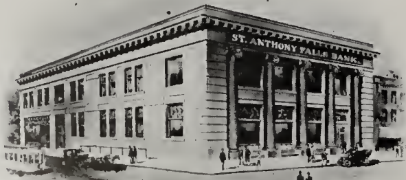
St. Anthony Falls Bank, Minneapolis, Heated by Andrews Locomotive Steel Boiler and The Andrews System.
