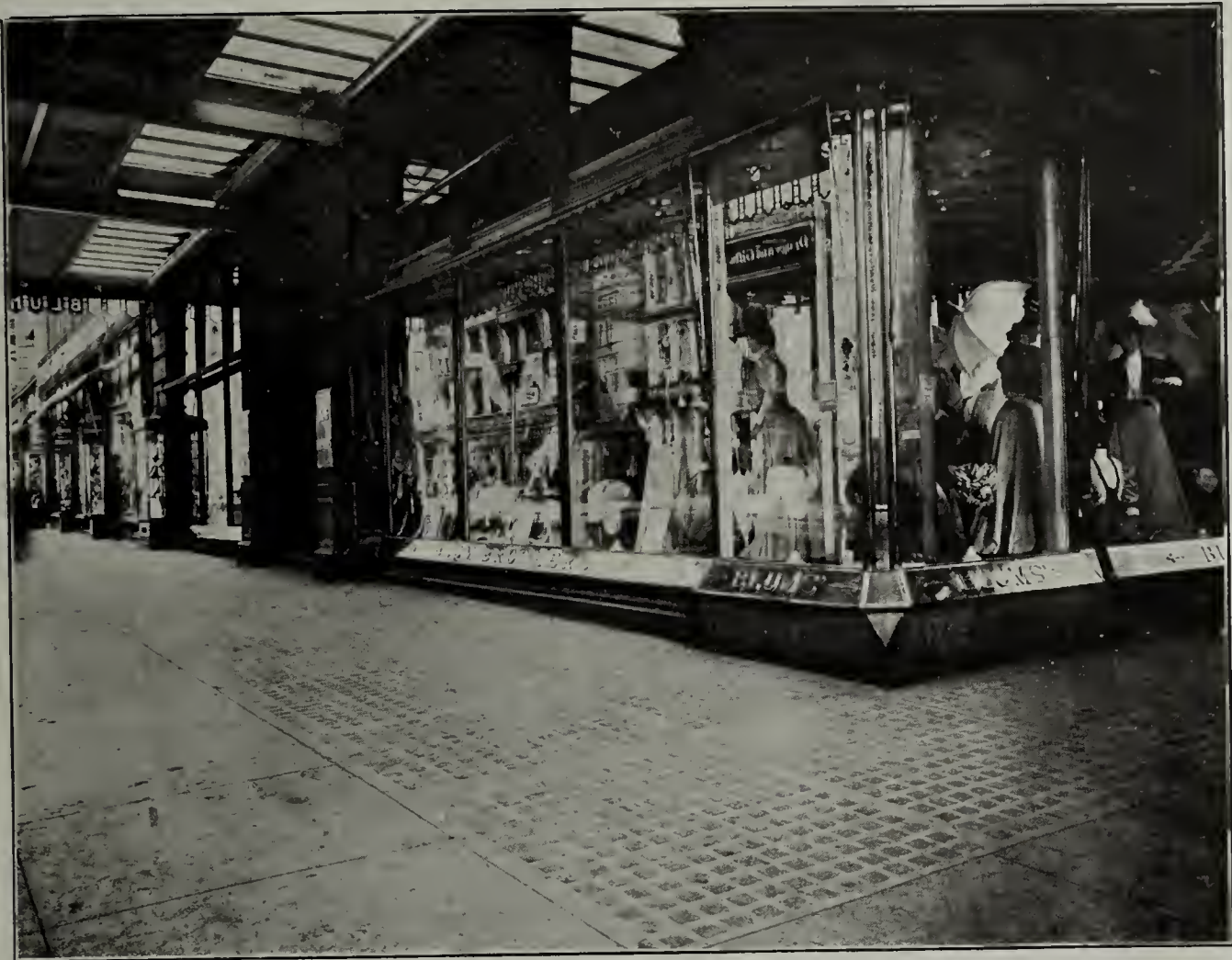
BLUM BROTHERS' DEPARTMENT STORE, PHILADELPHIA, PA. 'Bar-Lock' Galvanized Wrought Steel Construction and Patented "3" Point Prisms were used, which effectually lights the basement.
