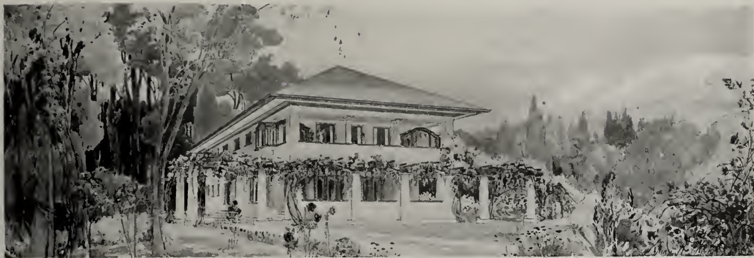
RESIDENCE OF E. B. BLIND, PASADENA, CALIFORNIA
