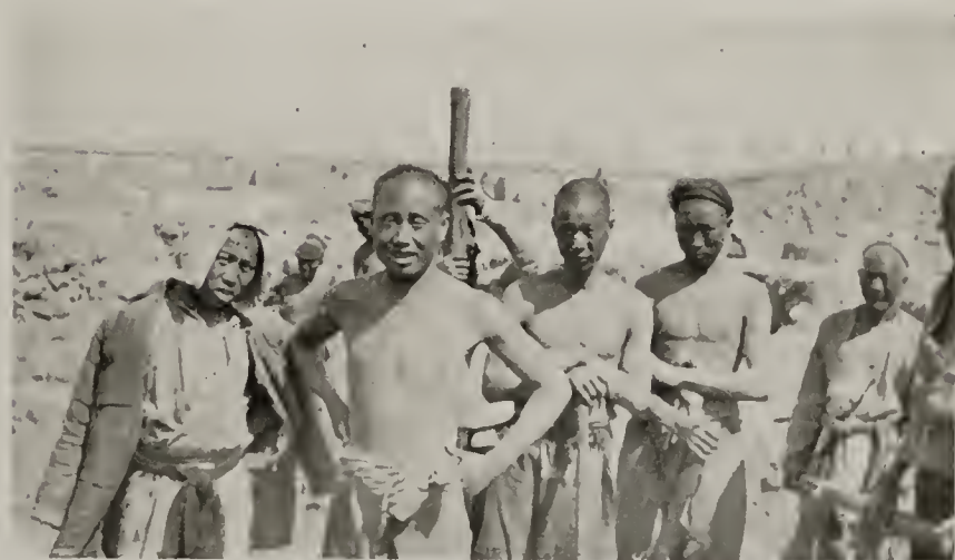
COOLIES ENGAGED IN EXCAVATION
