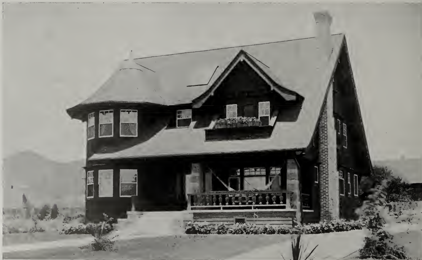
RESIDENCE (A) FOR O. P. DENNIS LOS ANGELES CAL DENNIS & FARWELL ARCHITECTS
