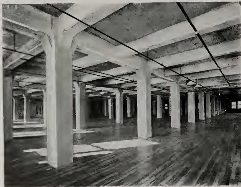
FINISHED SECTION OF 5TH FLOOR
