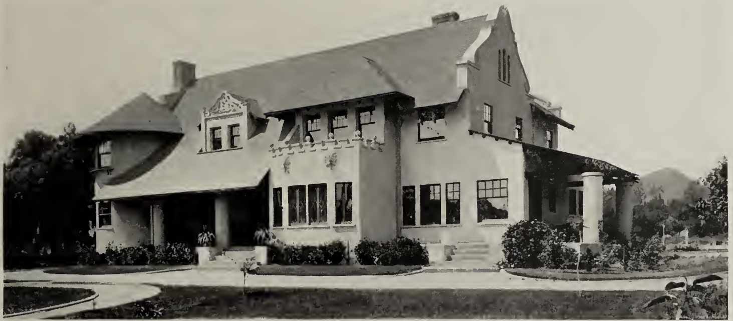
RESIDENCE OF H. C. BEVILLE, HOLLYWOOD, CALIFORNIA. HUNT AND EAGER, ARCHITECTS, LOS ANGELES.
