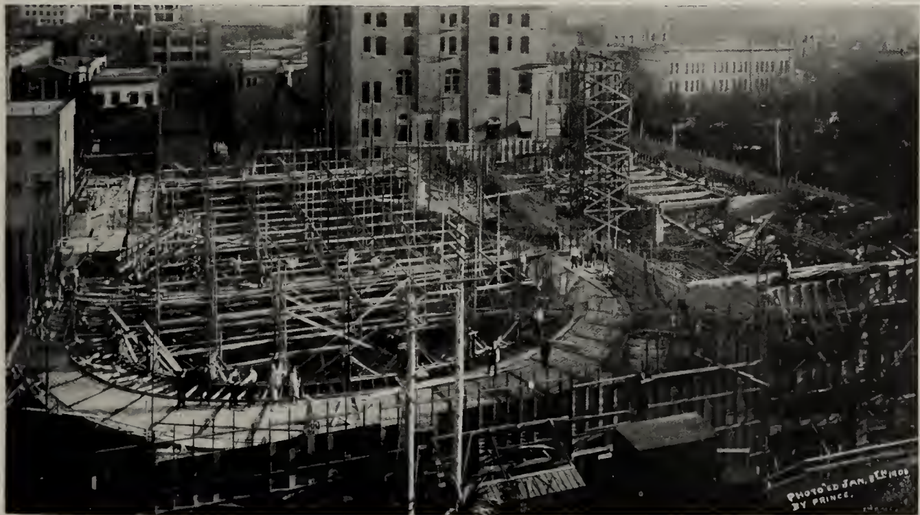
VIEW OF CONSTRUCTION OF AUDITORIUM.
