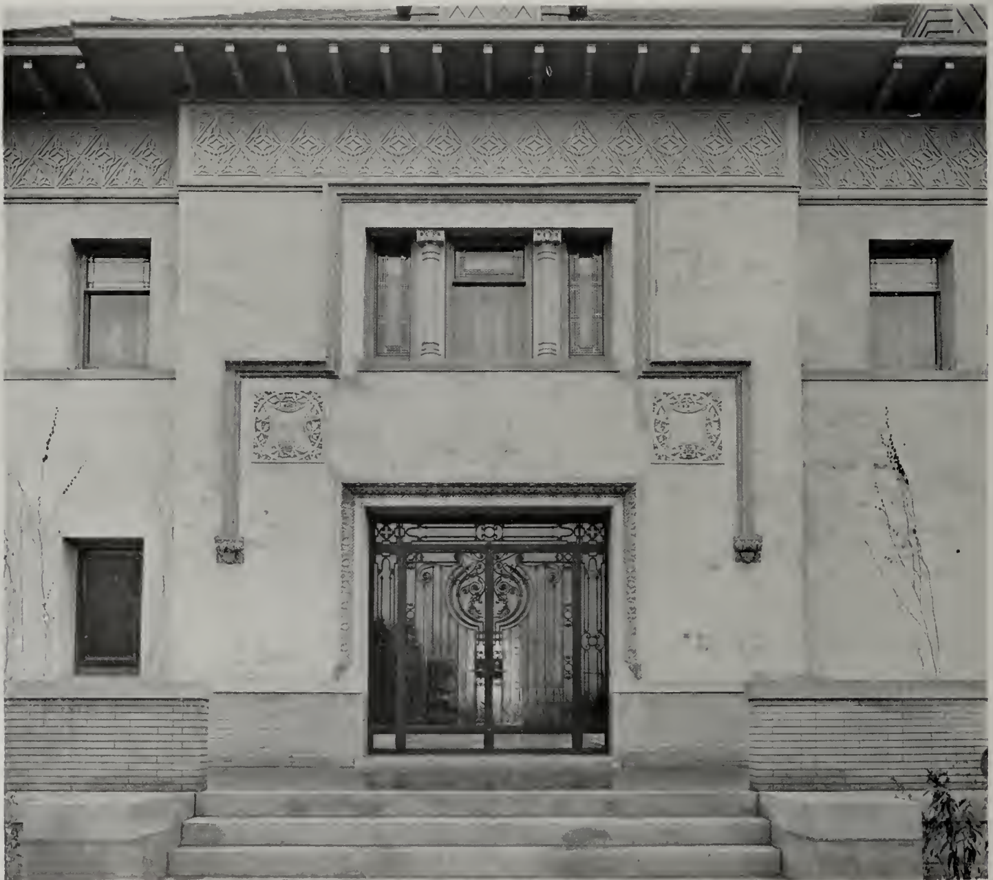
ENTRANCE DETAIL OF RESIDENCE FOR MR. P. R. BROOKS, MINNEAPOLIS MINN.
