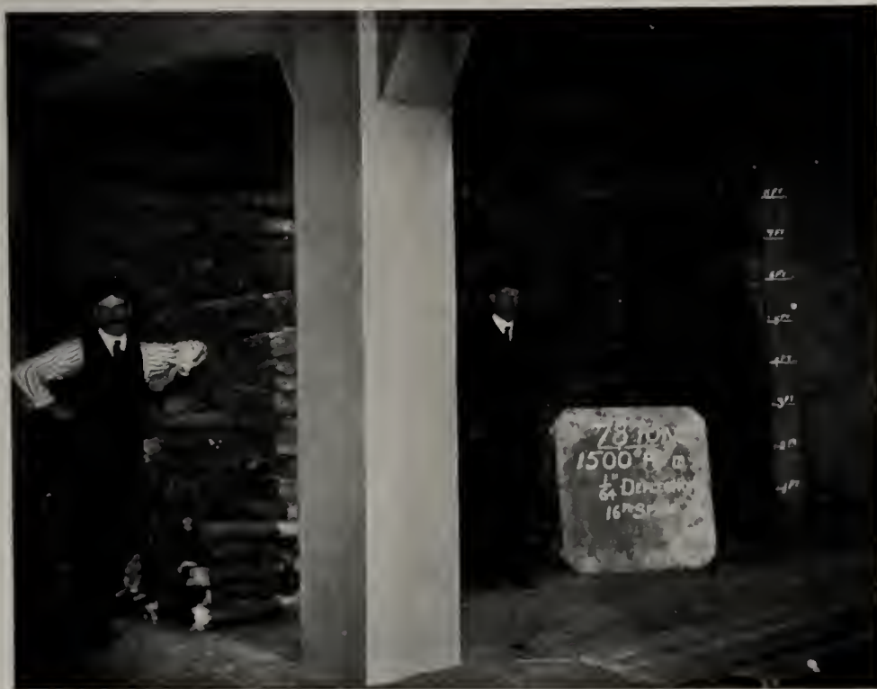
TEST MADE 2ND FLOOR
