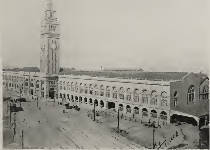
THE FERRY HOUSE, UNINJURED EXCEPT SLIGHT CRACKS IN TOWER
