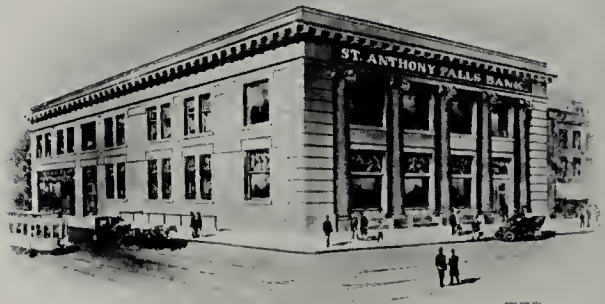
St. Anthony Falls Bank, Minneapolis, Heated by Andrews Locomotive Steel Boiler and The Andrews System.
