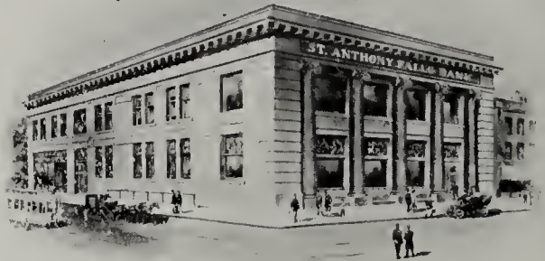
St. Anthony Falls Bank, Minneapolis, Heated by Andrews Locomotive Steel Boiler and The Andrews System.
