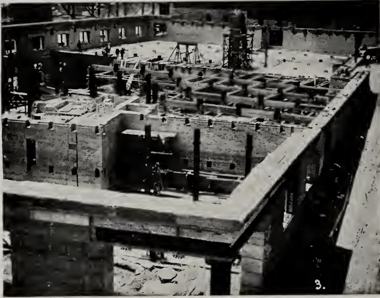
SHOWING WEST SECTION OF 3RD FLOOR COMPLETE
