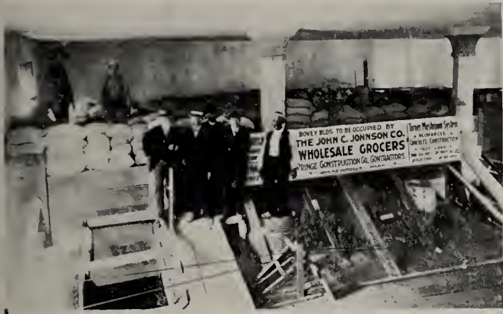
Test load of 180 tons to the square foot, applied to Mushroom System. Deflection scant \frac{1}{4} of an inch.
