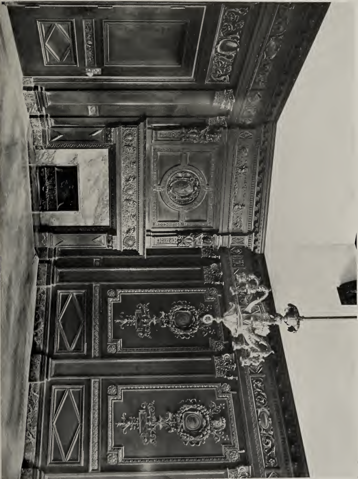
POSTMASTER'S PRIVATE OFFICE, U. S. POST OFFICE, SAN FRANCISCO, CALIFORNIA JAMES KNOX TAYLOR, SUPERVISING ARCHITECT, WASHINGTON, D. C.
