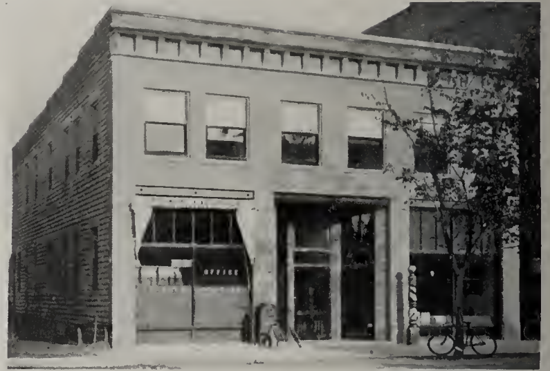
LYNDALE BRANCH OF MINNEAPOLIS POST OFFICE Front, Cement Brick and Stone. Cornice, Artificial Stone, manufactured and built by the Anchor Stone Laundry Tray Company, Minneapolis
