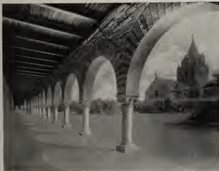
GOthic CHAPEL AT STANFORD UNIVERSITY, COMPLETELY DESTROYED
