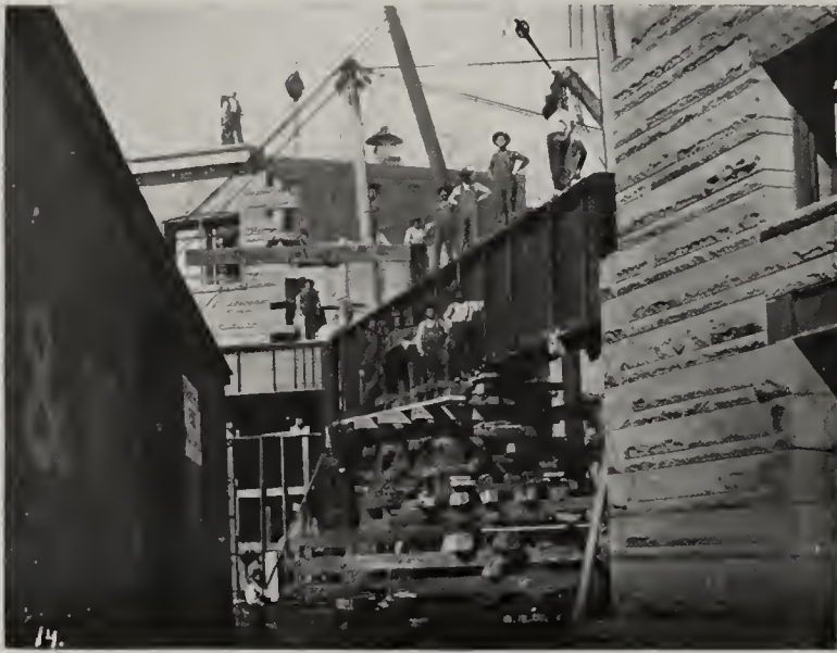
PUTTING IN PLACE 38 TON GIRDER
