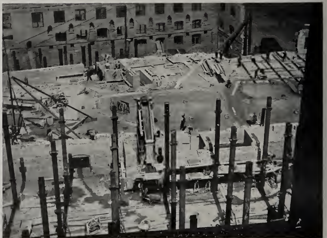
3RD FLOOR, TAKEN FROM ARMY BUILDING
