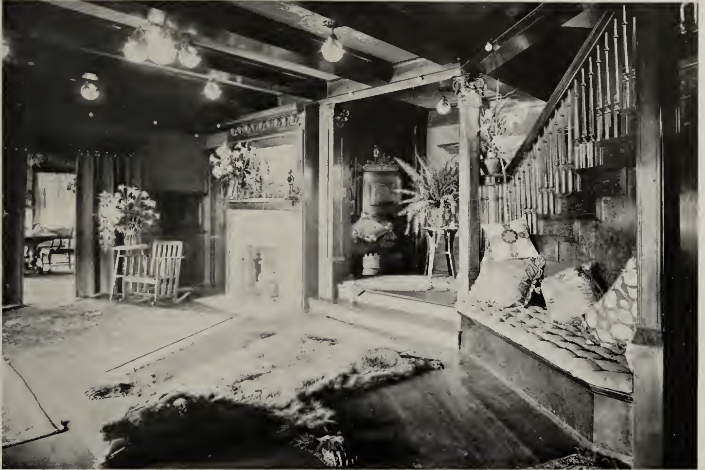
HALL IN RESIDENCE OF FRANK WILSON, ESQ., LOS ANGELES, CALIFORNIA. HUNT AND EAGER, ARCHITECTS.
