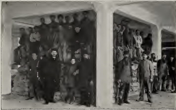
Test 100 Tons on Panel 16-ft. Square—N.W. Knitting Mill Warehouse, Minneapolis
