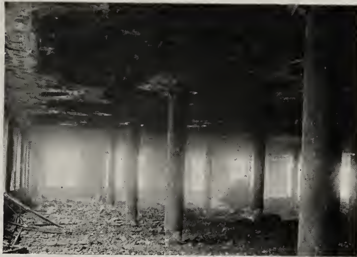
Note excellent condition of hollow tile floor arches and column covering.
