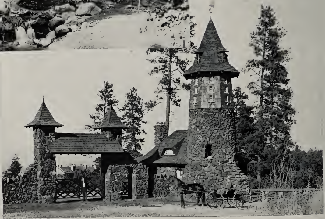
LODGE AND WATER TOWER IN GROUNDS OF L. M. DAVENPORT, SPOKANE, WASHINGTON Cutter and Malmgren, Architects
