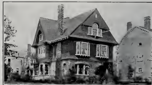
Residence at Newark, N. J. (Sheathed with Neponset) John H. & Wilson C. Ely, Architects.
