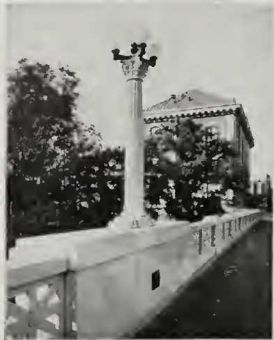
Railing of Bridge at Fergus Falls, Minn.
