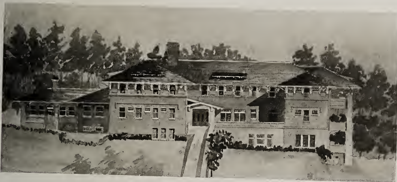
CHILDREN'S HOME, SPOKANE, UNDER CONSTRUCTION R. C. SWEATT, ARCHITECT
