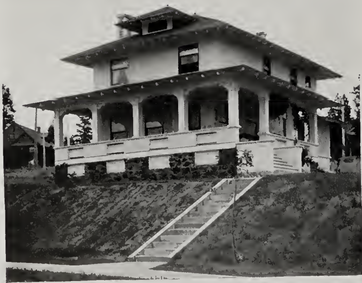
RESIDENCE OF HARL J. COOK, SPOKANE Clapp and Clapp, Architects
