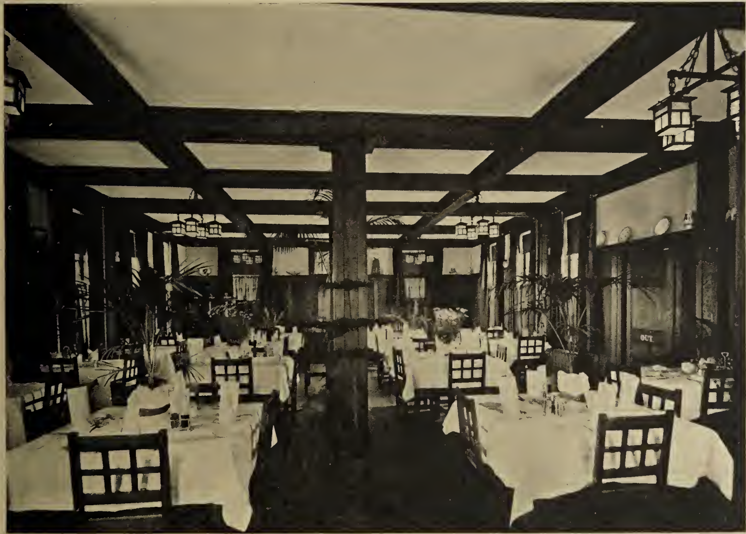
DINING ROOM IN DEER LODGE, WINNIPEG, MANITOBA PRATT AND RASS, ARCHITECTS
