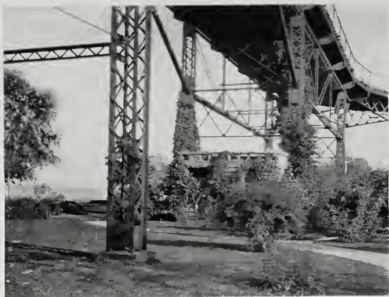
PUBLIC COMFORT STATION, WINONA RIVER FRONT EXAMPLE OF HOW VIACUCT PIERS CAN BE DECORATED AND SPACE UTILIZED
