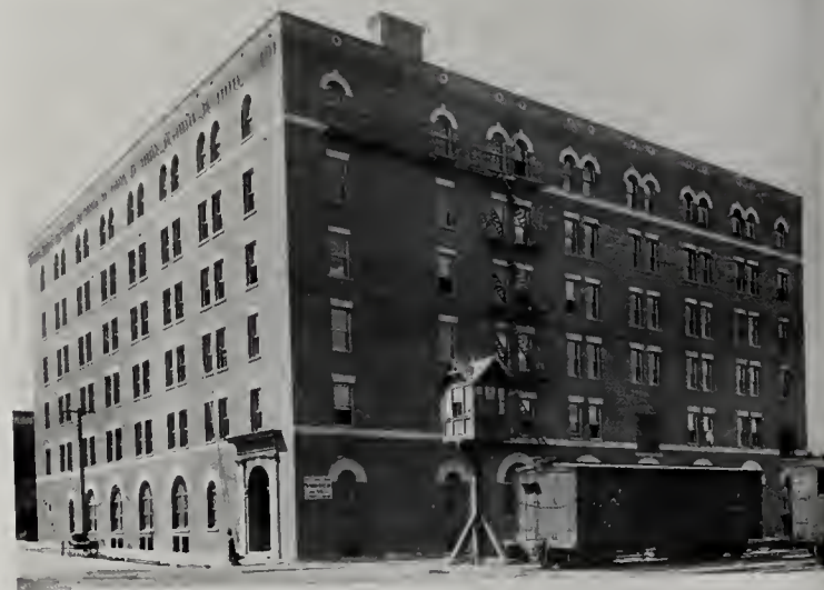
SPOKANE DRY GOODS COMPANY WAREHOUSE L. L. Rand, Architect
