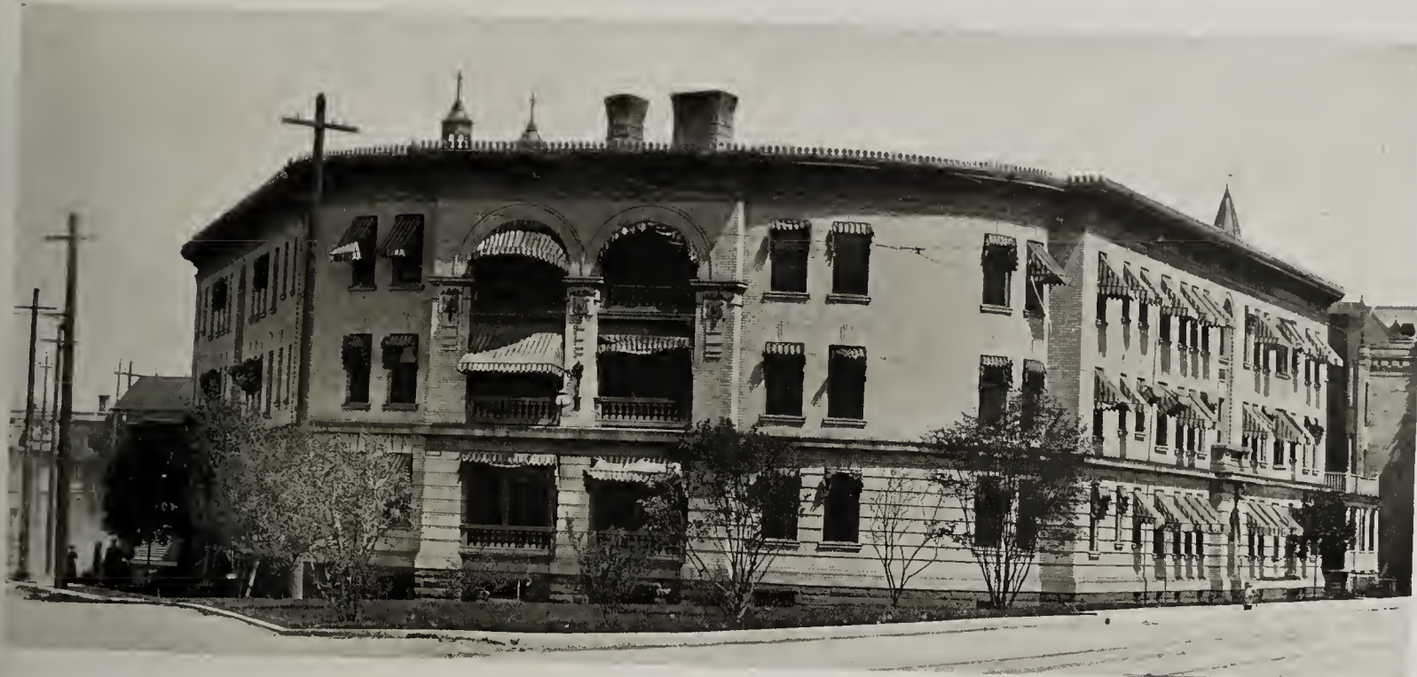
SAN MARCO APARTMENTS, SPOKANE, WASHINGTON ALBERT HELD, ARCHITECT
