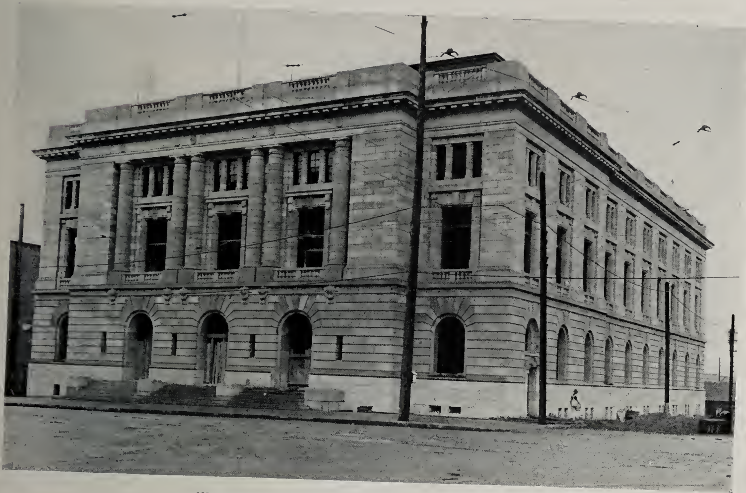
NEW POST OFFICE BUILDING, SPOKANE, WASHINGTON J. KNOX TAYLOR, ARCHITECT
