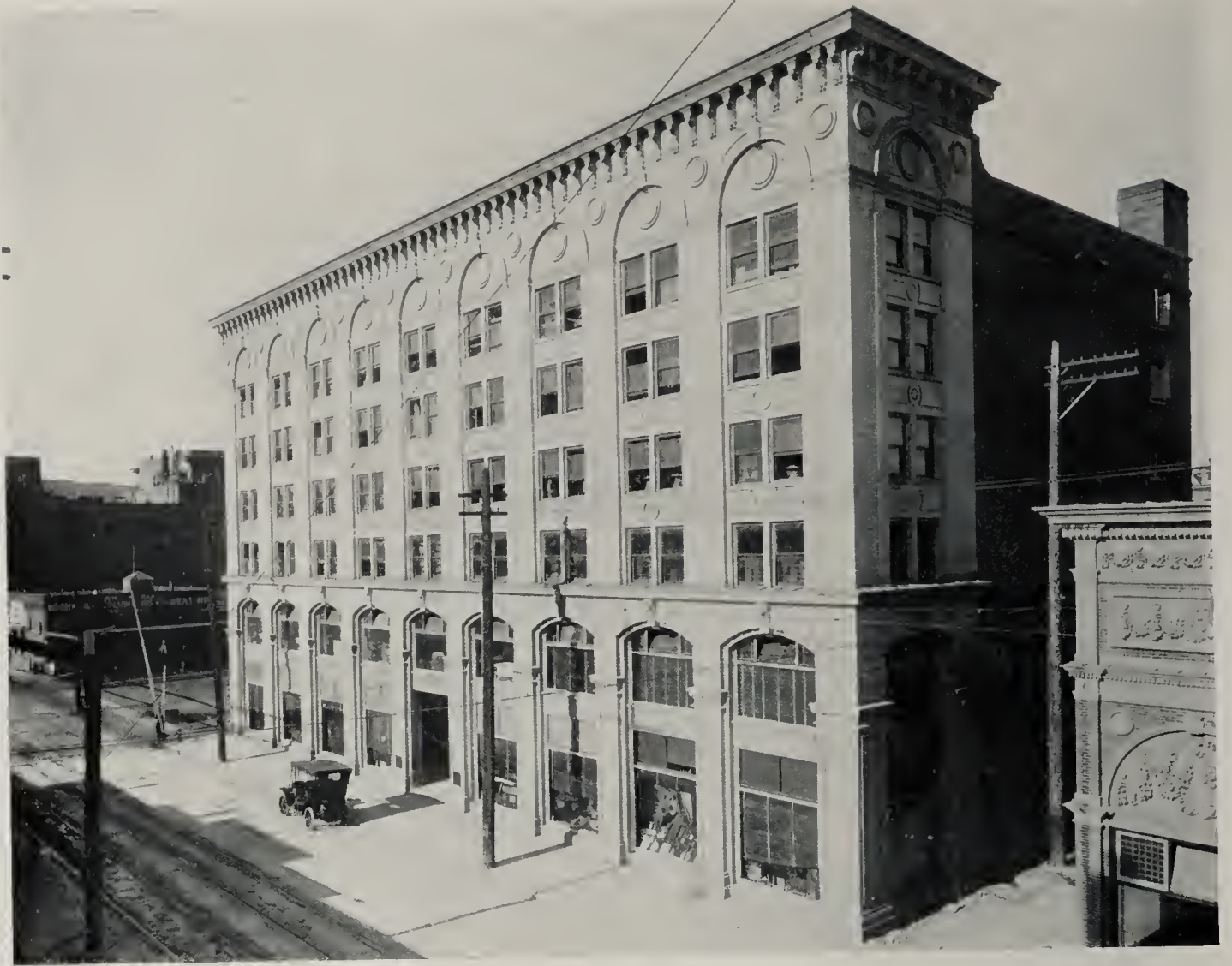
HOLLEY MASON & COMPANY'S BUILDING, SPOKANE ALBERT HELD, ARCHITECT
