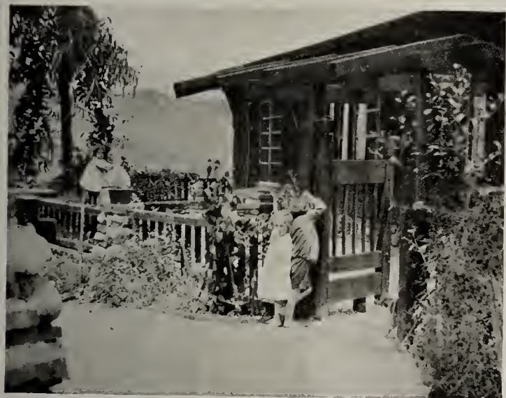
WEST VIEW OF PART OF BUNGALOW NUMBER 1
