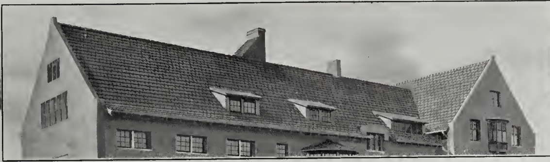
Asbestos "Century" Shingle Roof—Private Stable, Pabst Farms, Oconomowoc, Wis. Fernekes & Cramer, Milwaukee, Architects; Consolidated Sheet Metal Works, Milwaukee, Roofing Contractors
