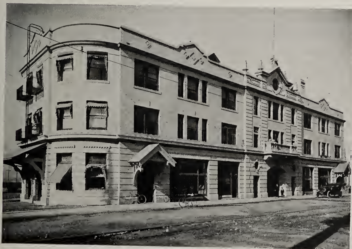
TERMINAL STATION, SPOKANE, WASHINGTON ALBERT HELD, ARCHITECT
