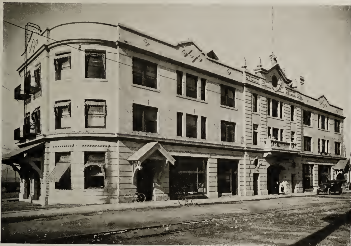
TERMINAL STATION, SPOKANE, WASHINGTON ALBERT HELD, ARCHITECT
