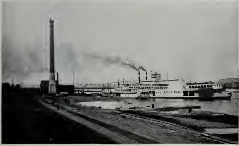
WINONA LEVEE IN 1893. A TYPICAL RIVER LEVEE WITHOUT IMPROVEMENTS
