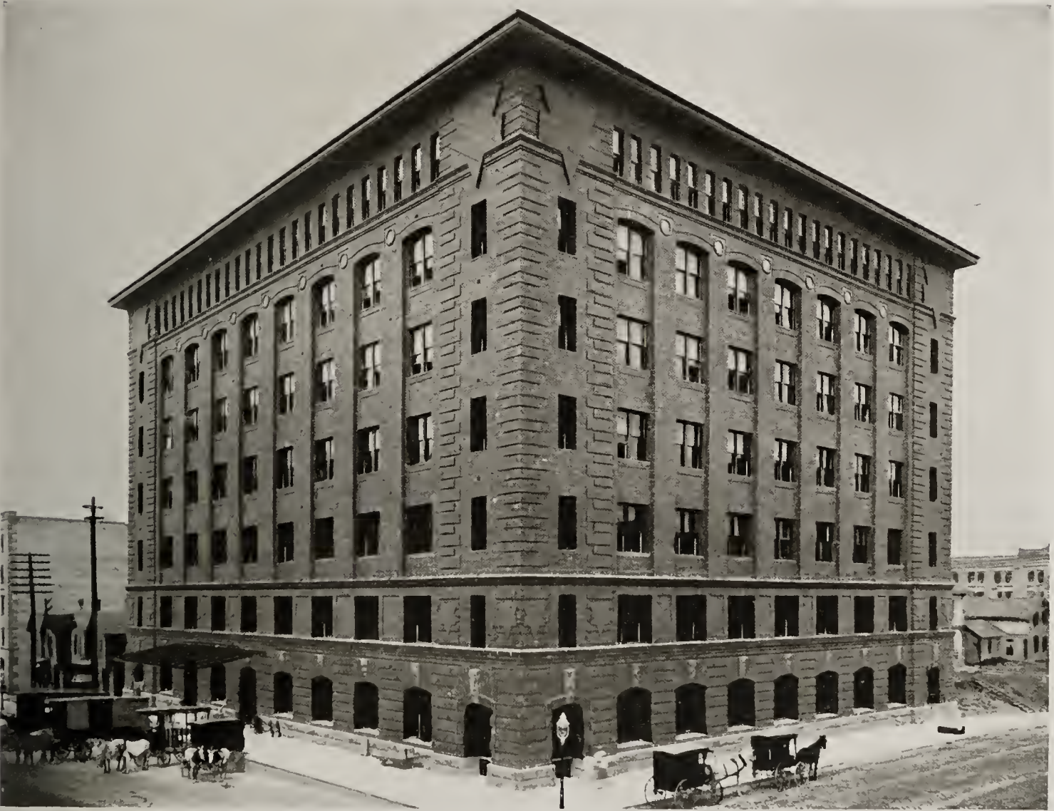
HURTY-SIMMONS BUILDING, MINNEAPOLIS, MINNESOTA GORDON, TRACY AND SWARTWOUT, ARCHITECTS, NEW YORK
