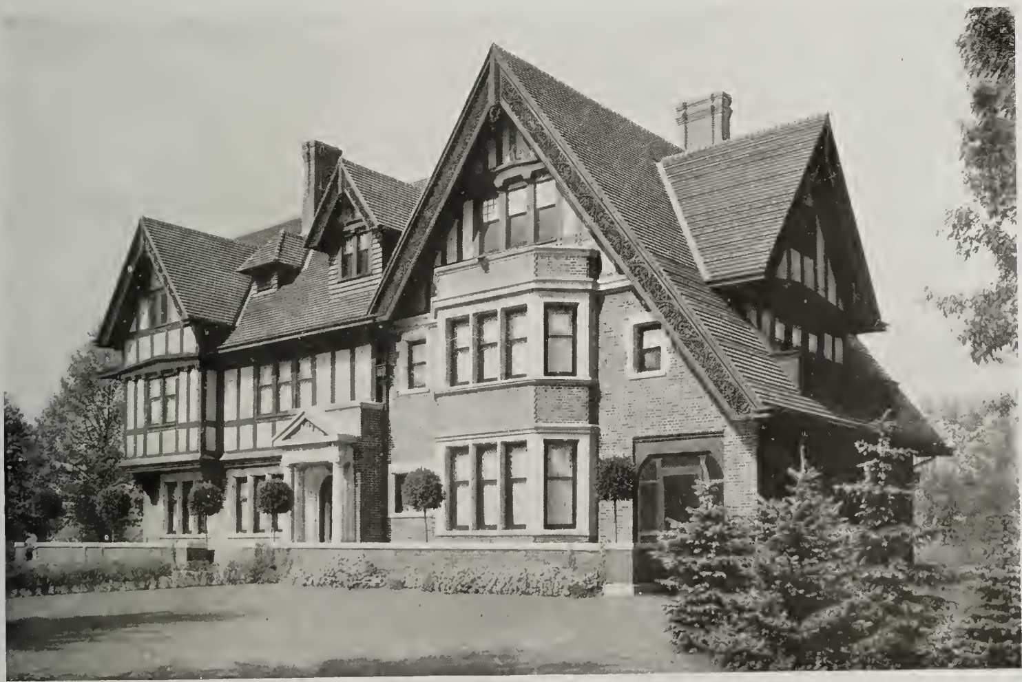
RESIDENCE OF S. W. DITTENHOFER, ST. PAUL, MINNESOTA CLARENCE H. JOHNSTON, ARCHITECT
