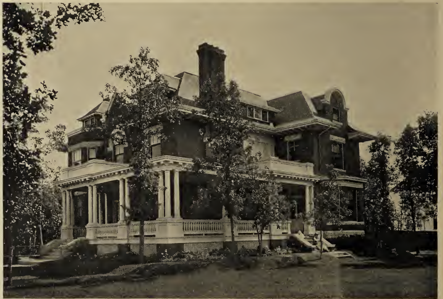
RESIDENCE OF H. H. BRADBURN, WINNIPEG, MANITOBA J. H. G. RUSSELL, ARCHITECT
