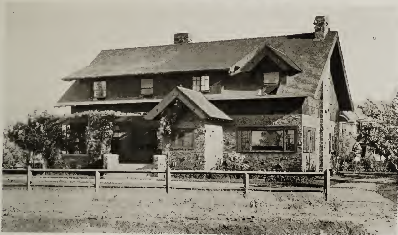
RESIDENCE OF WALDO PAINE SPOKANE, WASHINGTON C. FERRIS WHITE ARCHITECT DENNISON PHOTO
