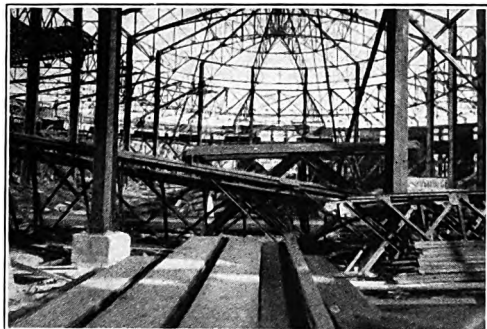
STOCK PAVILION, DENVER. 900,000 lbs. Structural Steel
