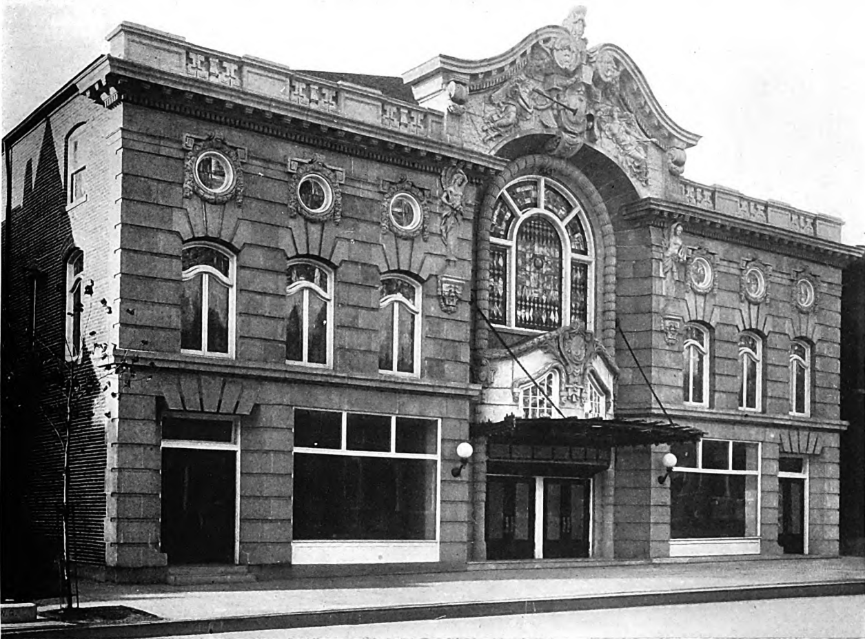
Photograph by Courtesy of Sandusky Portland Cement Co.
