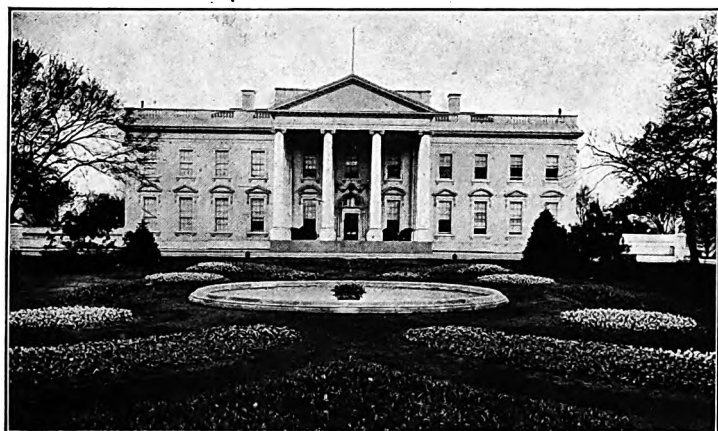
NEPONSET BUILDING PAPERS IN WHITE HOUSE, WASHINGTON, D. C.
