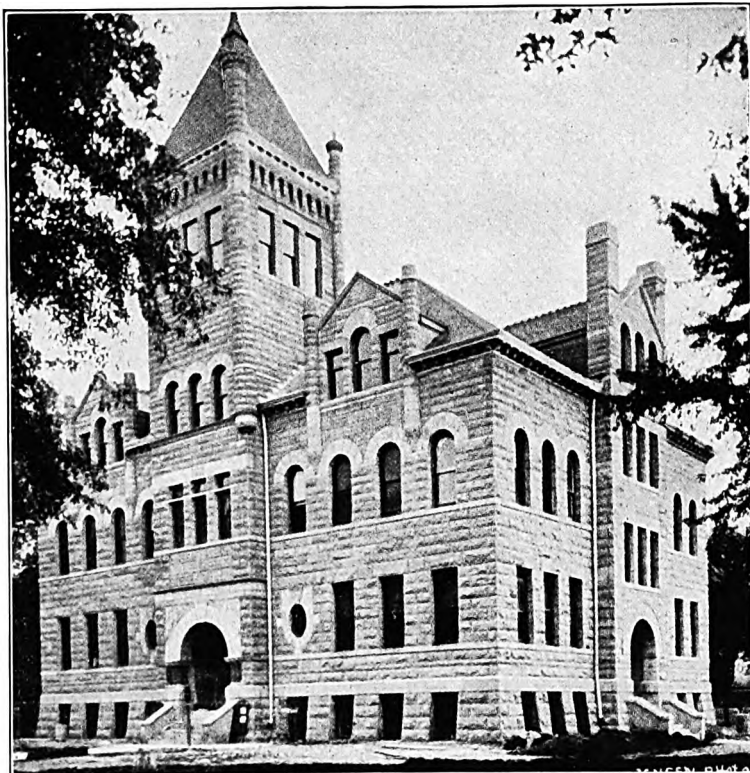
UNION COUNTY COURT HOUSE, ELK POINT, SO. DAKOTA Built of Kettle River Sandstone
