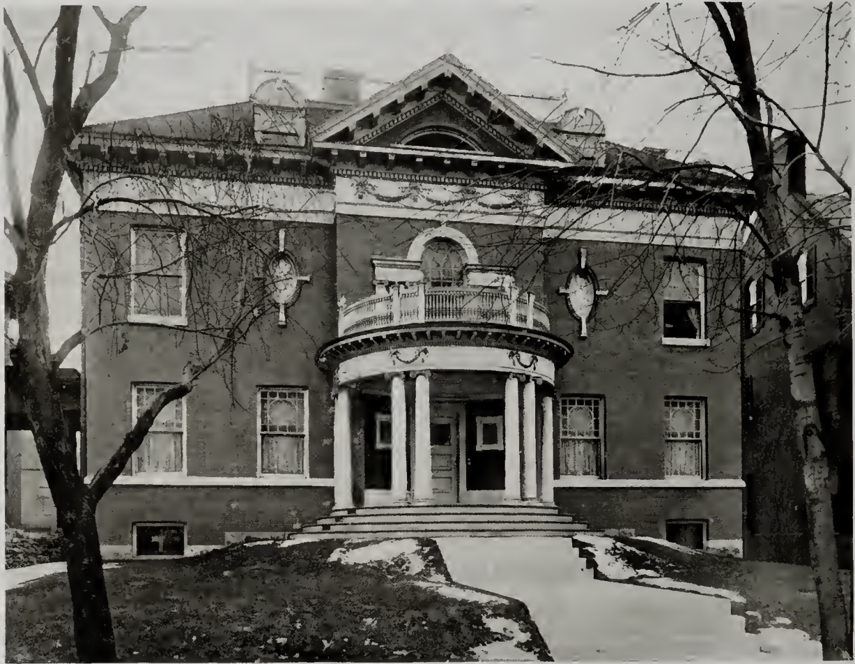
RESIDENCE F. D. HIRSCHBERG, ST. LOUIS BARNETT, HAYNES & BARNETT, ARCHITECTS
