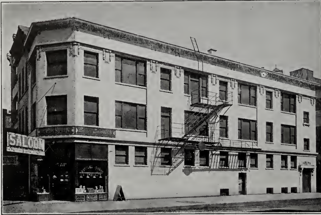
Store and Apartment Building, Madison and Jefferson Sts., Chicago, Ill.
