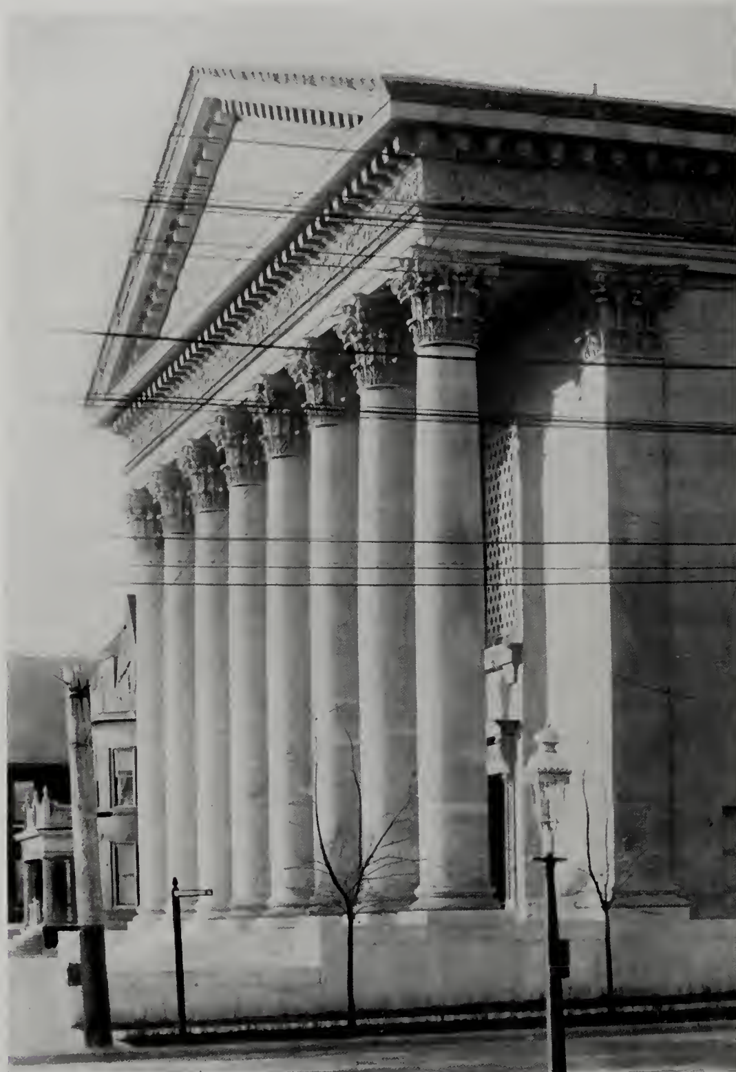
TEMPLE ISRAEL, ST. LOUIS, MISSOURI. BARNETT, HAYNES & BARNETT, ARCHITECTS. HYDRAULIC PRESSED BRICK
