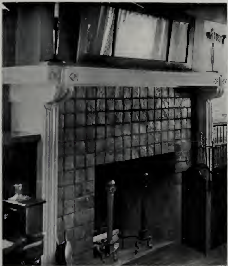
FIREPLACE OF UNUSUALLY GOOD PROPORTIONS. THE TILES ARE PLANNED TO HARMONIZE WITH GENERAL COLOR SCHEME OF ROOM. EACH TILE VARIES IN COLOR AND YET CONTRIBUTES TO ITS NEIGHBOR. NOT THE LEAST INTERESTING, IS THE SETTING IN CEMENT
