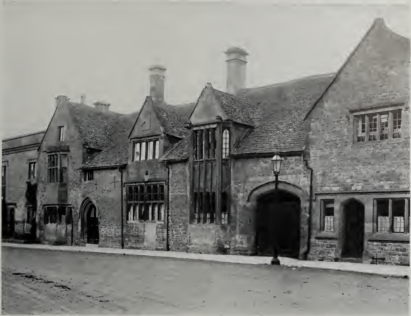
GREVEL HOUSE, CAMPDEN. BUILT BY WILLIAM GREVEL THE WOOLSTAPLER, IN 1396
