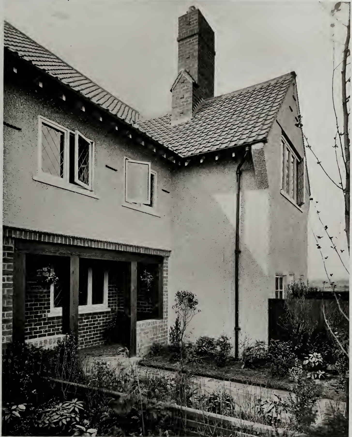
GARDEN FRONT RESIDENCE, WALSEND-ON-TYNE, ENGLAND EDWARD CRATNEY, ARCHITECT
