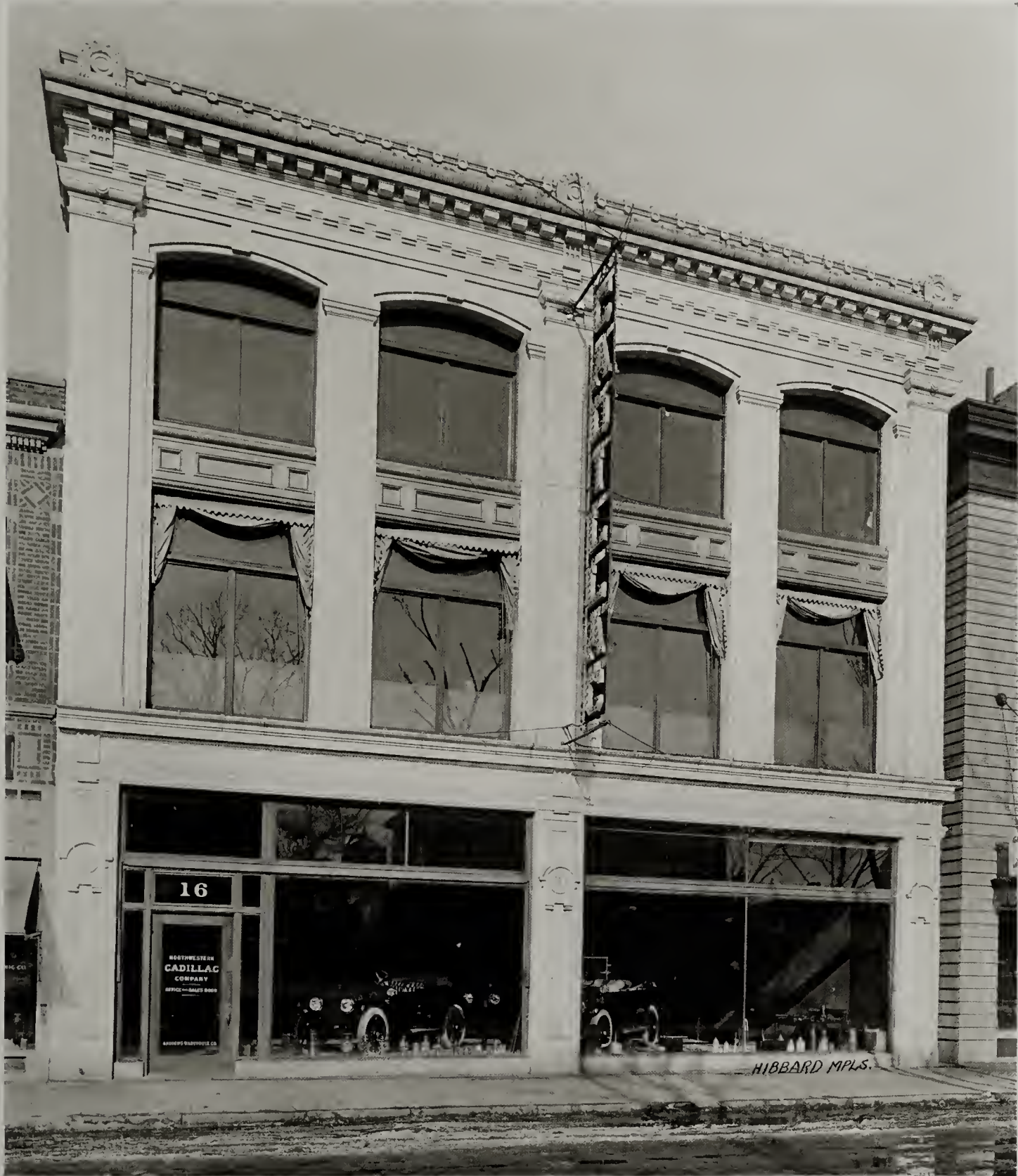
THREE STORY COMMERCIAL BUILDING, MINNEAPOLIS, MINNESOTA VICTOR F. V. DE BRAUWERE, ARCHITECT
