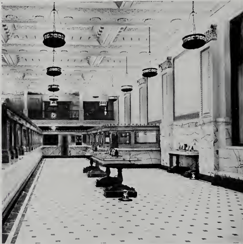
NIGHT PHOTOGRAPH OF THE UNION SAVINGS & TRUST COMPANY'S BANK. GROUND FLOOR HOGE BUILDING, SEATTLE, SHOWING THE EXCELLENT RESULT OF INDIRECT ILLUMINATION INSTALLED THEREIN.—C. H. BEBB, ARCHITECT
