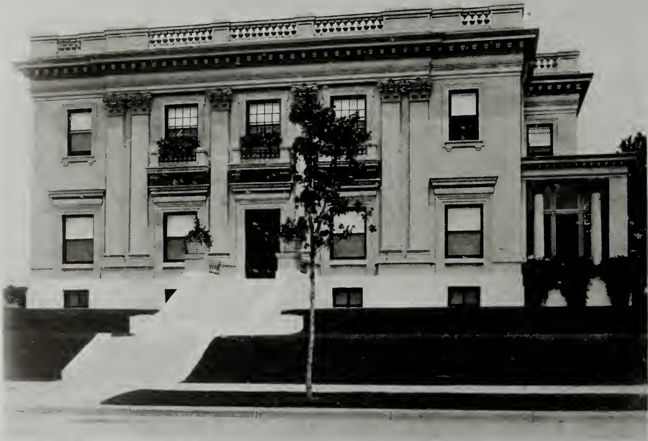
RESIDENCE HENRY ELLIOT, JR., ST. LOUIS BARNETT, HAYNES & BARNETT, ARCHITECTS HYDRAULIC PRESSED BRICK
