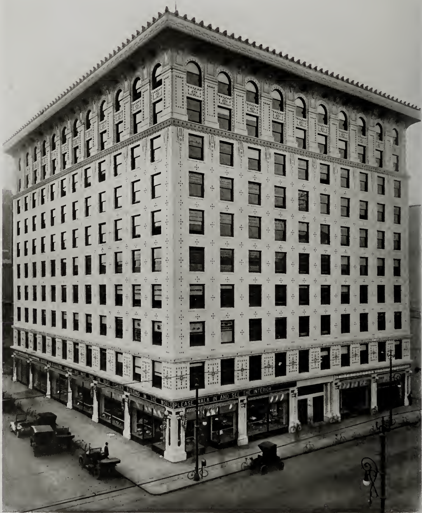
DENVER GAS & ELECTRIC BUILDING F. E. EDBROOKE, ARCHITECT
