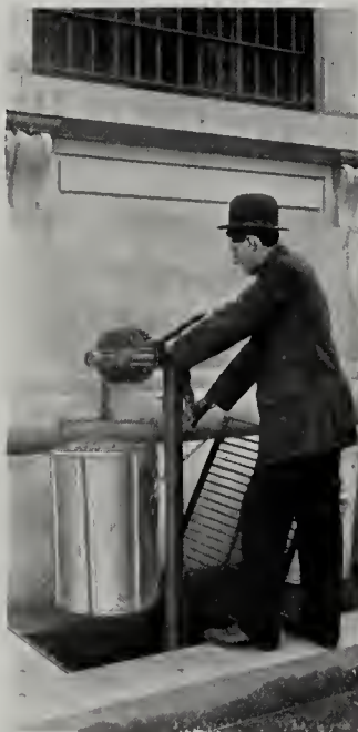
Hoist in Operation
