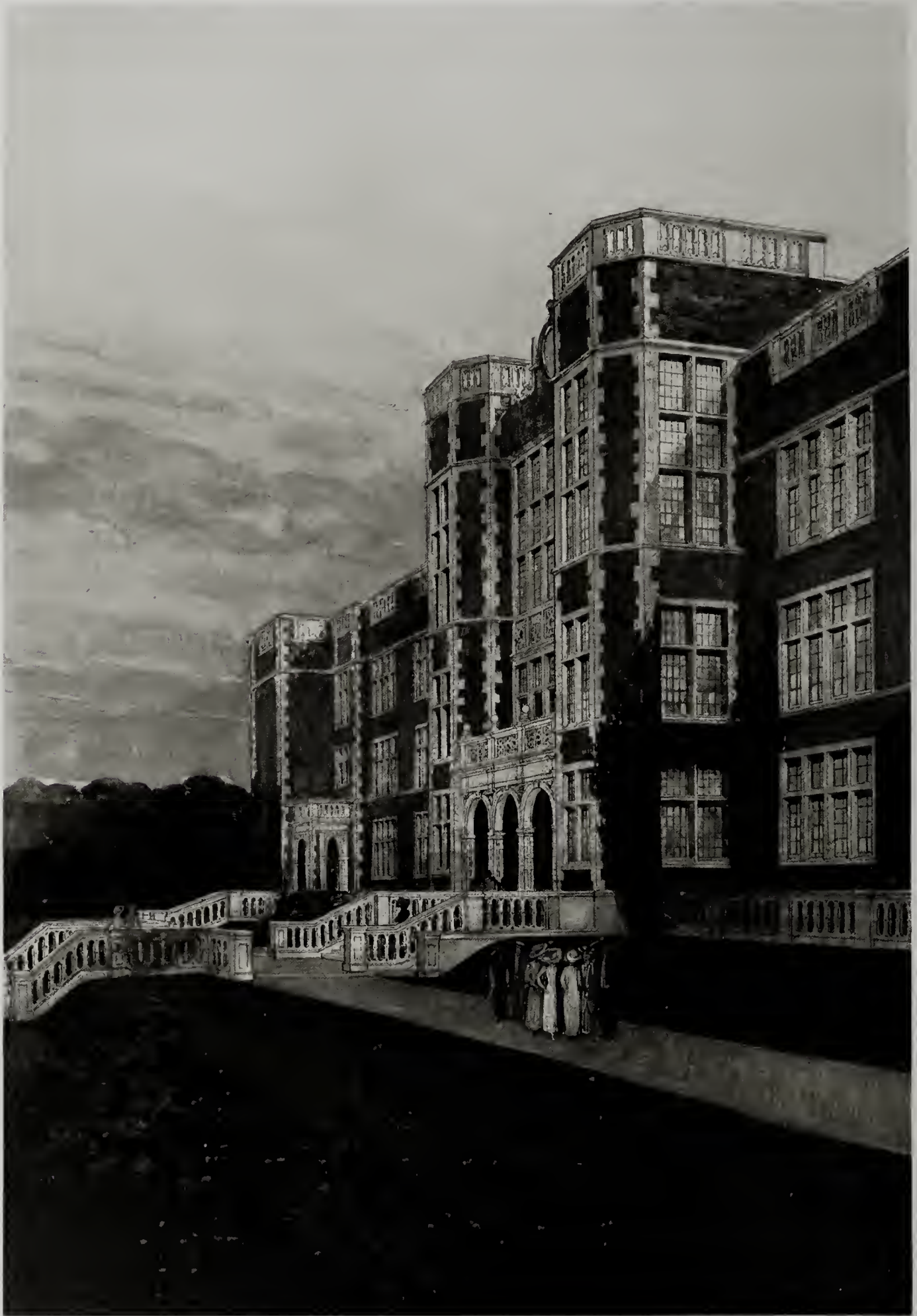
NEW CENTRAL HIGH SCHOOL, MINNEAPOLIS, MINNESOTA WILLIAM B. ITTNER, ARCHITECT, ST. LOUIS, MISSOURI
