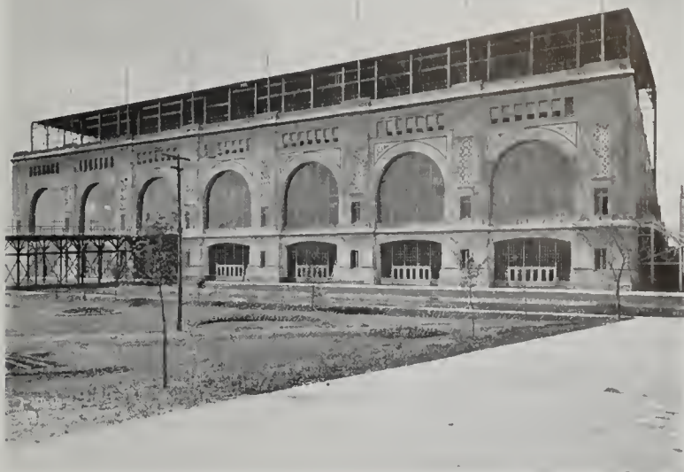
GRANDSTAND MINNESOTA STATE FAIR CLARENCE JOHNSTON, ARCHITECT
