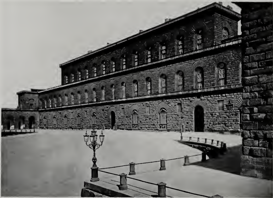
PLAZZA PITTE AT FLORENCE EXAMPLE OF POWERFUL OLD ARCHITECTURE
