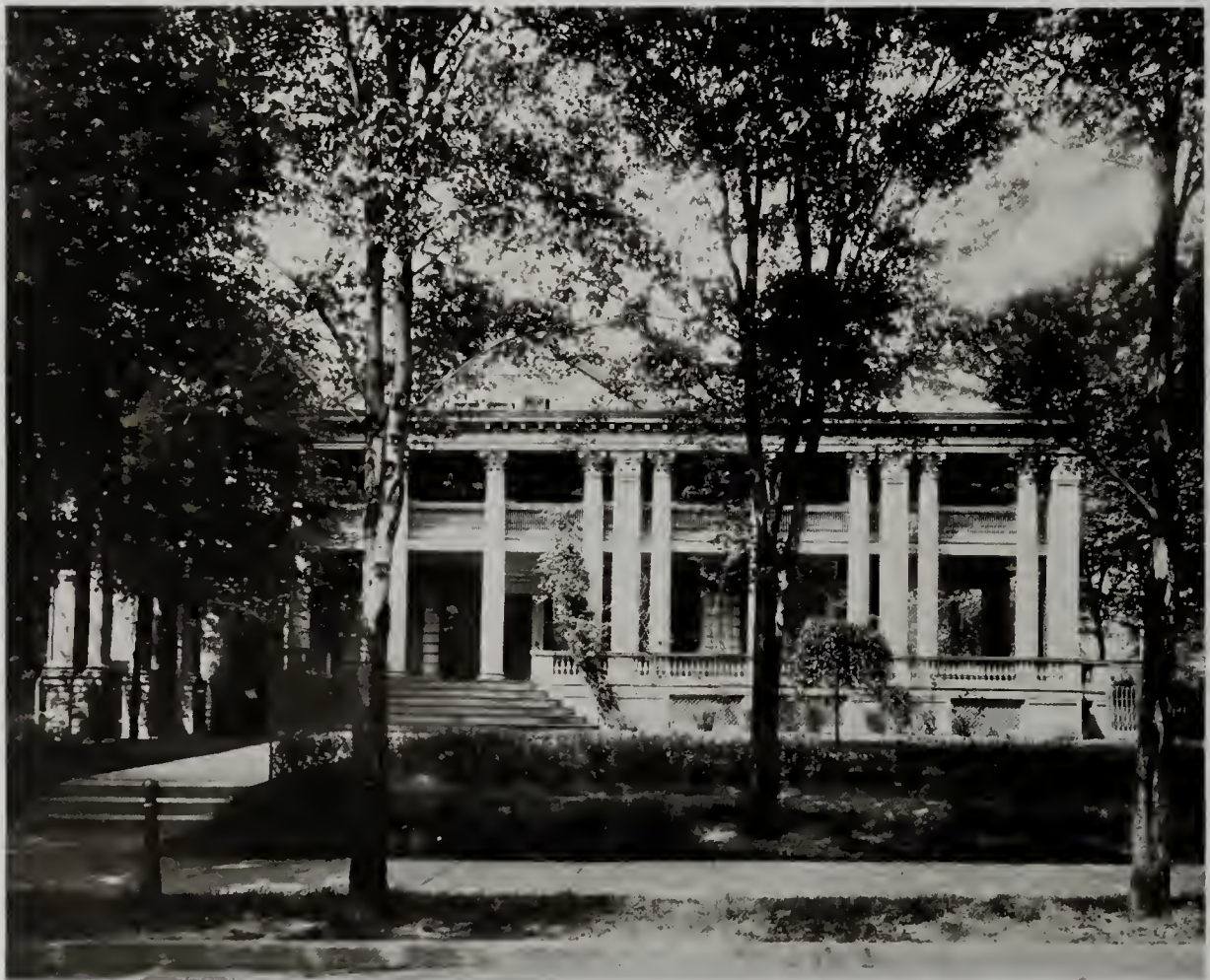
RESIDENCE MOSES GREENWOOD, ST. LOUIS BARNETT, HAYNES & BARNETT, ARCHITECTS
