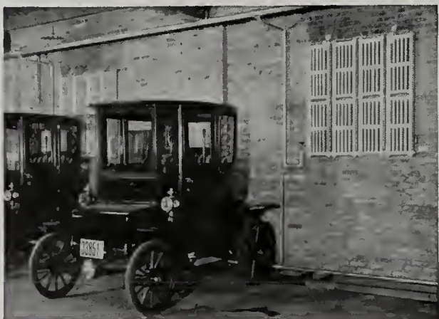
AMERICAN Rococo Wall Radiators in Lange Garage, Chicago Note the neat units or panels—effective but out of the way
