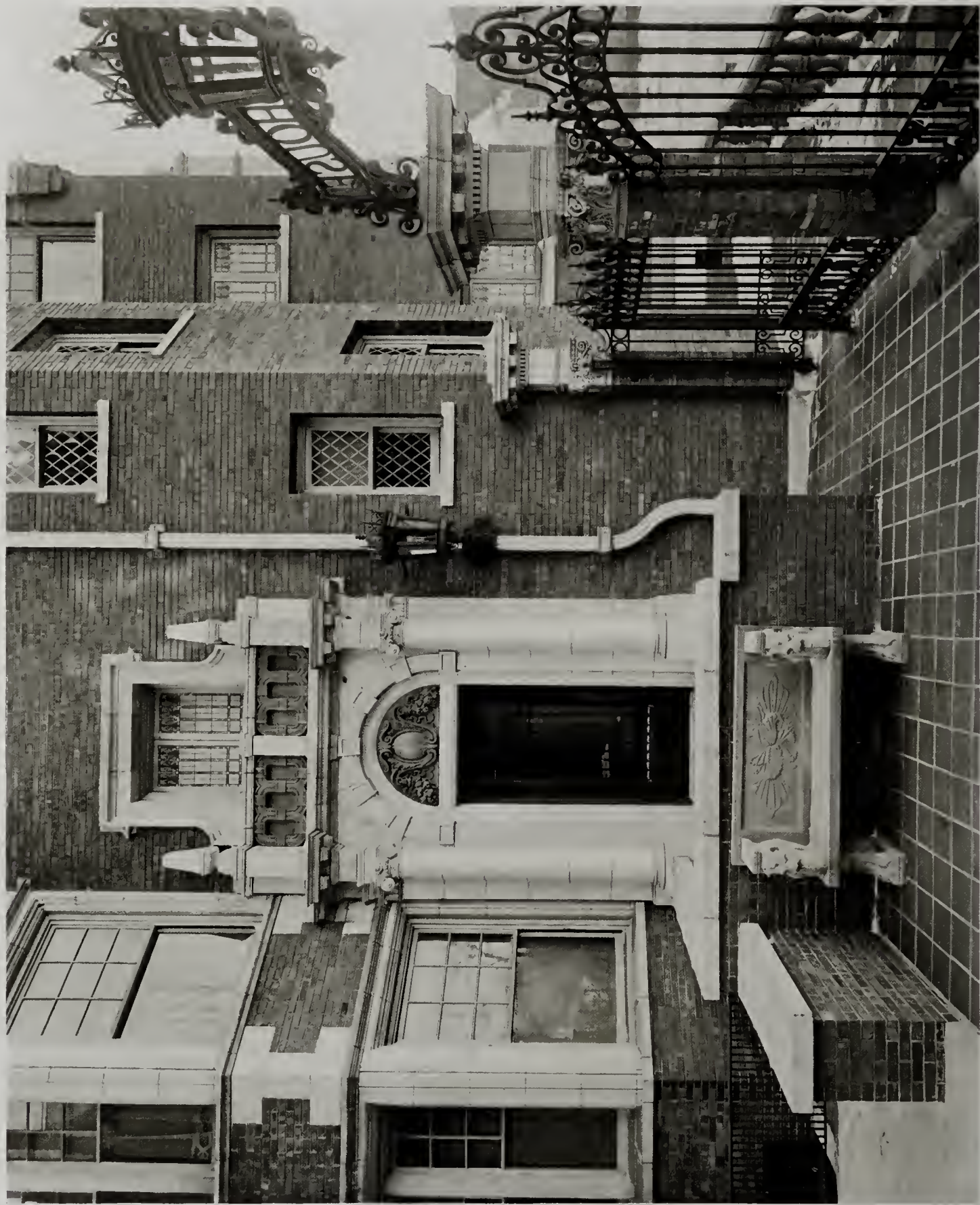
ENTRANCE DETAIL MANOR HOUSE APARTMENT, CHICAGO, ILLINOIS J. E. O. PRIDMORE, ARCHITECT
