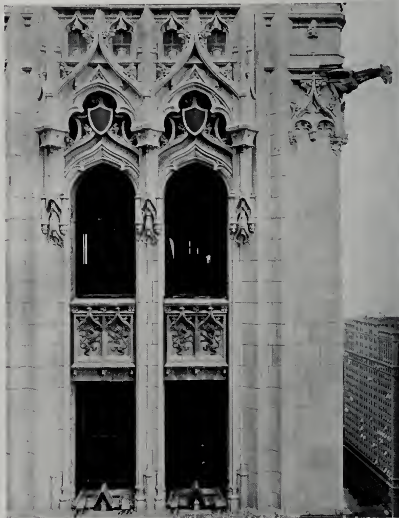
WOOLWORTH BUILDING DETAIL OF WINDOW AT THE TWENTY-SIXTH STORY OF THE COURT The inter-window panels are modeled in golden yellow against backgrounds of four colors; the shields over the windows are true gold. In the lower right hand corner is seen the Hudson-Terminal Bldgs., a Terra Cotta contract second in size to the Woolworth Bldg.
