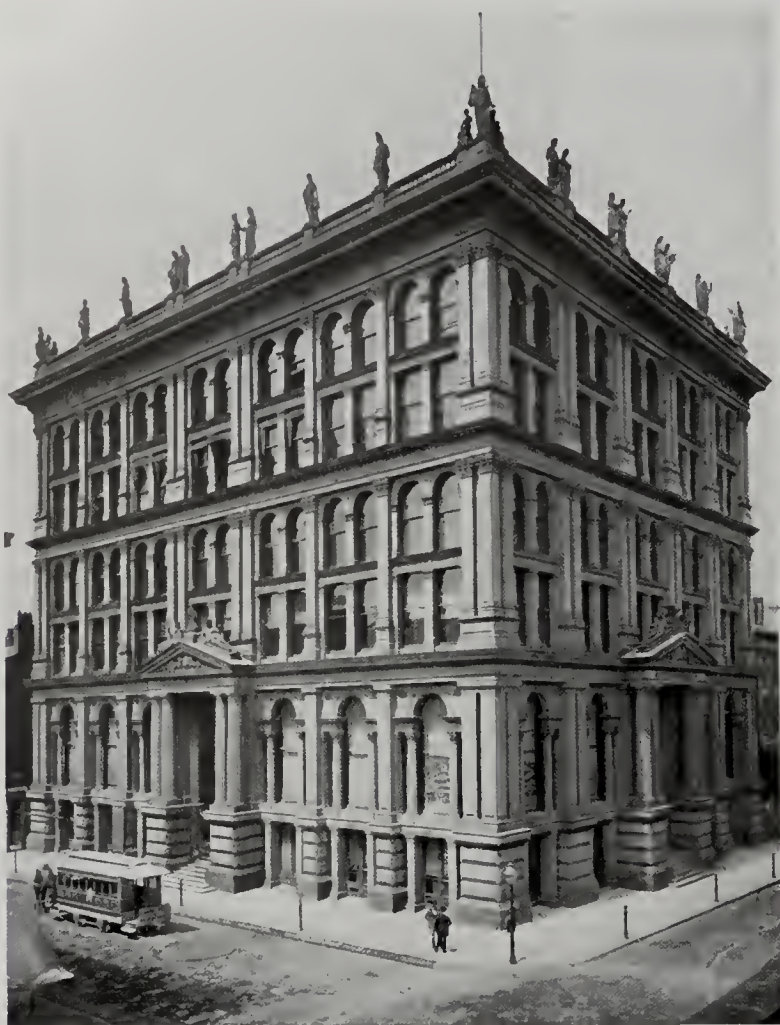
EQUITABLE BUILDING, ST. LOUIS, MISSOURI
