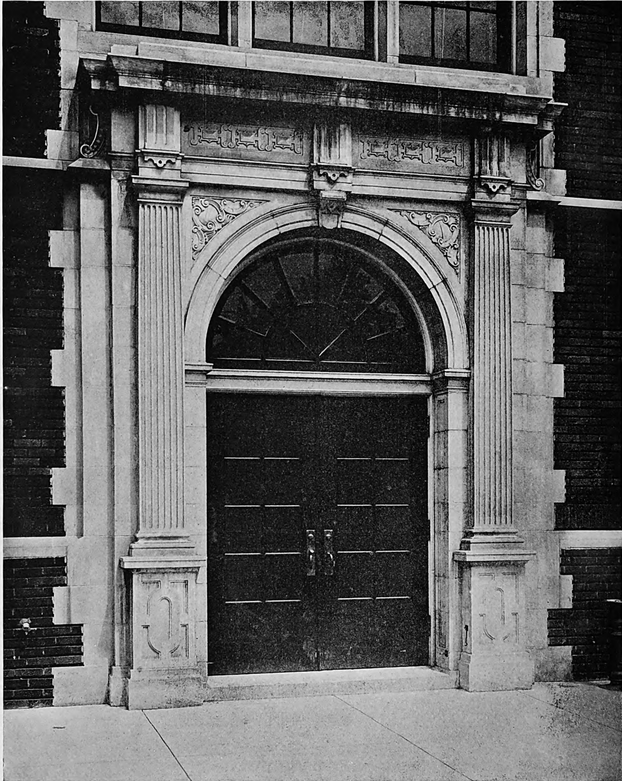
ENTRANCE DETAIL :: :: :: :: :: BOYS' HIGH SCHOOL, LOUISVILLE, KENTUCKY J. EARL HENRY, ARCHITECT :: :: :: ::
