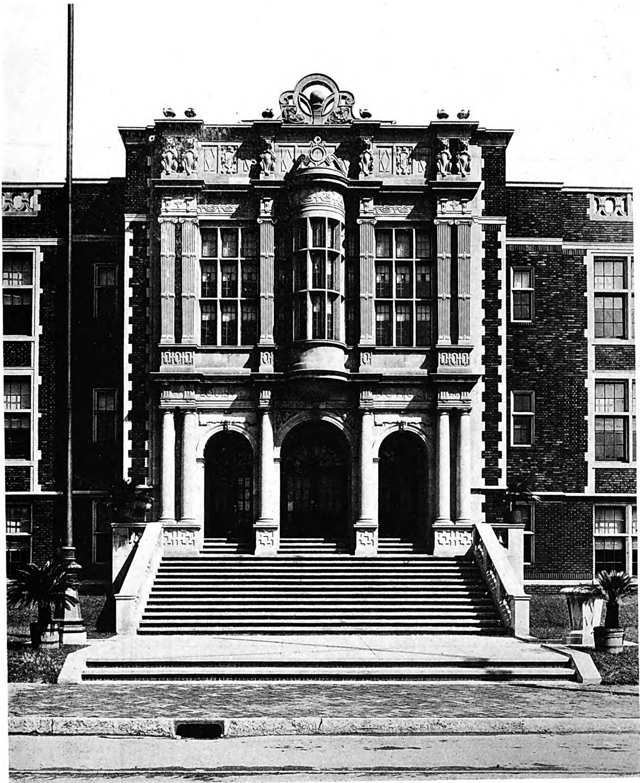
ENTRANCE DETAIL :: :: :: :: :: BOYS' HIGH SCHOOL, LOUISVILLE, KENTUCKY J. EARL HENRY, ARCHITECT :: :: :: ::
