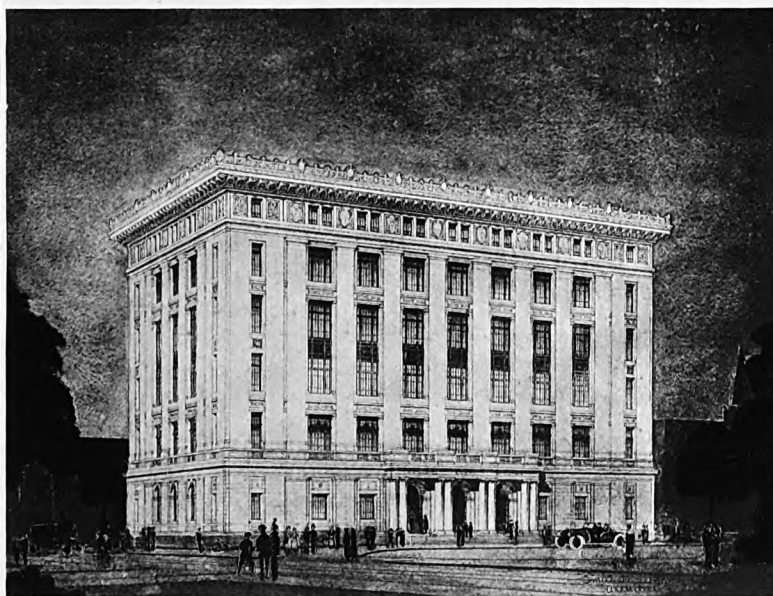
DETROIT MUNICIPAL COURT BUILDING. :: SMITH, HINCHMAN & GRYLLS, ARCHITECTS
