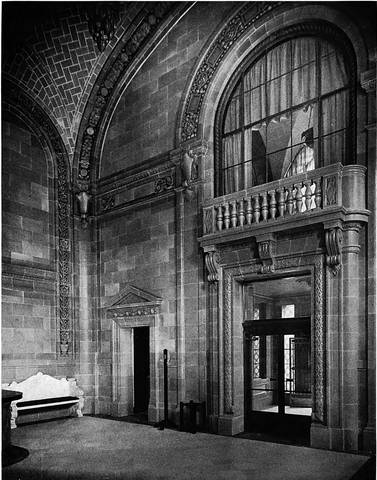
INTERIOR :: :: :: :: CITY NATIONAL BANK, EVANSVILLE, INDIANA MUNDIE & JENSEN, ARCHITECTS, CHICAGO, ILLINOIS
