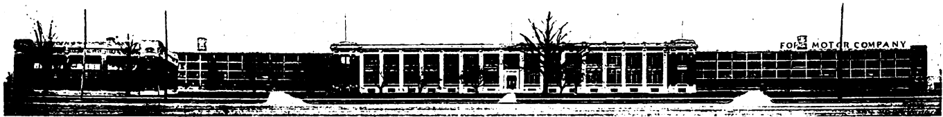
VIEW OF THE PLANT FOR FORD MOTOR COMPANY, DETROIT. ALBERT KAHN, ARCHITECT.
