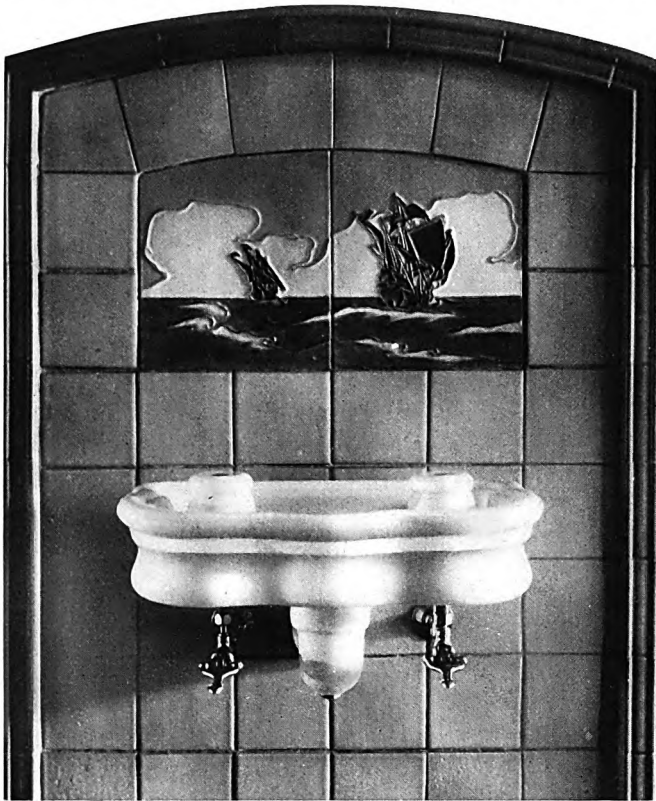
TYPICAL FOUNTAIN—McLAIN HIGH SCHOOL GREENFIELD, OHIO. W. B. ITTNER, ARCHITECT, ST. LOUIS
