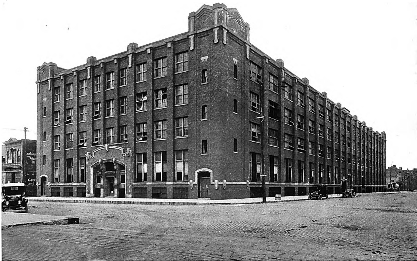
FACTORY BUILDING FOR A. H. WEINBRENNER COMPANY, MILWAUKEE, WIS. KIRCHOFF & ROSE, ARCHITECTS :: :: :: :: :: :: ::
