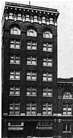
Building for Kunzelmann, Esser Company Kirchoff & Rose, Architects
