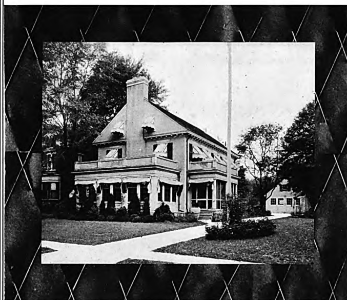
In this residence of Charles W. Oakley, Elizabeth, N. J., Charles W. Oakley, Architect, E-Cod Fabric was used as the plastering base.
