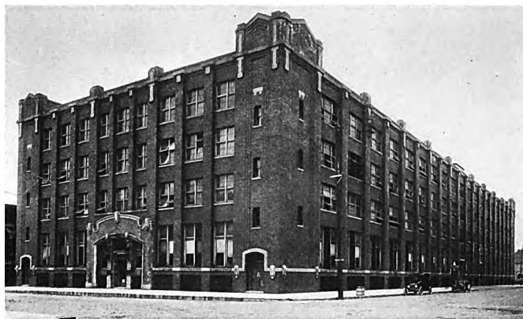
Factory Building for A. H. Weinbrenner Company Kirchoff & Rose, Architects
