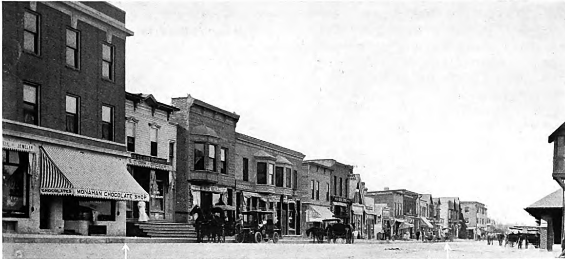
The Business District of Lake Forest, Illinois, (Western Avenue) as it was six years ago. The New Market Square improvement began by the wrecking of all fronts between the points marked.
