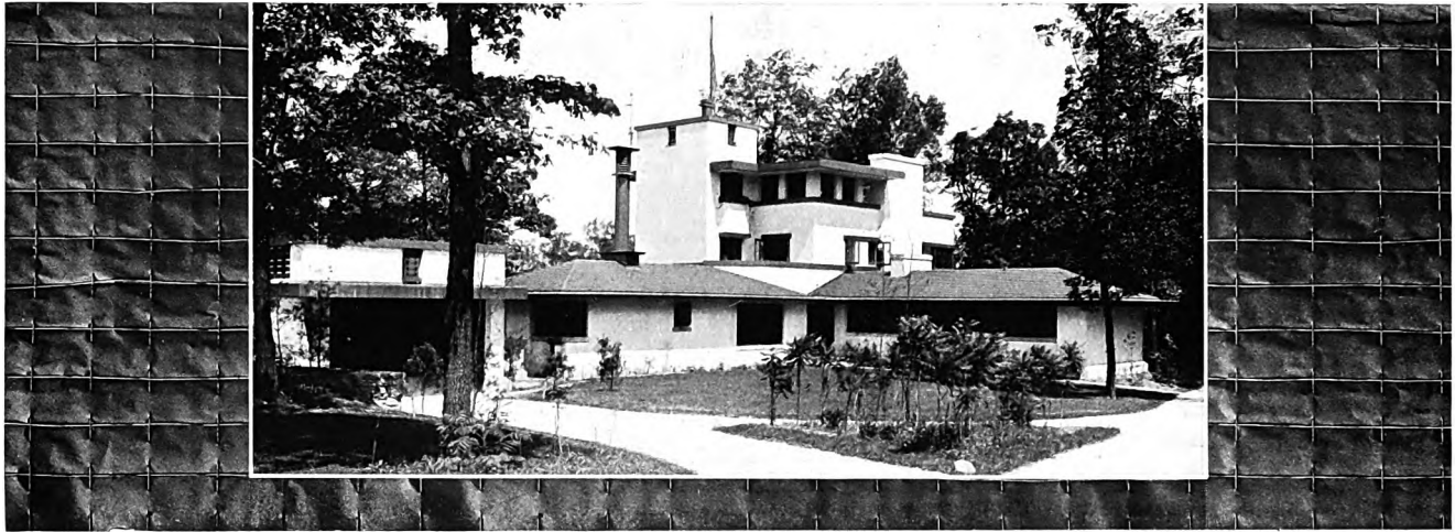
Residence for Sherman Booth, Glencoe, Illinois Frank Lloyd Wright, Architect Exterior Plastered on E-Cod Fabric
