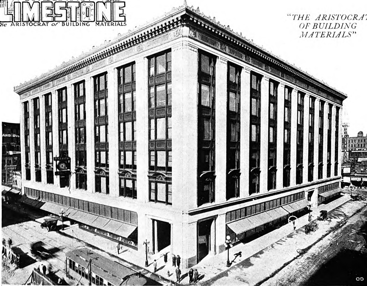
Indiana Limestone in the Golden Rule Department Store, St. Paul, Minn.—C. H. Johnston, Architect.
