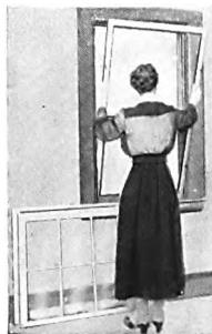
Taking Out Storm Sash Inside
