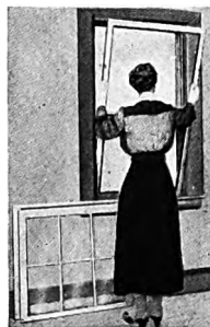
Taking Out Storm Sash Inside
