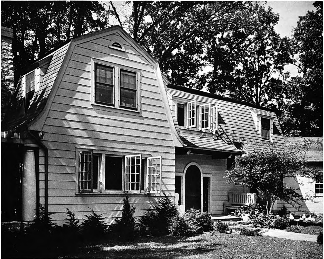
DETAIL OF ENTRANCE
