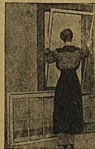
Taking Out Storm Sash Inside
