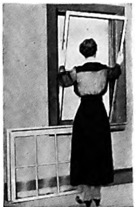
Taking Out Storm Sash Inside
