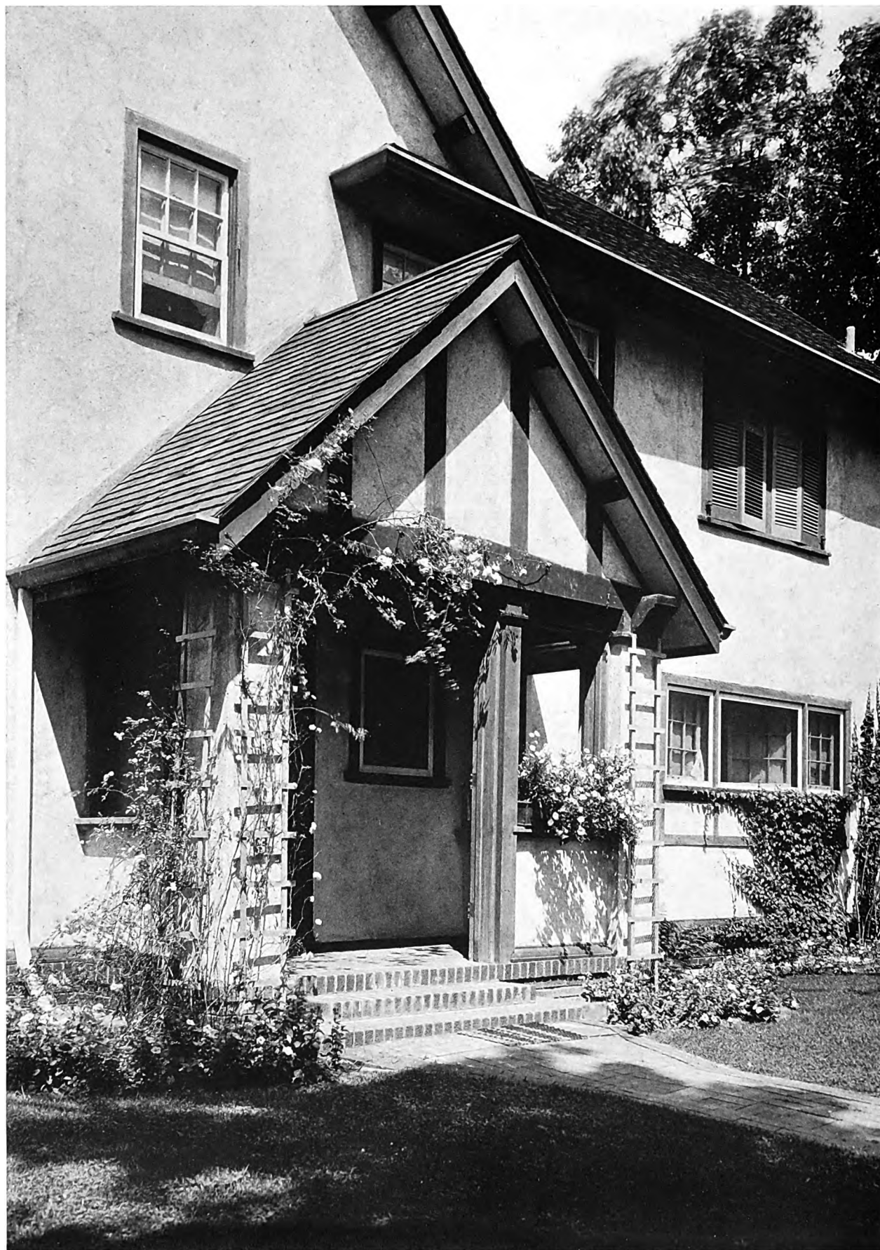
DETAIL OF ENTRANCE
