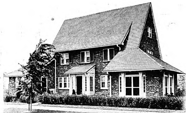
IMPERIAL CLOSED SHINGLE TILE Grosvenor Atterbury, New York, Architect
