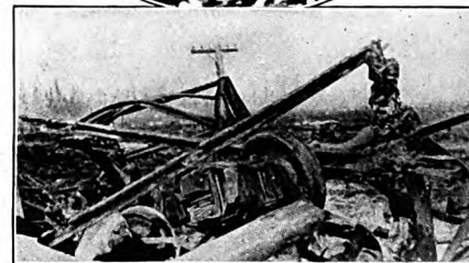
The photos above, taken after the great fire had passed through Iroquois Falls, give some idea of the terrific heat all around the Abitibi Pulp & Paper Co. plant. Note the bent and twisted steel rails and frame-work.
