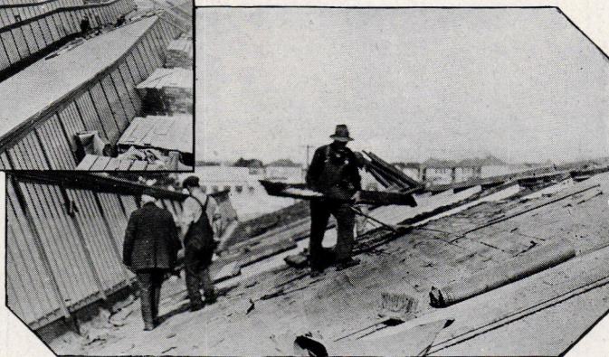
Saw-tooth roof Whitman Weaving Mill, New Bedford. Rotted boards replaced with long-lived Redwood
