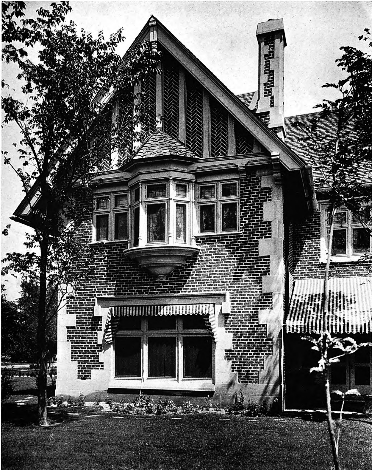
DETAIL OF GABLE HOUSE AT 360 HIGH STREET, DENVER, COLORADO J. B. BENEDICT, ARCHITECT :: :: :: :: :: :: (Note similar motif on Mountain Lodge for Mrs. Paul T. Mayo)
