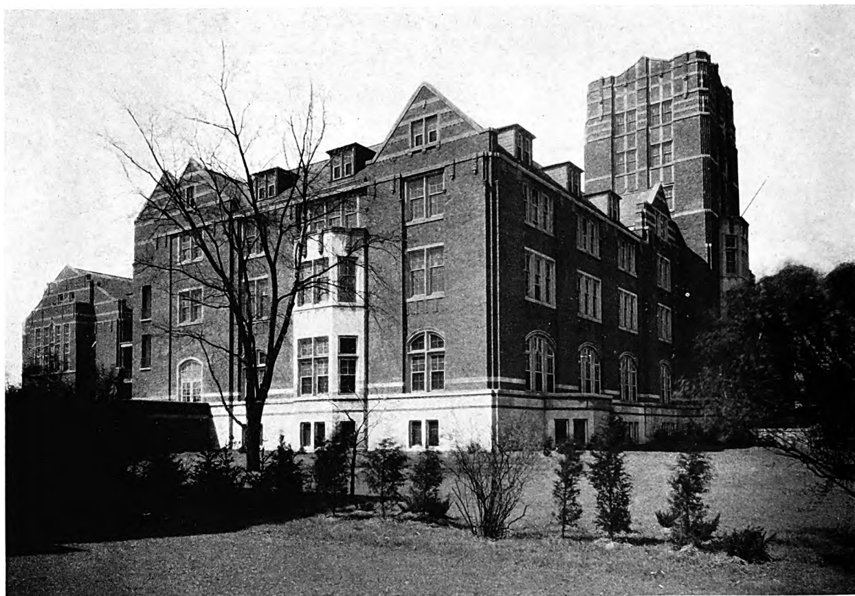
VIEW FROM THE SOUTHEAST
