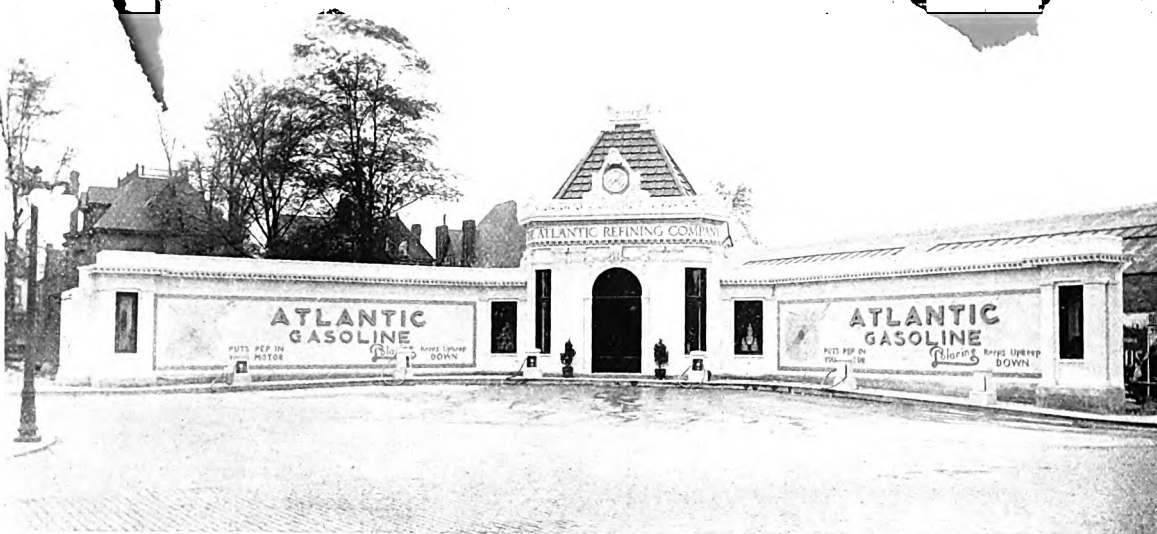
FILLER STATION OF WHITE MAT TERRA COTTA, FOR ATLANTIC REFINING COMPANY, AT WILKINSBURG, PENNSYLVANIA. G. W. WILKINS COMPANY, ARCHITECTS. FENCE ALSO OF TERRA COTTA.
