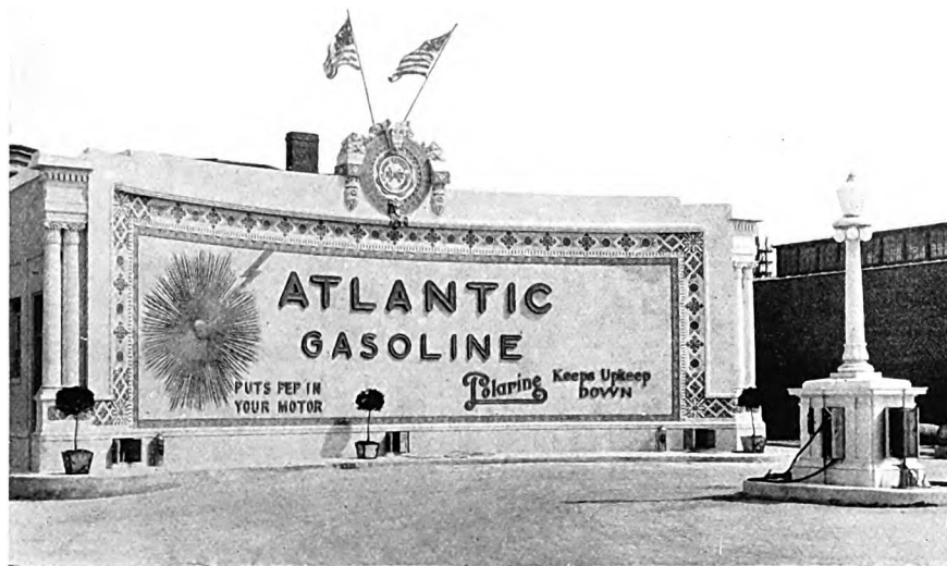
FILLER STATION FOR ATLANTIC REFINING COMPANY, FRANKFORD, PHILADELPHIA, OF WHITE MAT TERRA COTTA. FLASH ON SIGN IS RED, WITH CENTER OF PURE CERAMIC GOLD.
