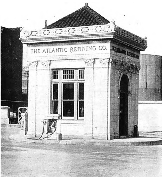
FILLER STATION FOR ATLANTIC REFINING COMPANY, ERIE, PENNSYLVANIA. JOSEPH FRANKLIN KUNZ, ARCHITECT.
