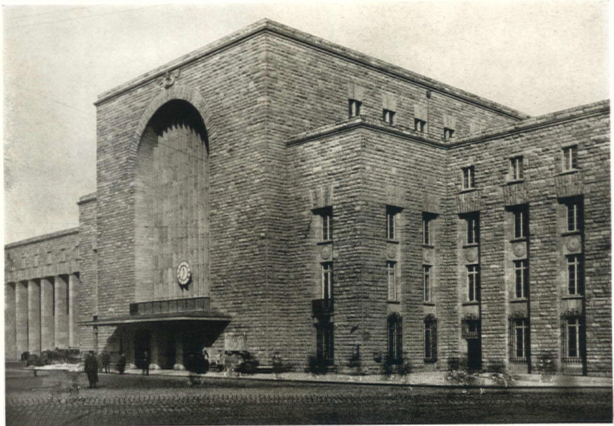
DETAIL OF STATION FRONT RAILWAY STATION, STUTTGART, GERMANY PROFESSOR PAUL BONATZ AND F. E. SCHOLER, ARCHITECTS
