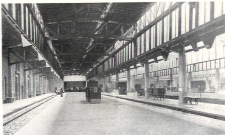
MAIN SHED IN THE STATION AT STUTTGART
