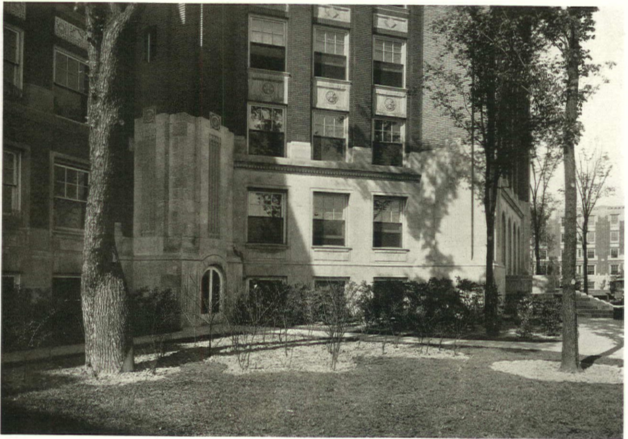
DETAIL OF CENTRAL PAVILION HENRY FORD HOSPITAL, DETROIT, MICHIGAN ALBERT WOOD, ARCHITECT :: :: :: :: ::
