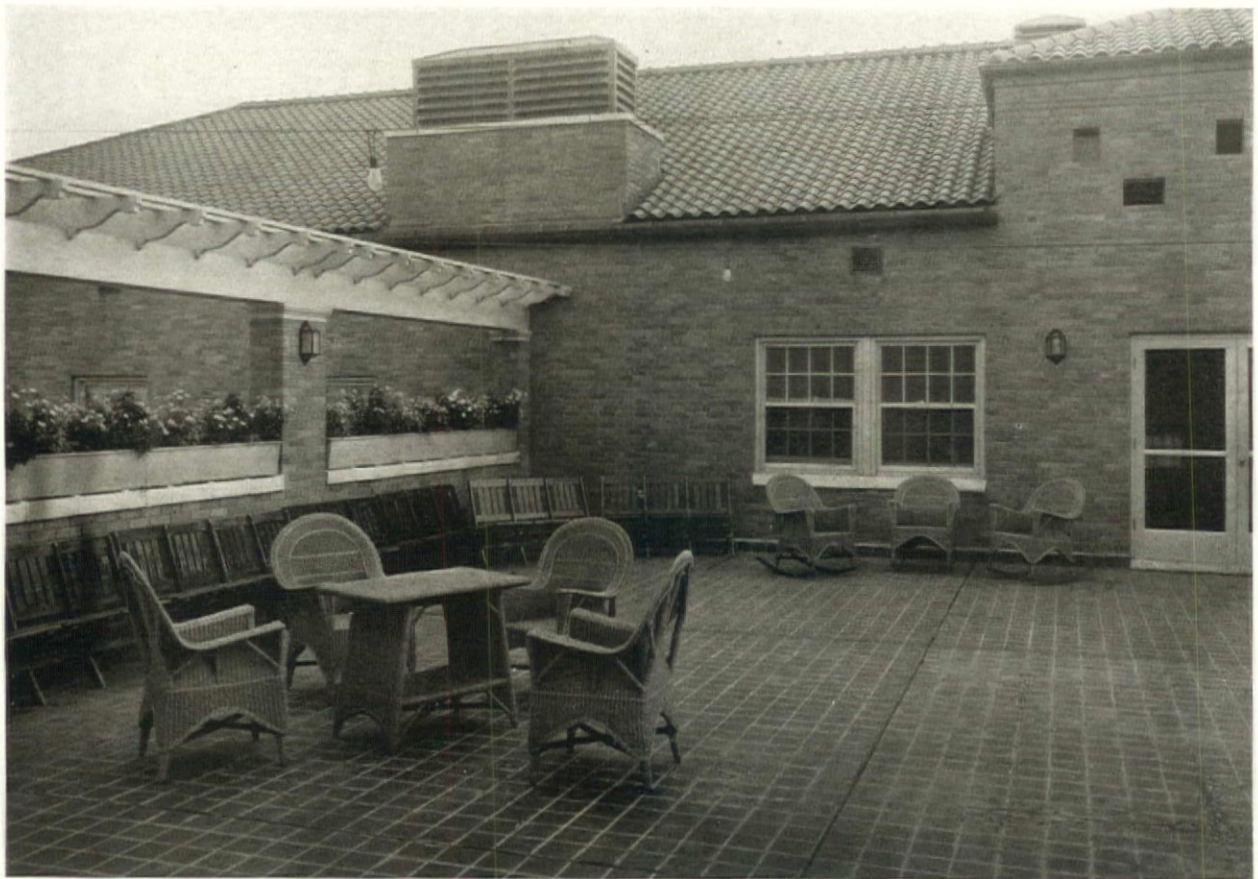
ROOF GARDEN YOUNG MEN'S HEBREW ASSOCIATION, KANSAS CITY, MISSOURI GREENEBAUM, HARDY AND SCHUMACHER, ARCHITECTS :: ::
