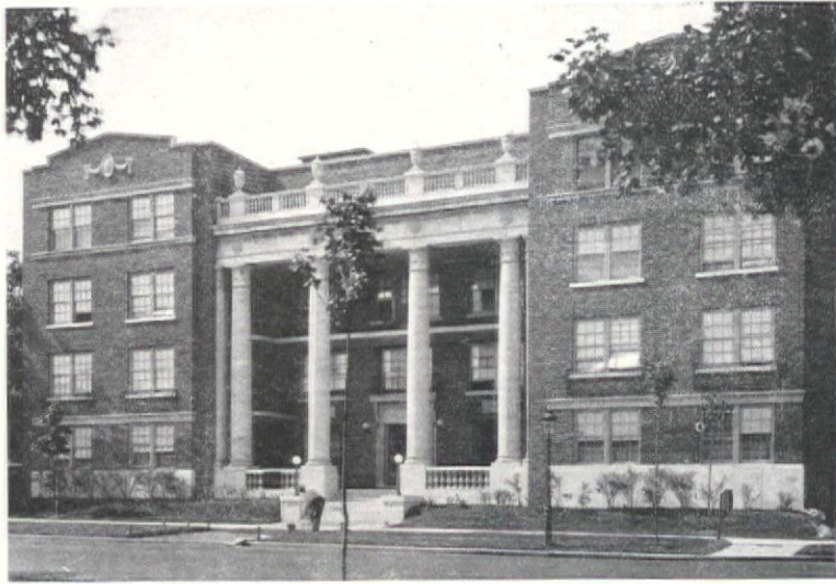
THE GOTHAM APARTMENT HOTEL, KANSAS CITY; GREENEBAUM, HARDY AND SCHUMACHER, ARCHITECTS.
