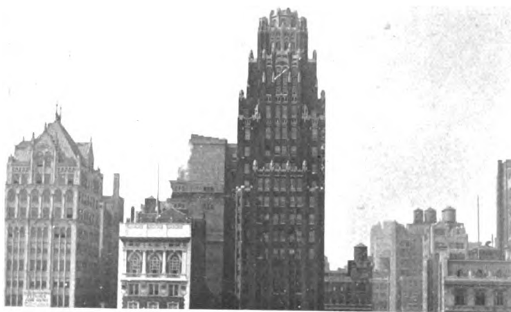
THE AMERICAN RADIATOR BUILDING OUTLINED AGAINST THE SKY
