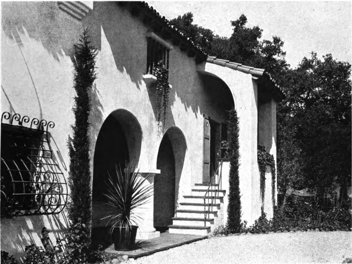
DETAIL OF ENTRANCE STAIRWAY
