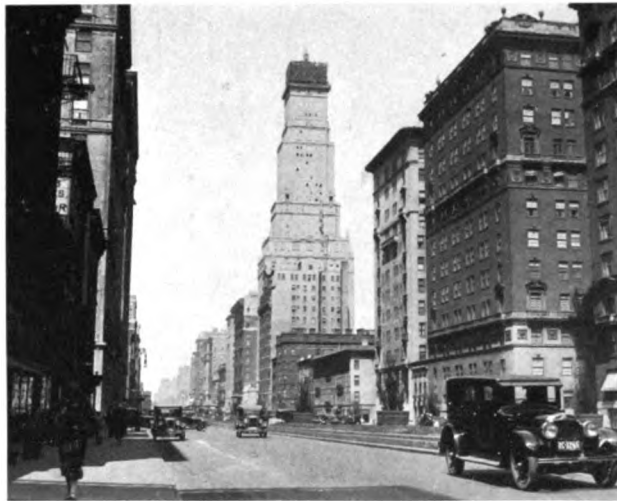
THE RITZ TOWER UNDER CONSTRUCTION, EMERY ROTH, ARCHITECT.
