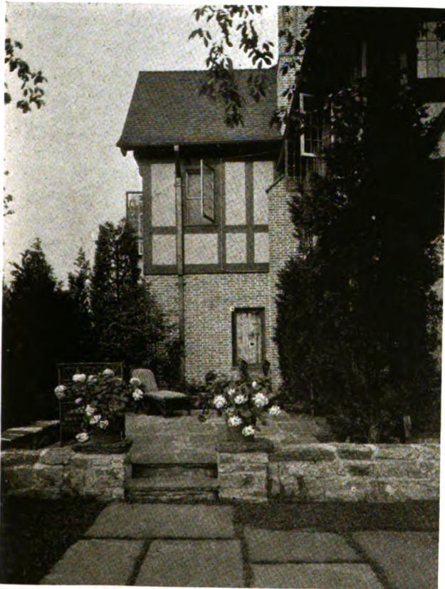
DETAIL OF TERRACE ESTATE OF MR. Z. G. SIMMONS, GREENWICH, CONNECTICUT SIMONDS AND WEST, LANDSCAPE DESIGNERS, GREENWICH, CONNECTICUT
