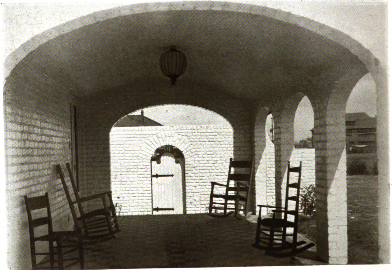
DETAIL OF PORCH RESIDENCE FOR MR. H. M. HOLDEN, HOUSTON, TEXAS J. W. NORTHROP, JR., A. I. A., ARCHITECT :: :: ::
