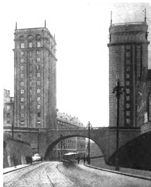
TWIN OFFICE BUILDINGS, STOCKHOLM.
