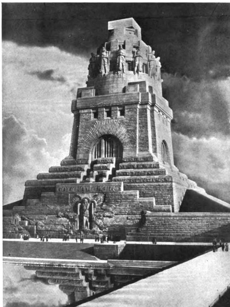
VOELKERSCHLACHT MONUMENT, LEIPSIG, BUILT TO COMMEMORATE THE BATTLE OF LEIPSIG. BRUNO SCHMITZ, ARCHITECT
