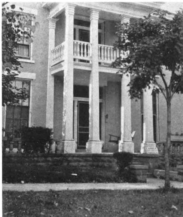
FIG. 6. THE TWO-STORY PORCH OF THE BOOK STORE AND HALL, BUILT IN 1840 BY JOSEPH HUTCHINS. THE STORE WAS NOTED BECAUSE IT SPECIALIZED IN LAW BOOKS.
