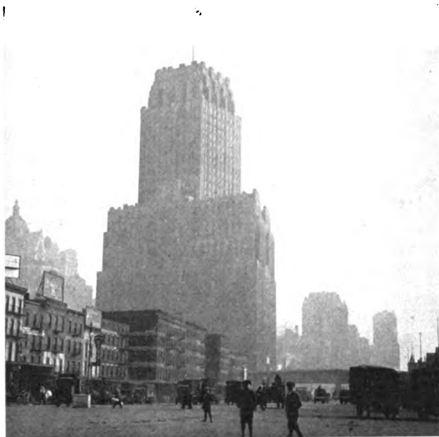
VIEW OF THE BARCLAY-VESEY BUILDING FOR THE NEW YORK TELEPHONE COMPANY FROM WEST STREET LOOKING SOUTH.
