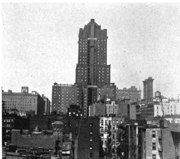
REAR VIEW OF THE SHELTON, FROM THE EAST
