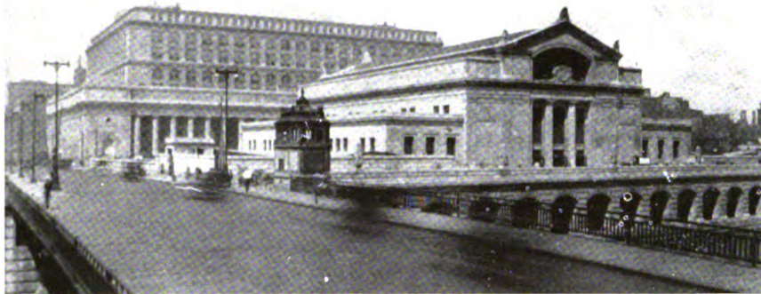
THE STATION FROM JACKSON BOULEVARD BRIDGE. THE HEAD HOUSE IN THE BACKGROUND WILL LATER RISE TO ITS FULL HEIGHT AS FOUNDATIONS SO PROVIDE.
