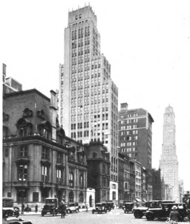
THE RITZ TOWER, EMERY ROTH, ARCHITECT, AT EXTREME RIGHT. BUILDING IN CENTER IS A NEW TYPE, NARROW BUILDING SET BACK BOTH FRONT AND REAR.
