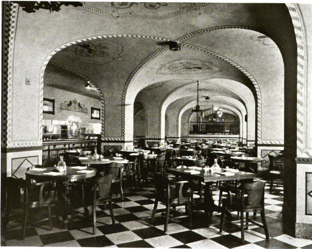
GRILLE. HOTEL PEABODY, MEMPHIS, TENNESSEE WALTER W. AHLSCHLAGER, ARCHITECT ::
