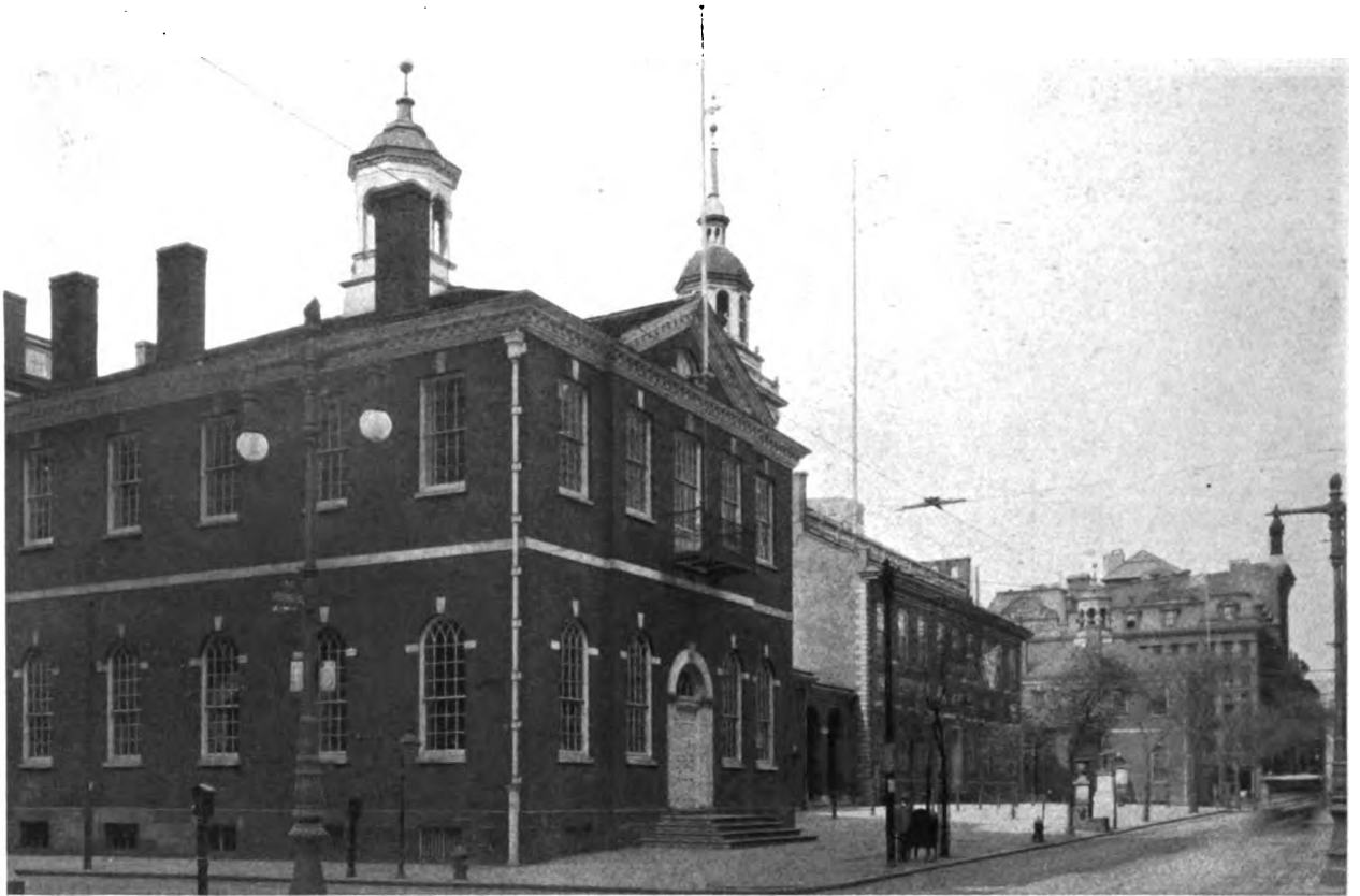
OLD CITY HALL (1791) IN FOREGROUND
