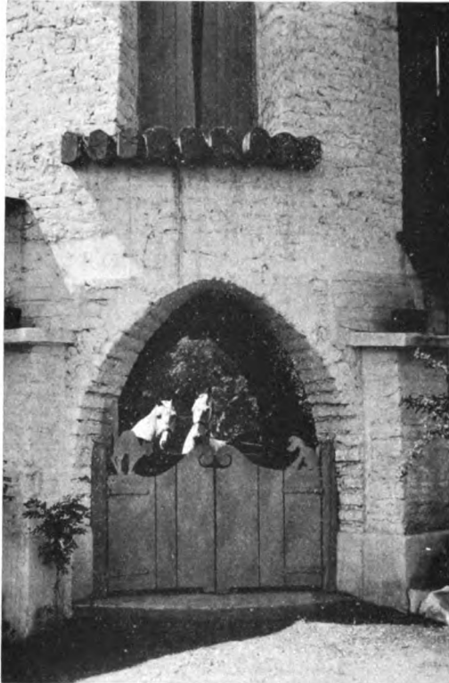
DETAIL OF GATE IN TOWER OF LIBBEY STABLES IN THE OJAI VALLEY, CALIFORNIA. WALLACE NEFF, ARCHITECT
