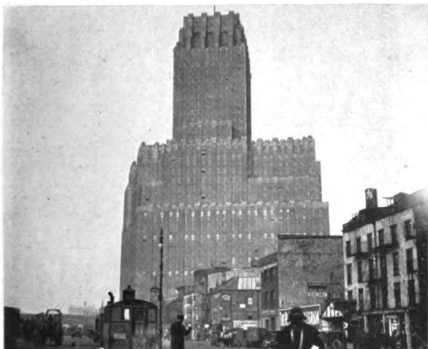
VIEW OF THE BARCLAY-VESEY BUILDING FOR THE NEW YORK TELEPHONE COMPANY TAKEN FROM WEST STREET, LOOKING NORTH.
