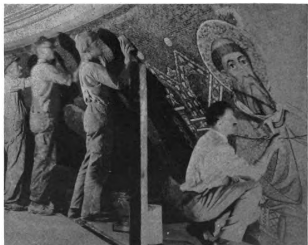
FIG. 6. INSTALLING THE MOSAIC IN PLACE.
