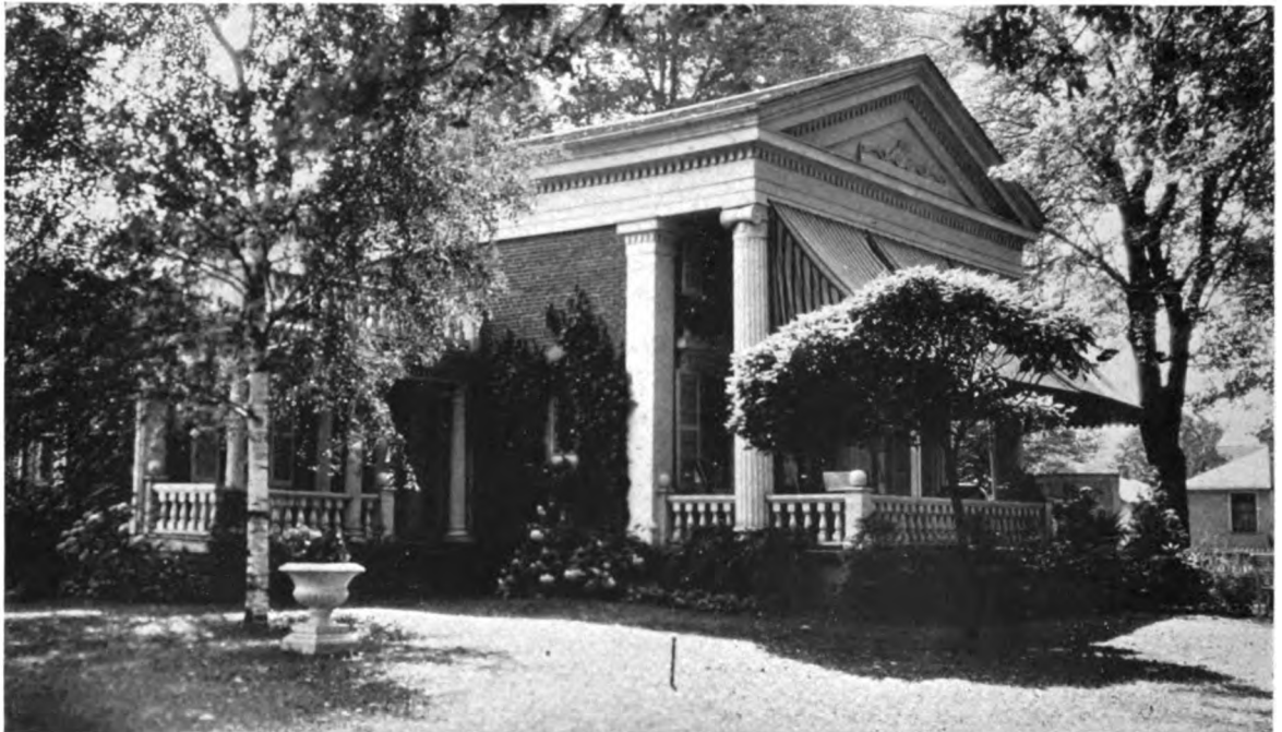
FIGURE 7. THE SMITH-TURNER HOUSE, MILAN, OHIO. VIEW SHOWING ONE-STORY WING ON NORTH SIDE.
