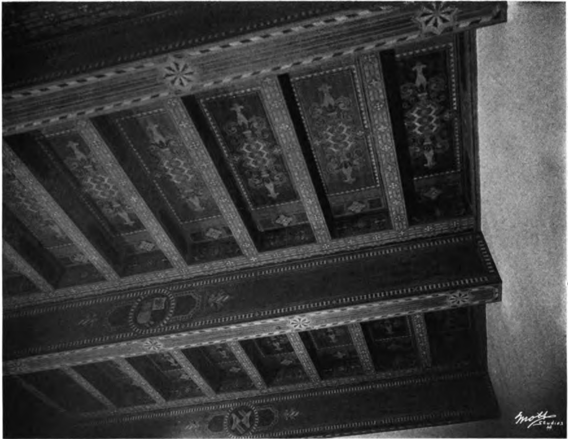
DETAIL OF CEILING IN REFERENCE ROOM
