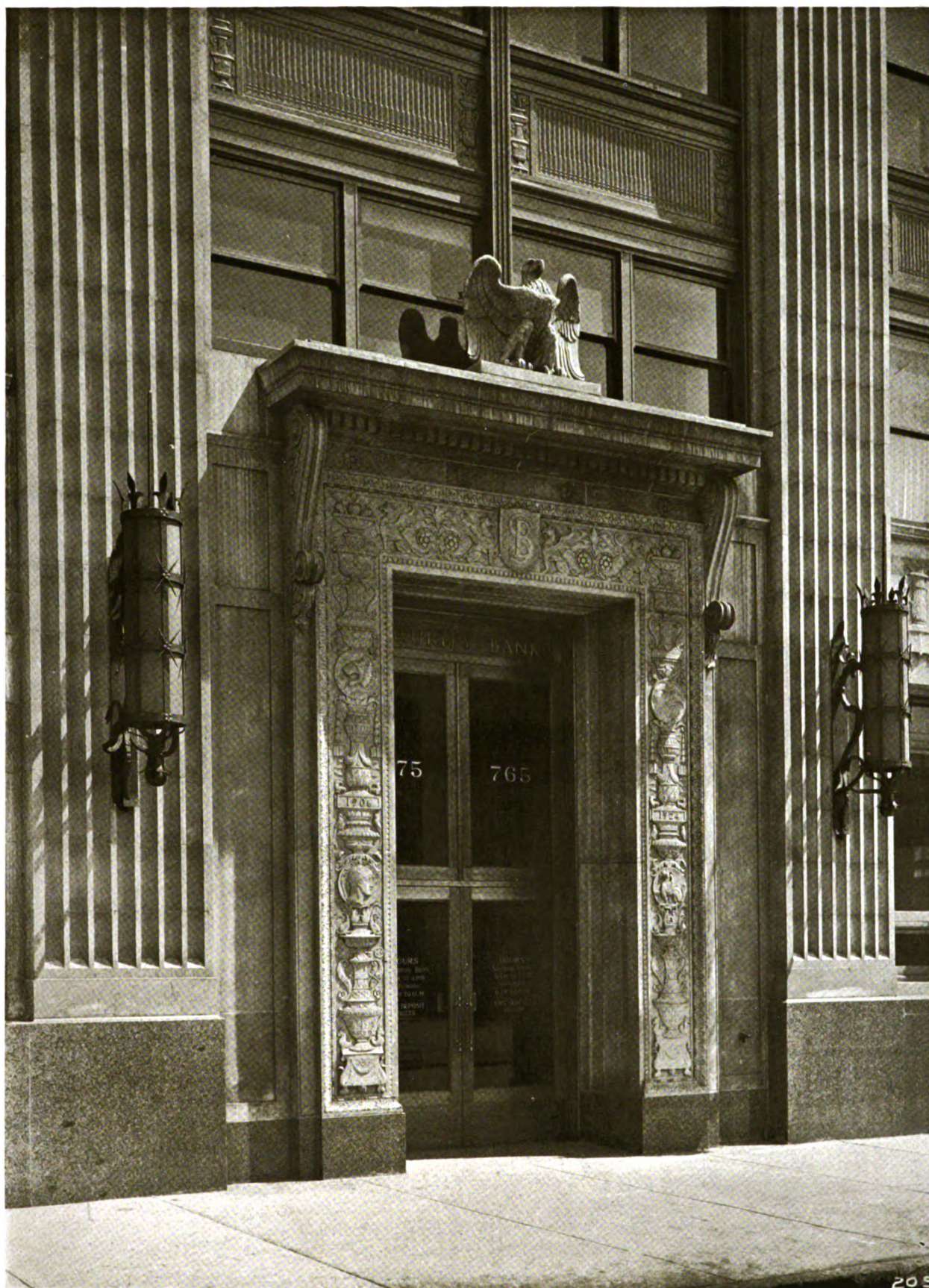
DETAIL OF ENTRANCE SECURITY BANK, CHICAGO CHILDS AND SMITH, ARCHITECTS
