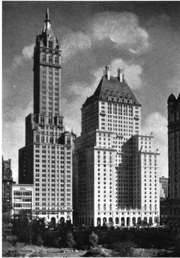
THE SAVOY-PLAZA, NEW YORK. McKIM, MEAD AND WHITE, ARCHITECTS. PHOTO BY AMEMYA.
