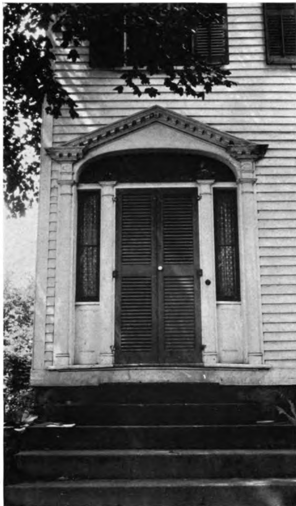
FIGURE 2. DOORWAY OF THE LOCKWOOD HOUSE, MILAN, OHIO. AN EARLY OHIO RENDERING OF A CONNECTICUT COLONIAL TYPE.
