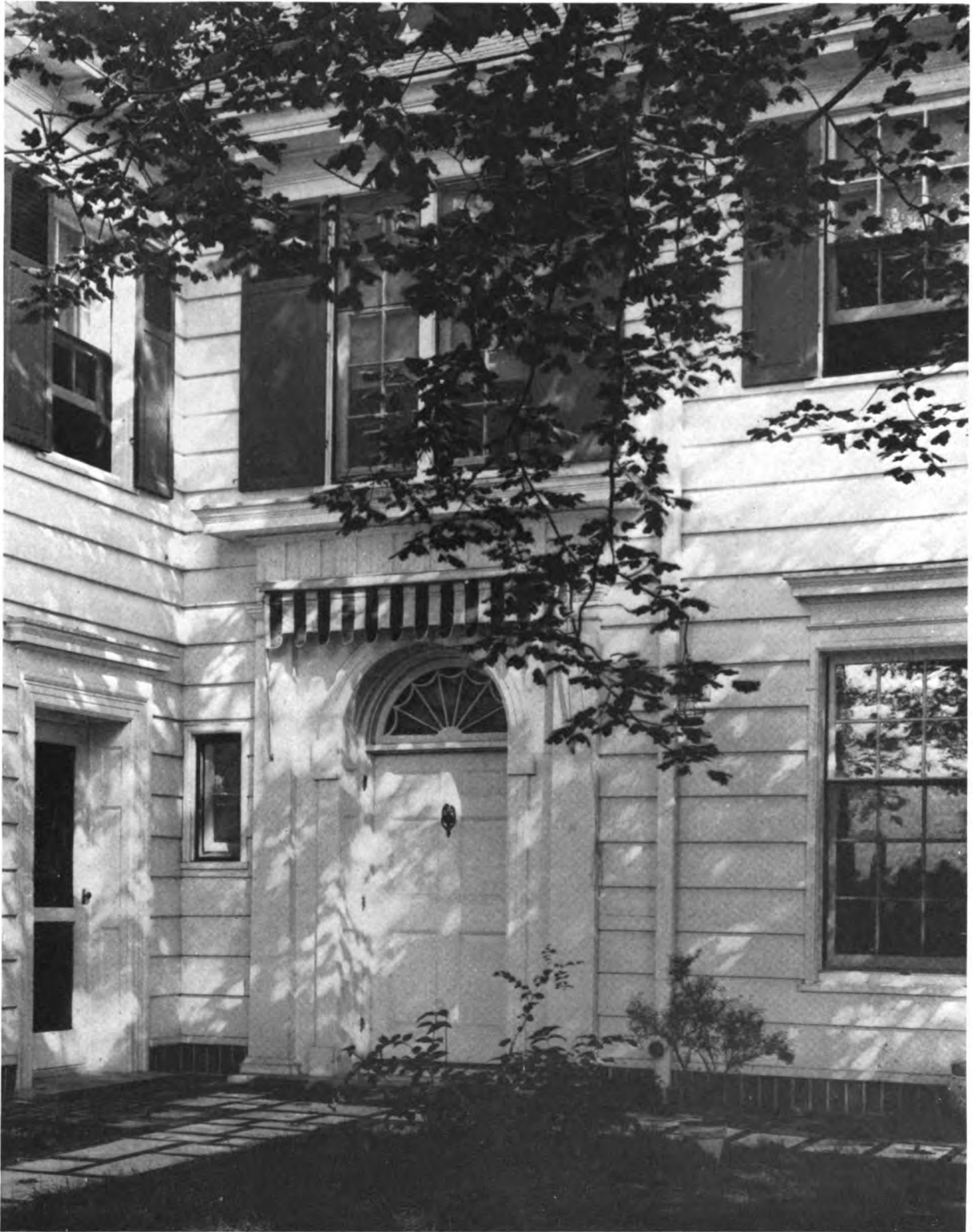
DETAIL OF MAIN ENTRANCE RESIDENCE FOR MR. WILLIAM H. COBURN, INDIANAPOLIS, INDIANA FREDERICK WALLICK, ARCHITECT
