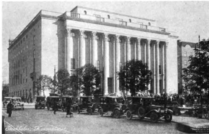
CONCERT HOUSE AT STOCKHOLM, SWEDEN, PROFESSOR IVAR TENGBOM, ARCHITECT.
