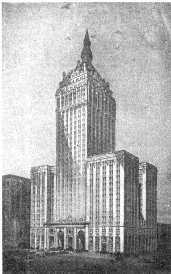
THIS BUILDING STRADDLES ONE OF NEW YORK'S MOST PROMINENT STREETS, ACTING AS AN APPARENT STREET TERMINAL ALTHOUGH VEHICULAR TRAFFIC PASSES THROUGH IT ON THE STREET LEVEL.
