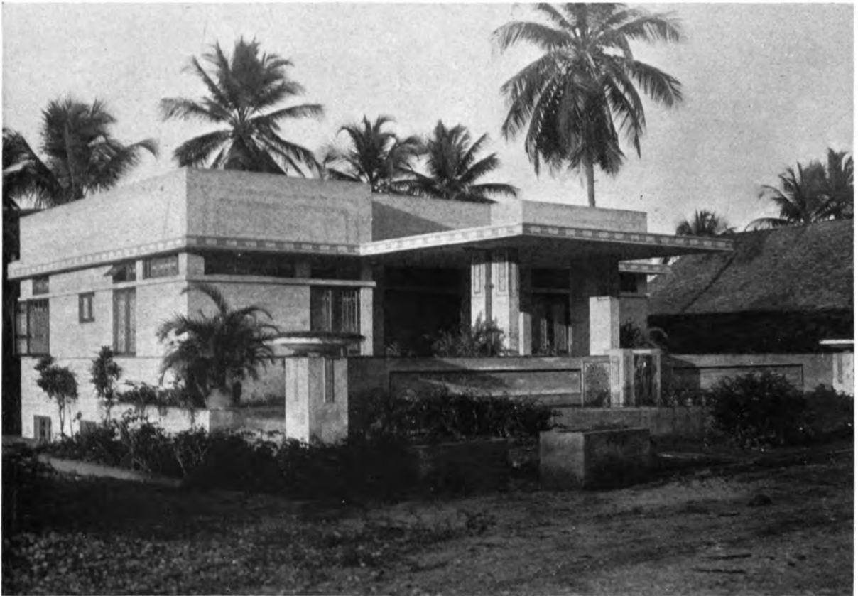
PEACOCK HOUSE, SAN JUAN, PORTO RICO ANTONIN NECHODOMA, ARCHITECT ::
