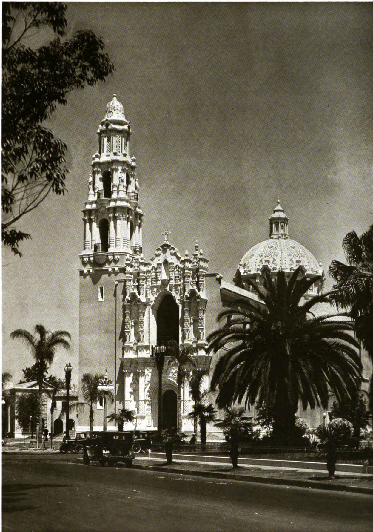
✓ GENERAL VIEW ST. VINCENT DE PAUL CATHOLIC CHURCH, LOS ANGELES, CALIFORNIA ALBERT C. MARTIN, ARCHITECT :: :: :: :: :: :: :: ::
