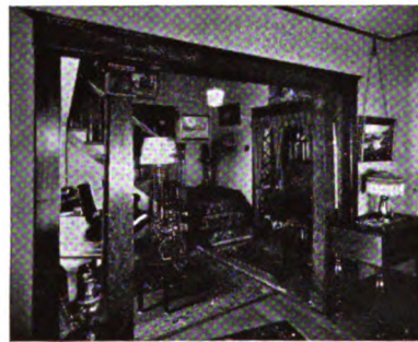
As tained flat-grain durable Douglas Fir interior—18 years old.
