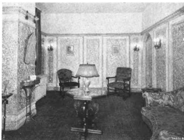
FIG. 2. LIVING ROOM OF TWO-ROOM APARTMENT, SHOWING WALL PANELS ON REAR OF WHICH BEDS ARE FASTENED
