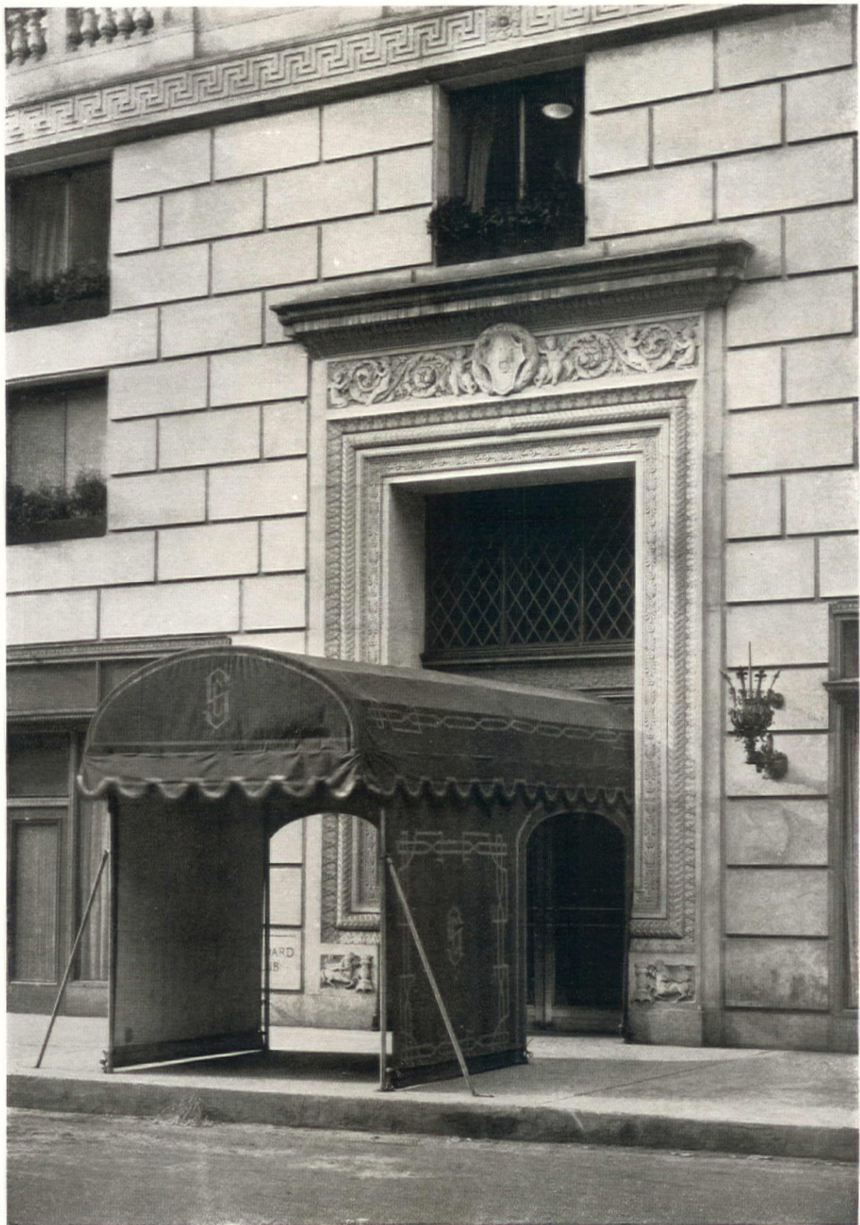
PLYMOUTH COURT ENTRANCE THE STANDARD CLUB, CHICAGO, ILLINOIS ALBERT KAHN, INCORPORATED, ARCHITECTS
