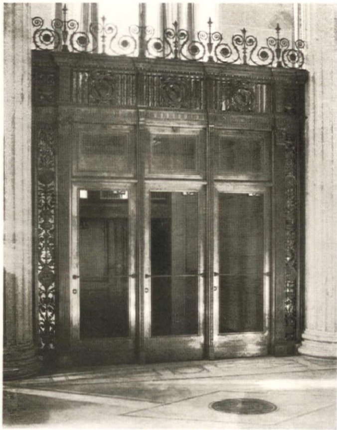
DETAIL OF DOOR HIBERNIA BANK AND TRUST COMPANY, NEW ORLEANS, LOUISIANA FAVROT AND LIVAUDAIS, LIMITED, ARCHITECTS :: :: :: :: ::
