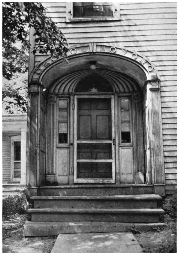
THE VERY UNUSUAL DOORWAY OF THE PROFESSOR'S HOUSE. IT IS OF THE RECESSED TYPE AND HAS SOME INTERESTING DECORATIVE DETAILS
