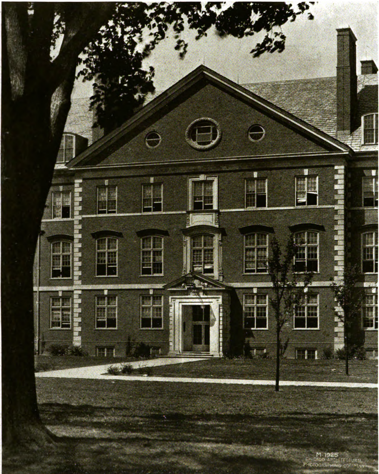
DETAIL OF EAST FACADE
