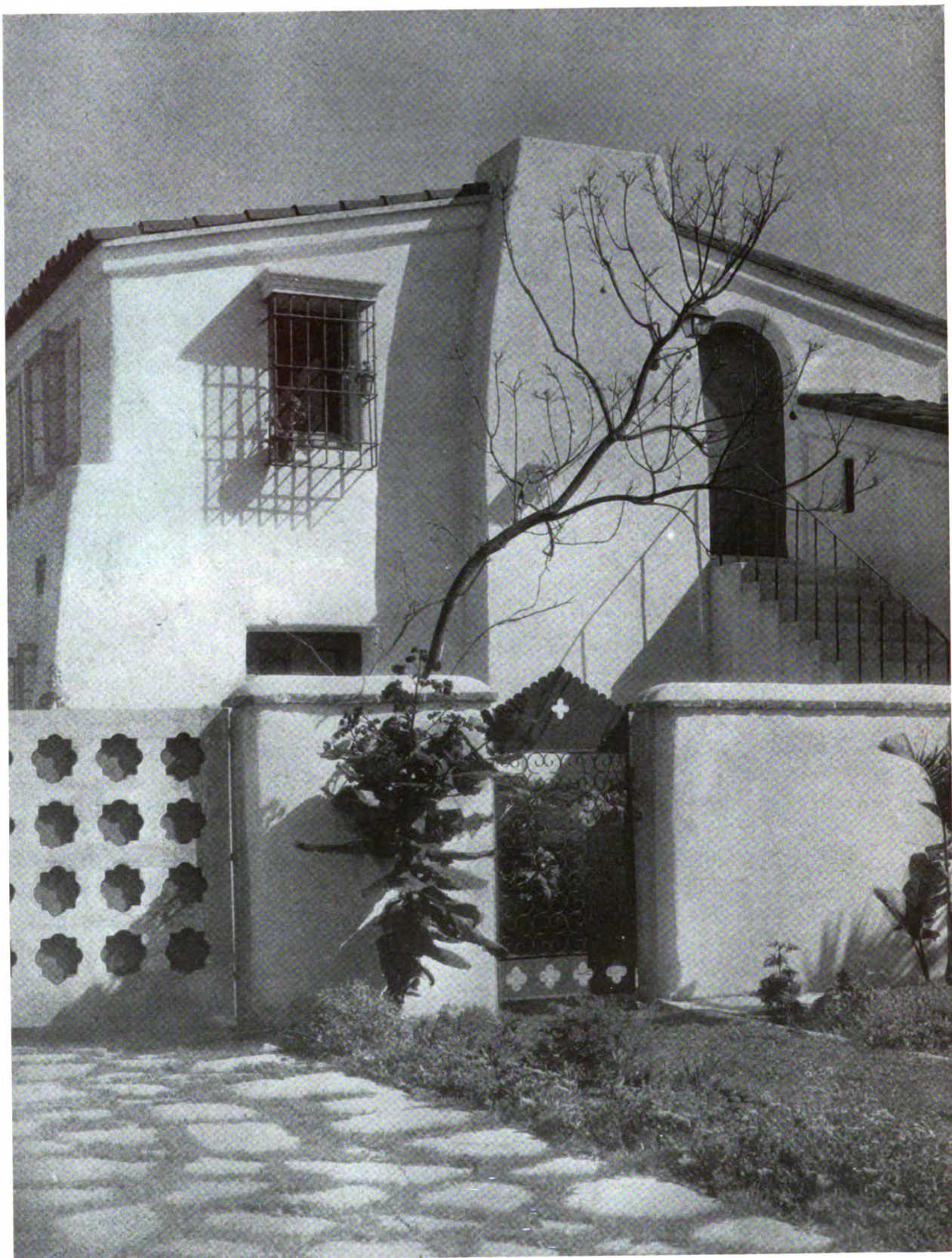
RESIDENCE OF MRS. H. M. GORHAM, SANTA MONICA, CALIFORNIA JOHN BYERS, ARCHITECT
