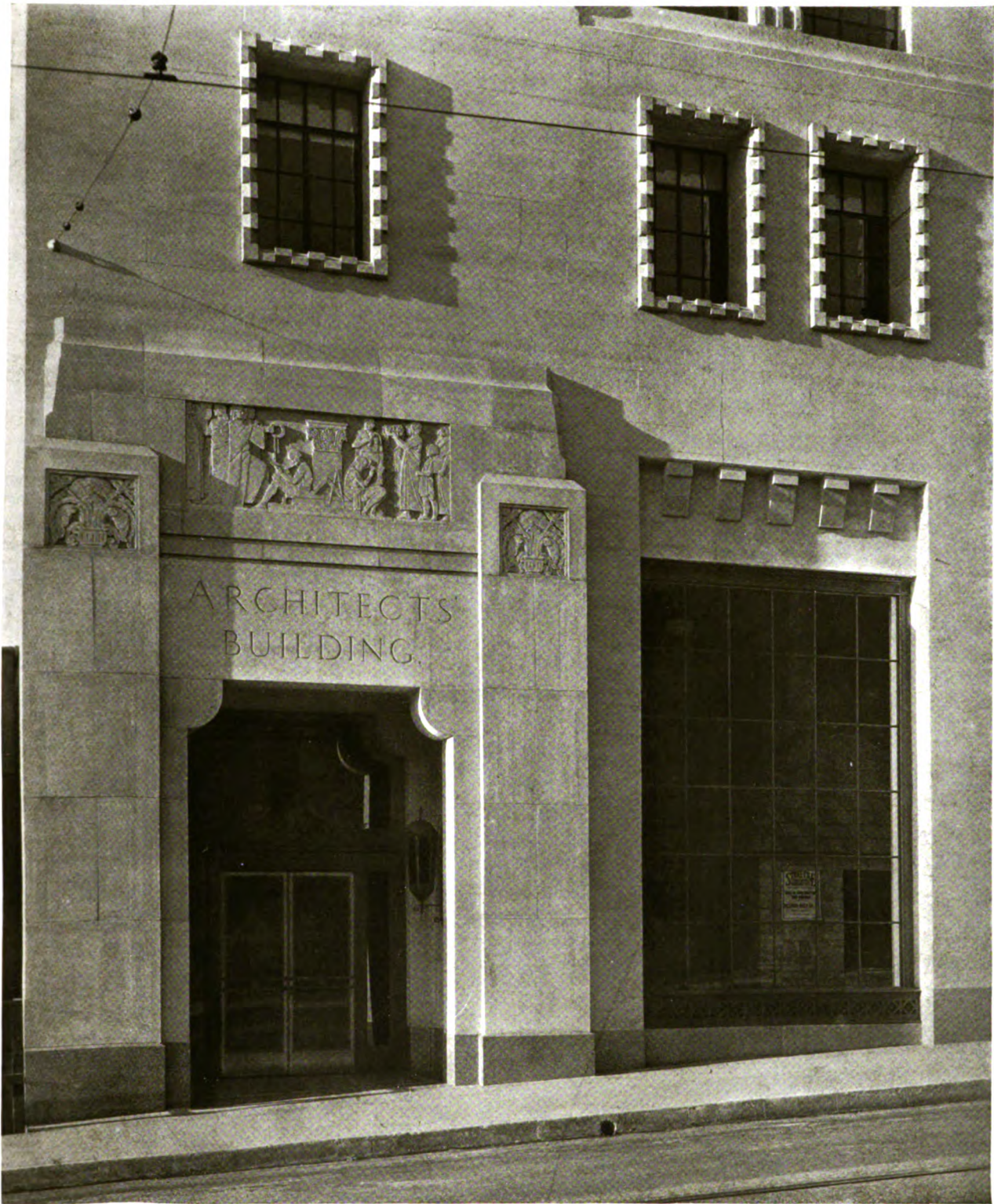
ENTRANCE DETAIL ARCHITECTS' BUILDING, LOS ANGELES, CALIFORNIA
