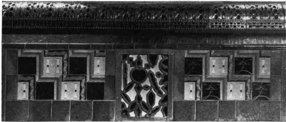
PERFORATED RADIATOR GRILLE. AMERICAN ENCAUSTIC TILING BUILDING, NEW YORK, N. Y.
