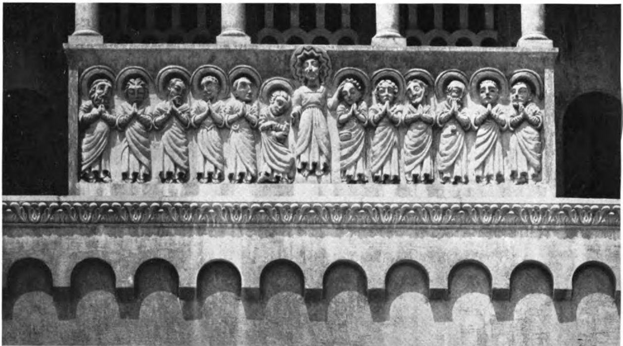
CONCRETE PANEL OVER PORCH—SCULPTURE BY ROBERT HOWARD FIRST CONGREGATIONAL CHURCH, OAKLAND, CALIFORNIA JOHN GALEN HOWARD AND ASSOCIATES, ARCHITECTS
