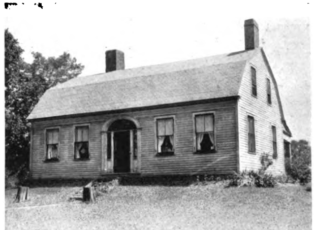
THE HORSFORD-LEE HOUSE, IS ANOTHER OF THE INTERESTING TYPES TO BE FOUND IN HUDSON. IT IS MODELED AFTER THE GAMBREL-ROOFED HOUSES OF NEW ENGLAND
