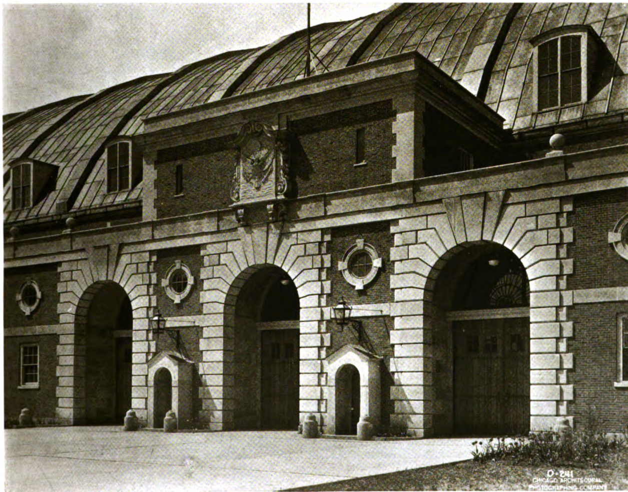
DETAIL—ARMORY UNIVERSITY OF ILLINOIS, URBANA, ILL.
