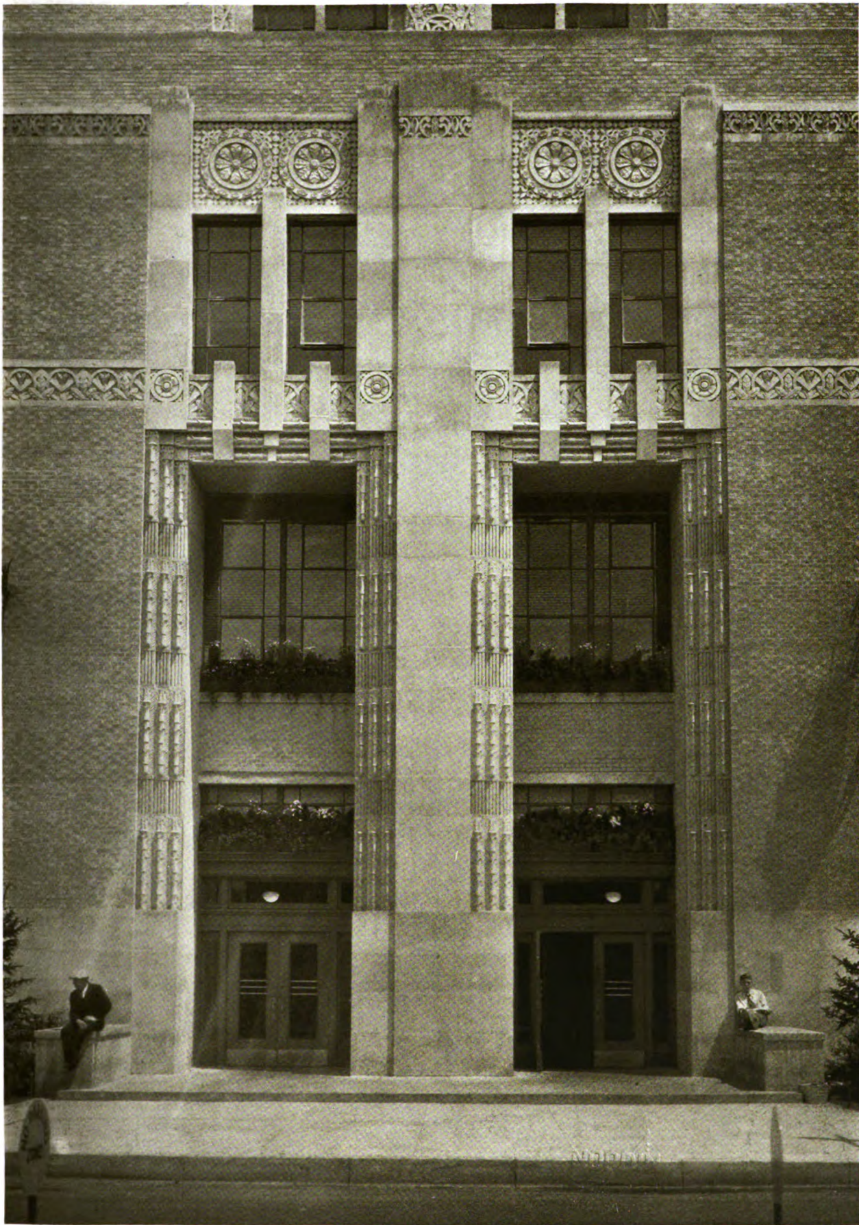
ENTRANCE DETAIL SEARS, ROEBUCK & CO. MAIL ORDER STORE, MINNEAPOLIS, MINN. NIMMONS, CARR & WRIGHT, ARCHITECTS :: :: :: :: ::
