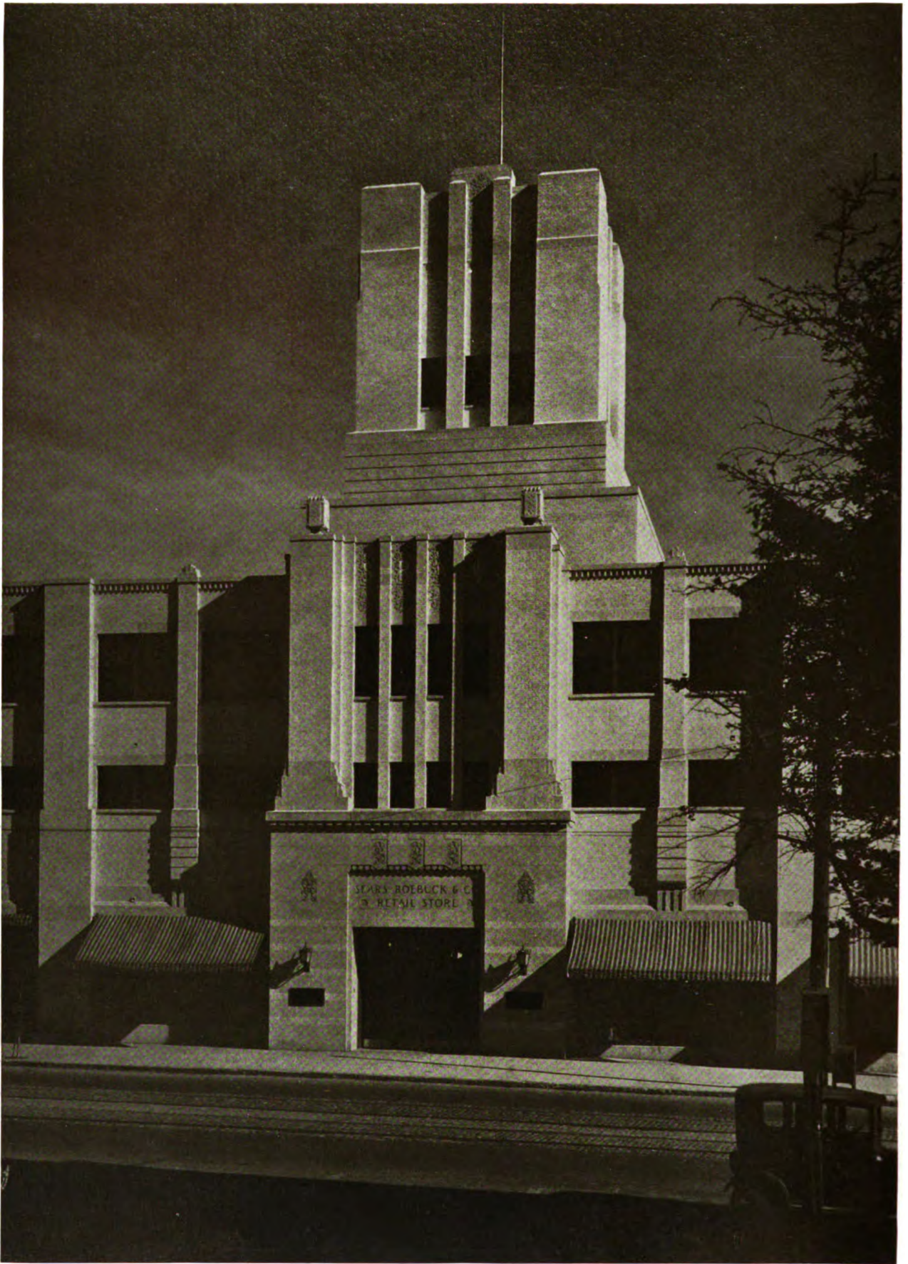
SEARS, ROEBUCK & CO. RETAIL STORE, BOSTON, MASS. NIMMONS, CARR & WRIGHT, ARCHITECTS :: :: ::
