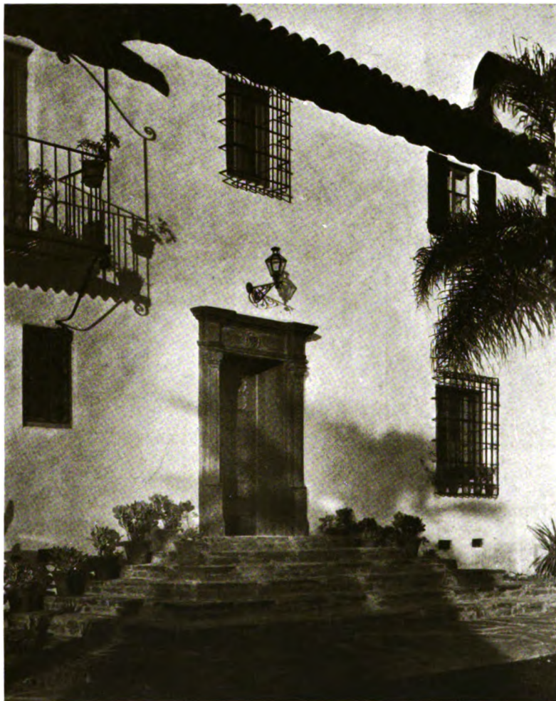
ENTRANCE DETAIL RESIDENCE OF MR. HUNTER S. ROBBINS, FLINTRIDGE, CALIFORNIA JOHN BYERS, ARCHITECT :: :: :: :: :: :: :: :: :: ::
