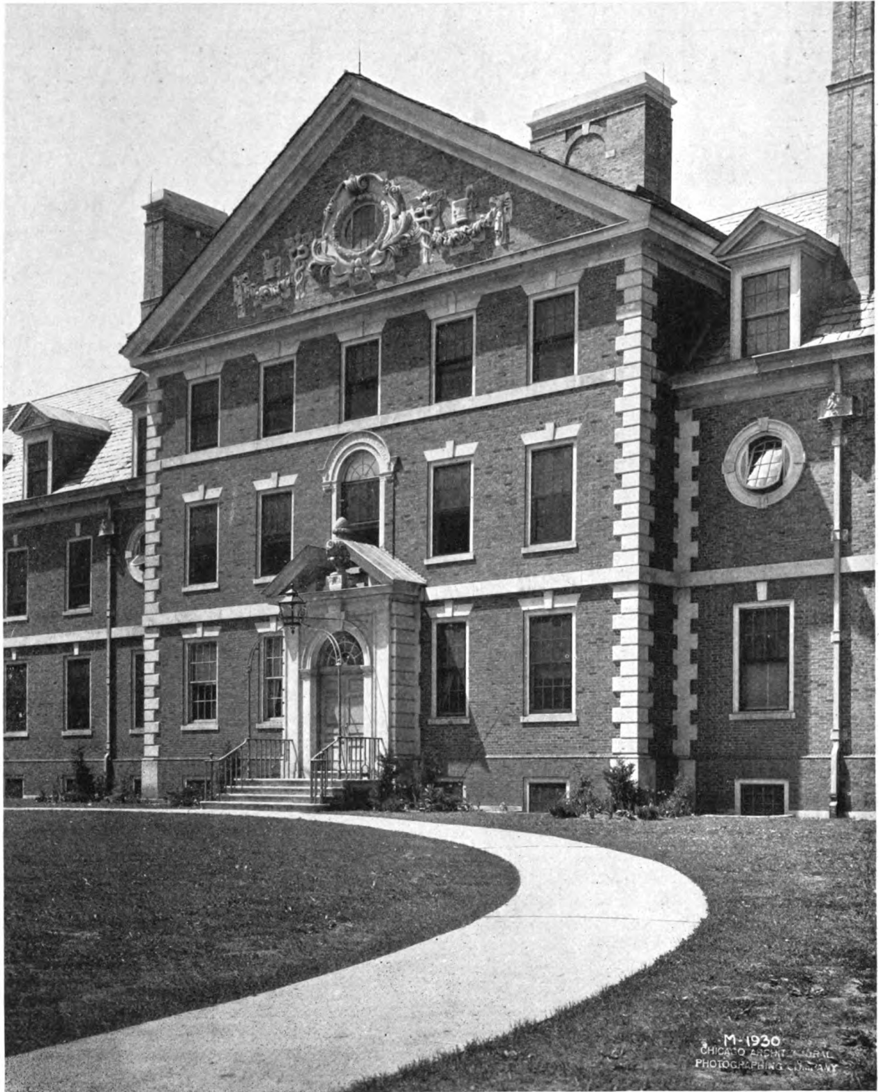
McKINLEY MEMORIAL HOSPITAL UNIVERSITY OF ILLINOIS, URBANA, ILL. CHARLES A. PLATT AND JAMES M. WHITE, ASSOCIATED ARCHITECTS
