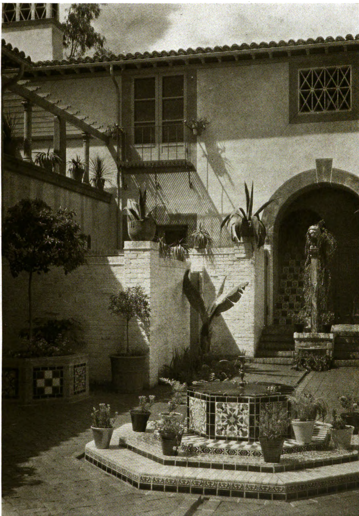
COURT OF THE FOUNTAIN RESIDENCE (APARTMENT) AT 1355 N. LAUREL AVE., LOS ANGELES, CALIFORNIA PIERPONT & WALTER DAVIS, ARCHITECTS
