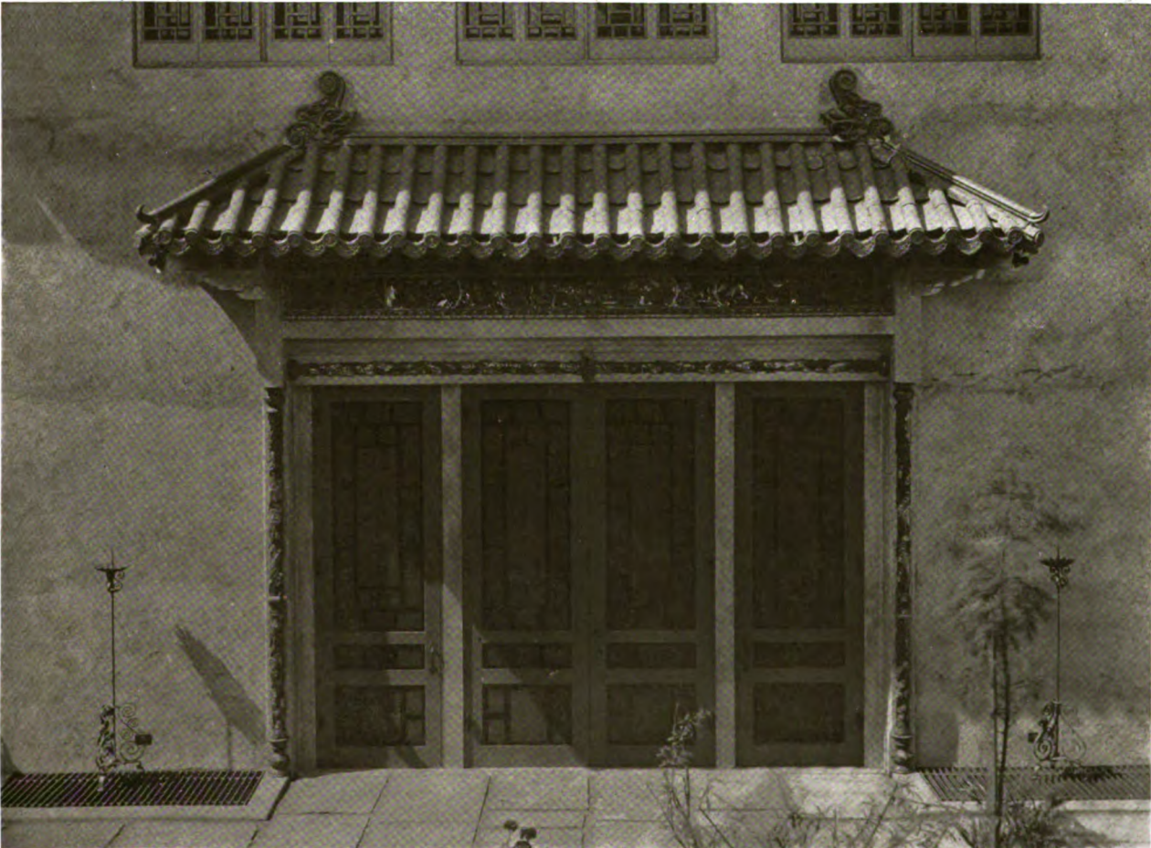
DOORWAY IN CHINESE COURT—GRACE NICHOLSON'S TREASURE HOUSE, PASADENA, CALIFORNIA MARSTON, VAN PELT & MAYBURY, ARCHITECTS
