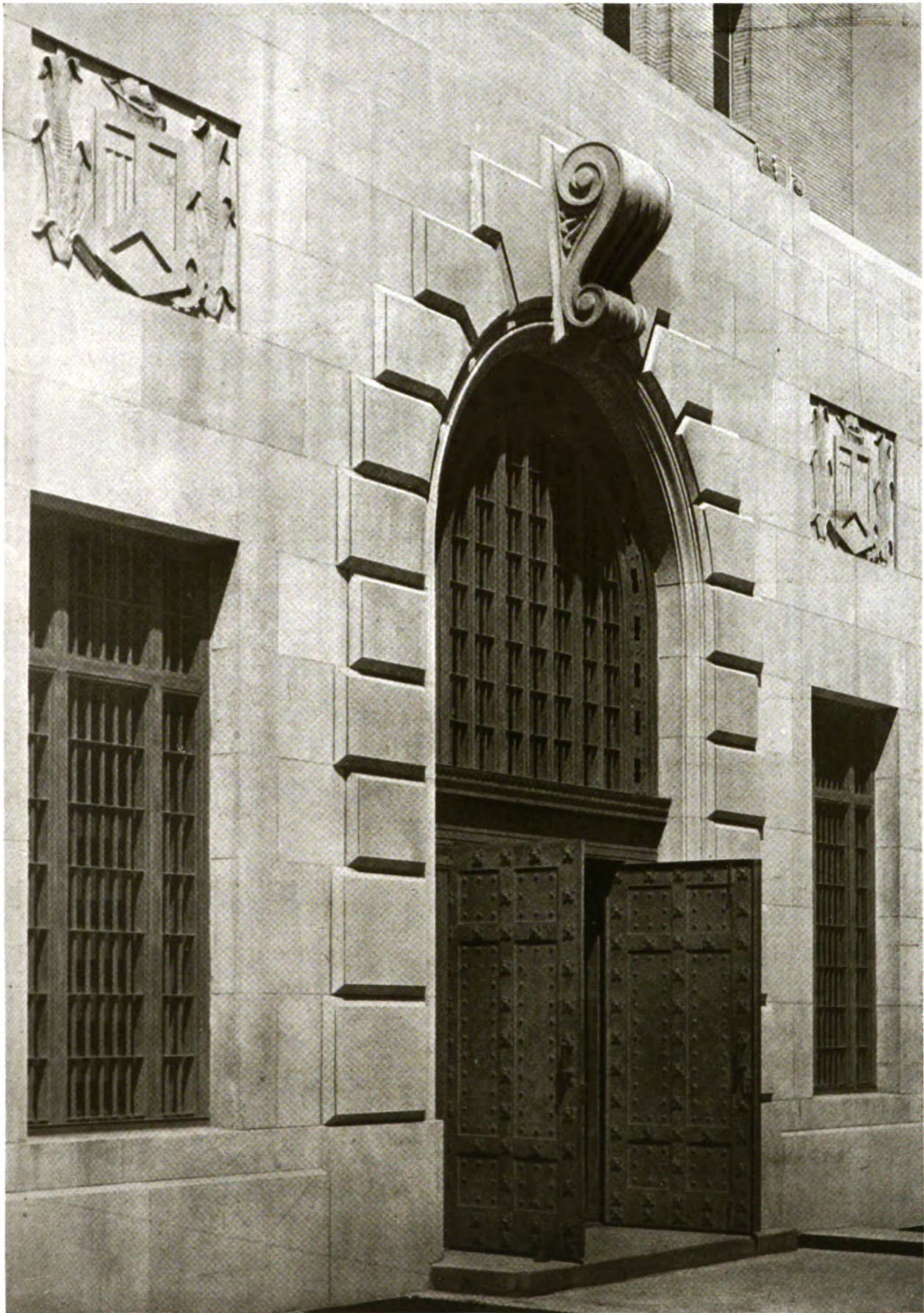
DETAIL, JAIL ENTRANCE COOK COUNTY JAIL, CHICAGO ERIC E. HALL, COUNTY ARCHITECT OF HALL, LAWRENCE & RATCLIFFE, INC.
