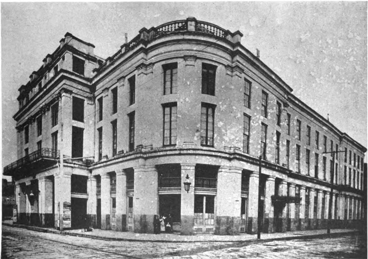
THE FRENCH OPERA, NEW ORLEANS, JAMES GALLIER, JR., ARCHITECT
