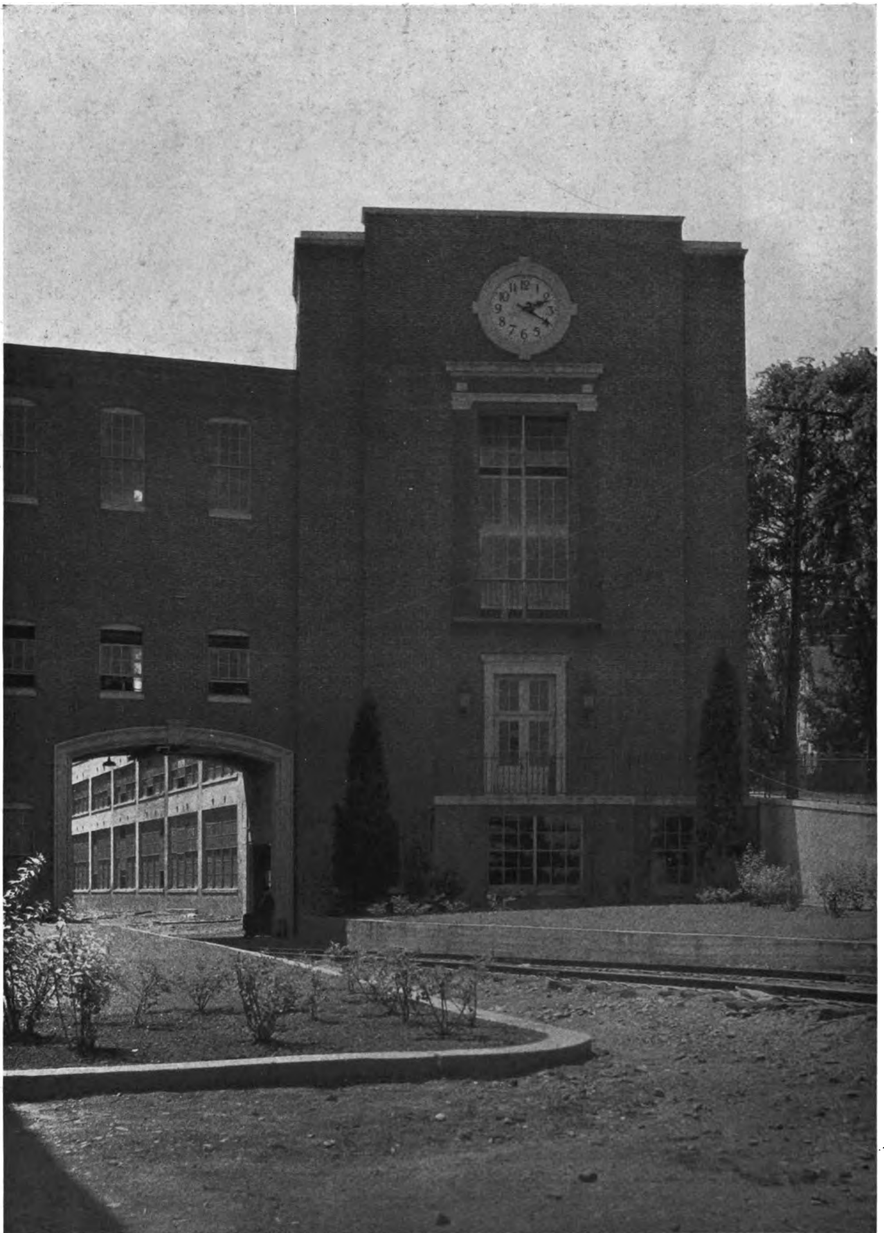
END PAVILION, FACTORY NO. 14 WHITIN MACHINE WORKS, WHITINSVILLE, MASS. J. D. LELAND & CO., ARCHITECTS :: :: ::
