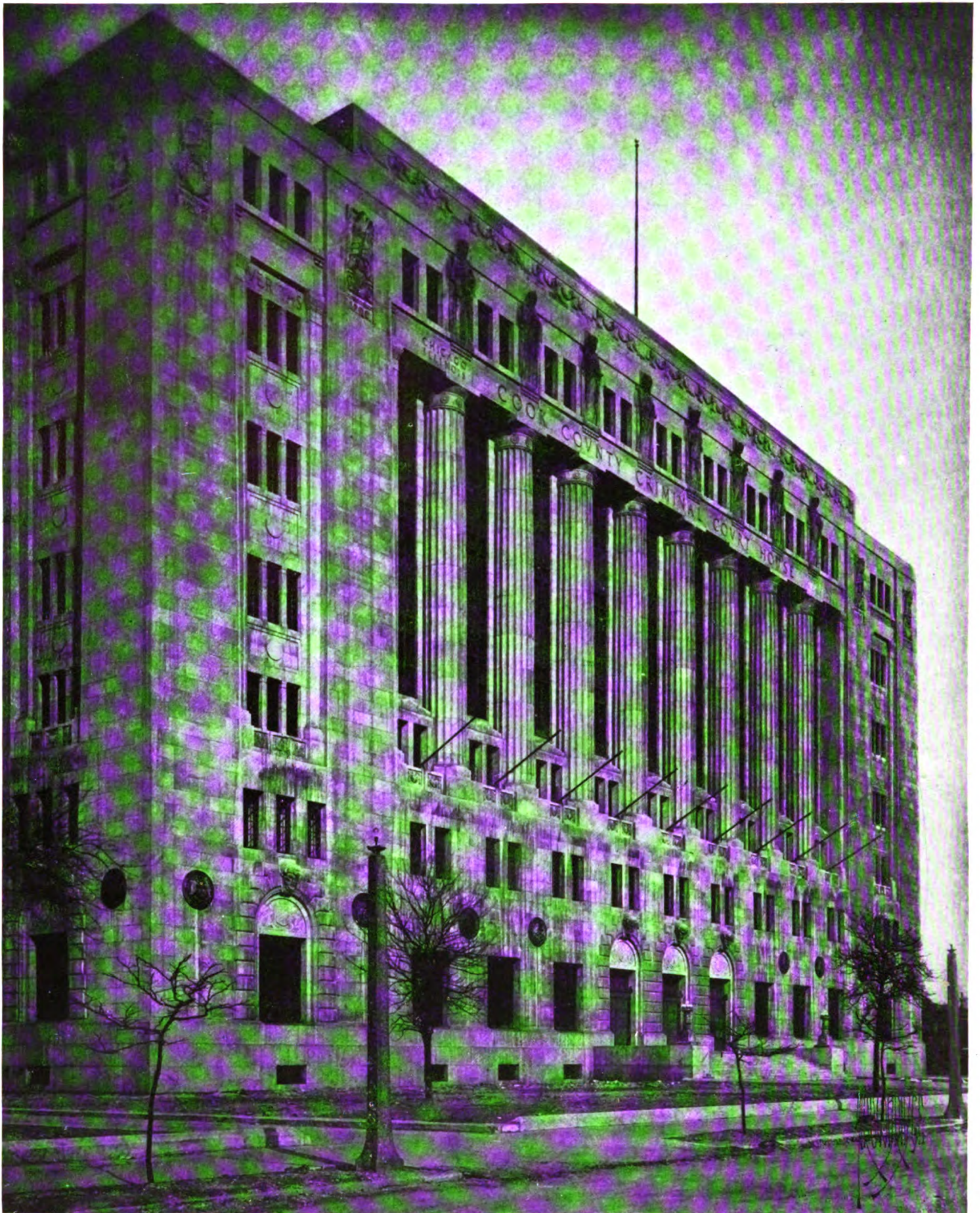
COOK COUNTY CRIMINAL COURT HOUSE, CHICAGO ERIC E. HALL, ARCHITECT, OF HALL, LAWRENCE & RATCLIFFE, INC.
