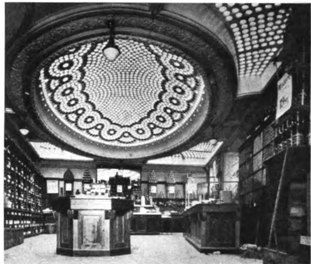
FIG. 8—GLASS-STONE FERRO-CONCRETE CEILING IN PARIS STORE.
