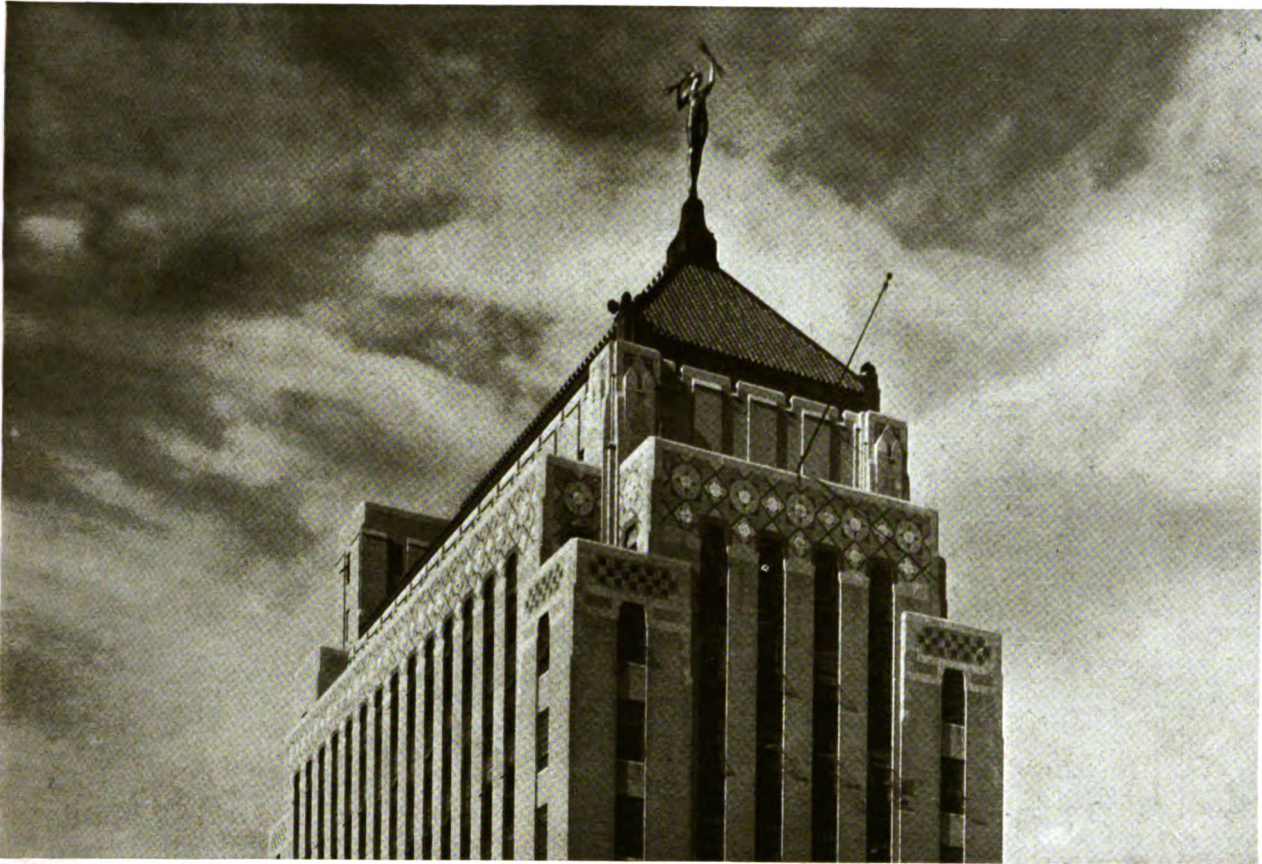
DETAIL ALABAMA POWER COMPANY BUILDING, BIRMINGHAM, ALABAMA COURTESY ASSOCIATED TILE MANUFACTURERS
