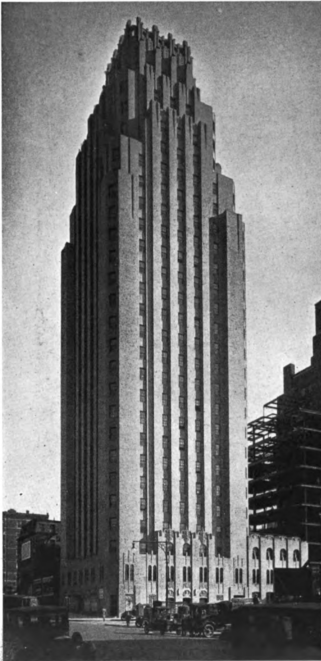
THE PAN-HELLENIC BUILDING, NEW YORK, N. Y. JOHN MEAD HOWELLS, ARCHITECT
