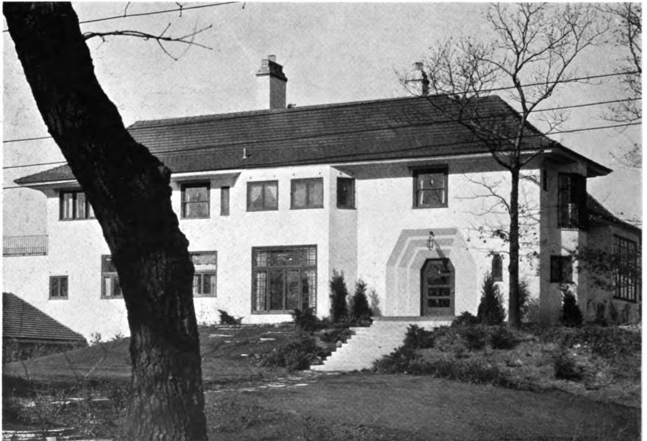
Southeast View of Main Entrance
