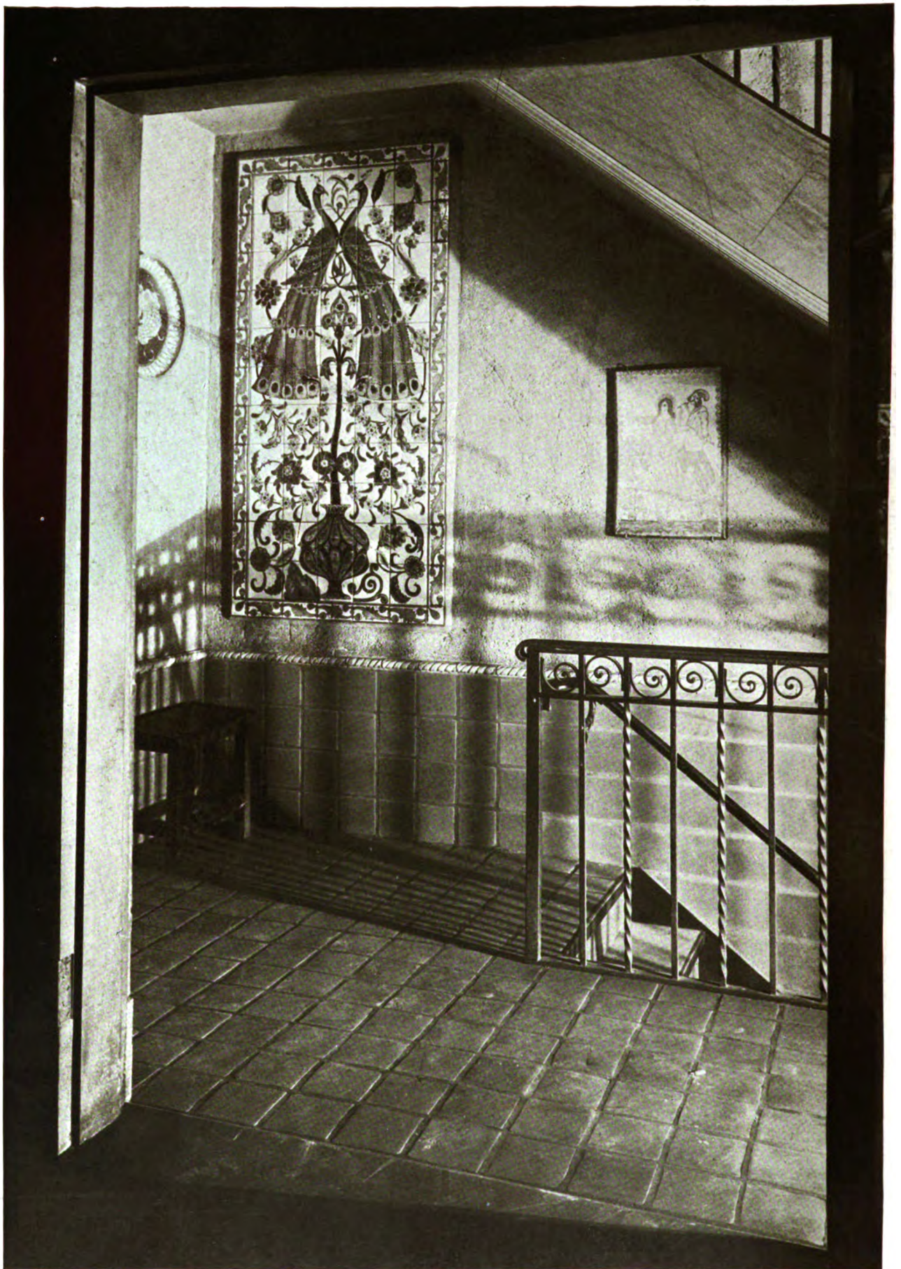
STAIR DETAIL AMERICAN ENCAUSTIC TILING BUILDING, NEW YORK, N. Y. COURTESY AMERICAN ENCAUSTIC TILING CO. :: :: :: ::
