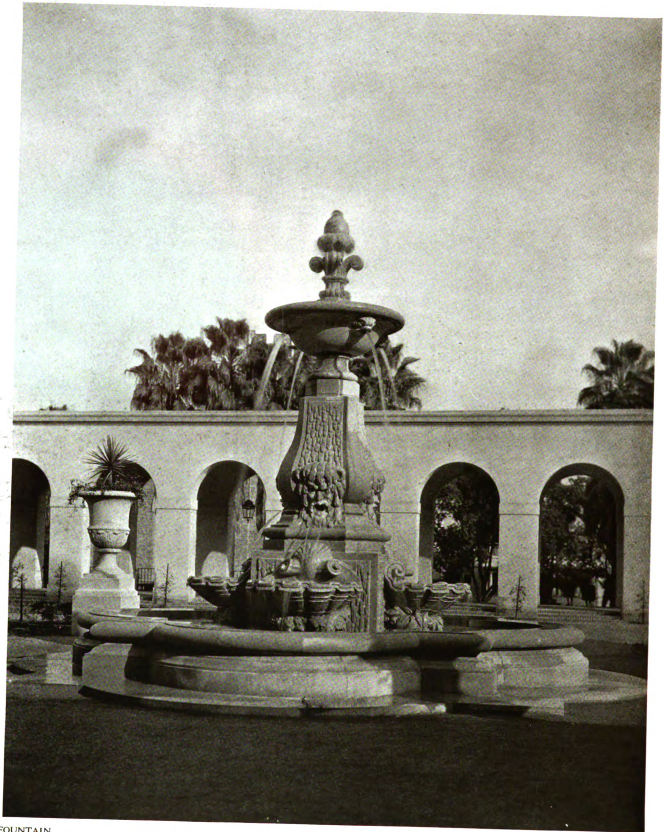
FOUNTAIN PASADENA CITY HALL, PASADENA, CALIFORNIA BAKEWELL AND BROWN, ARCHITECTS :: ::
