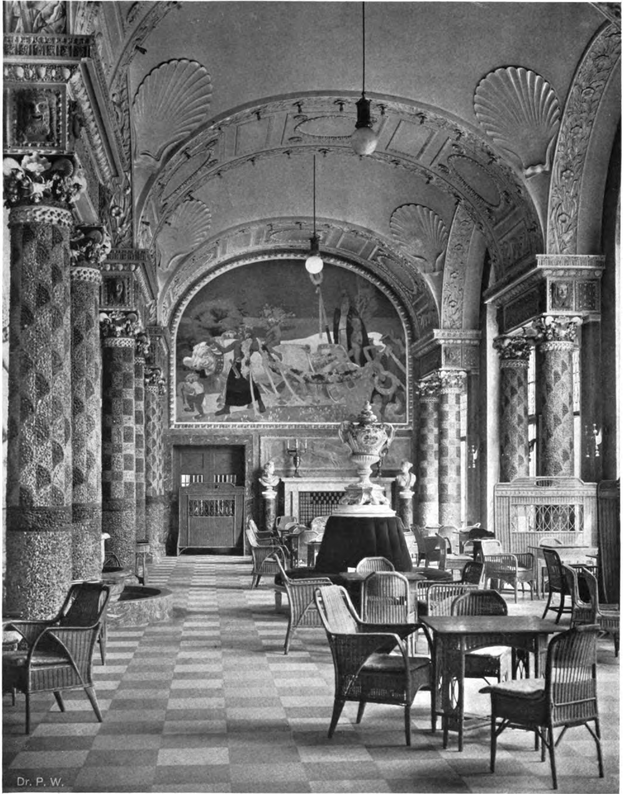
FIG. 14—CONCRETE COLUMNS IN THE HALL OF SHELLS, KURHAUS, WIESBADEN, GERMANY. SHELLS ARE CEMENTED TO THE CONCRETE CAPITALS AND PEBBLES FASTENED WITH CEMENT ON THE CONCRETE SHAFTS.
