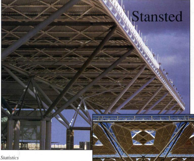
Total area covered by roof 39,204 sq.m. Total weight of steel structure 3,022 tonnes comprising 2,268 tonnes of tubular sections (69,000 lin.m), 490 tonnes of plates and 264 tonnes of castings.
