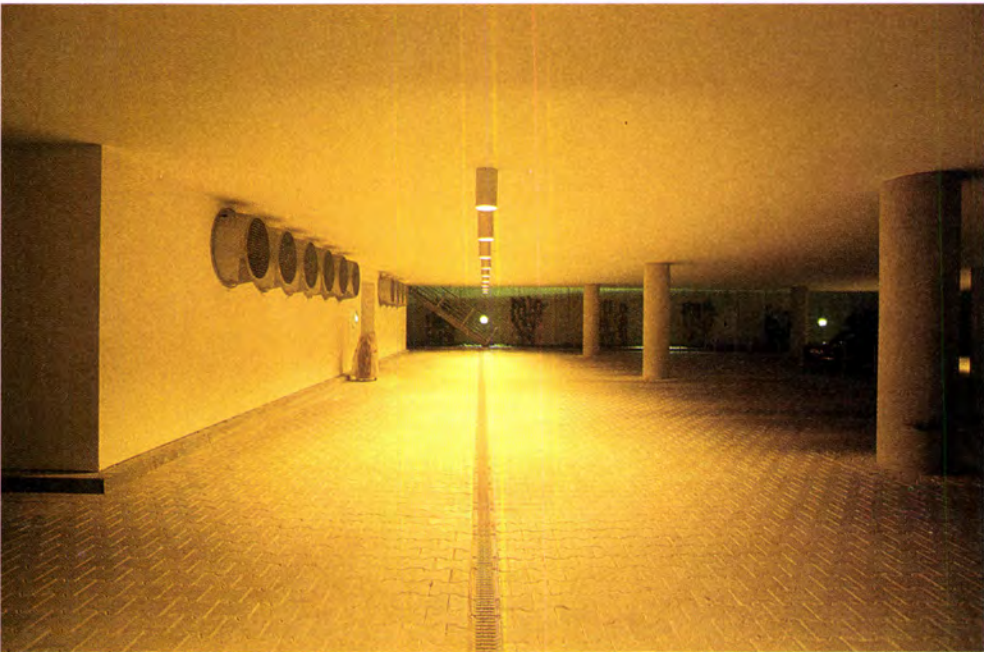
Garages; mounted downlights for sodium high pressure lamps 50 W; median illumination intensity 50 lux; median specific connect load 2 W/m 2 .
