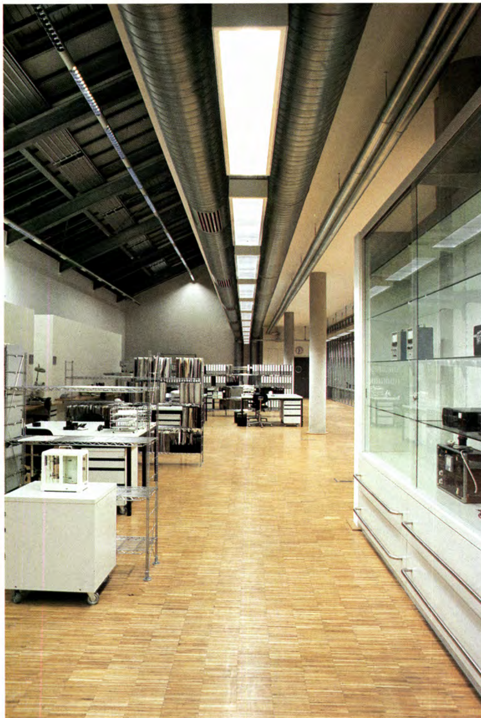
Laboratory and manufacturing area: Visionair darklight lamps for fluorescent lights 58 W, neutral white colour, median illumination intensity 750 lux; specific connect load 16 W/m
