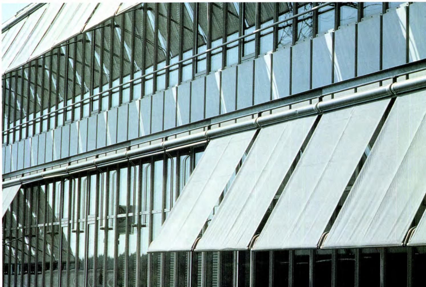
Sun protection on vertical windows is provided by exterior textile blinds together with interior variable horizontal lamella.
