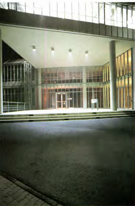
Entrance area outside: zonal illumination with downlights for mercury high-pressure lamps, HME 125 W, light colour off white. Revolving entrance door: downlights for low voltage halogen bulbs there are 8 \times 20 W.
