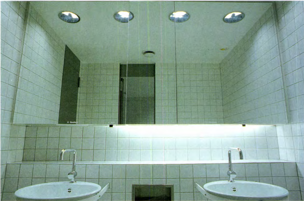
Subsidiary rooms and corridors; downlights for compact fluorescent lamps TC 2 × 9 W, neutral white colour; median specific connect load 5 W/m 2 .
