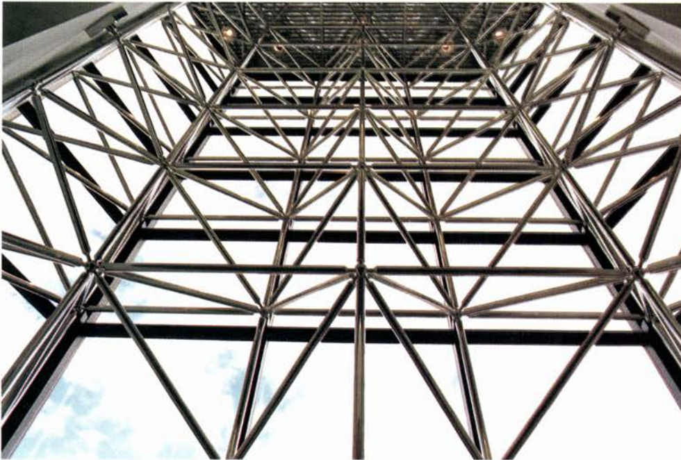
Above and right: A spaceframe used as a component part of a building – "The Triad Center", Gulph Mills, Pennsylvania (Arch. Rhett Hamilton Jones Associates)
