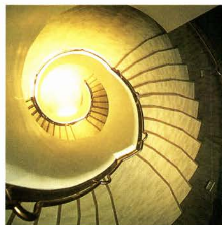
The main central staircase, its spiral form echoing the plan of the library itself.
