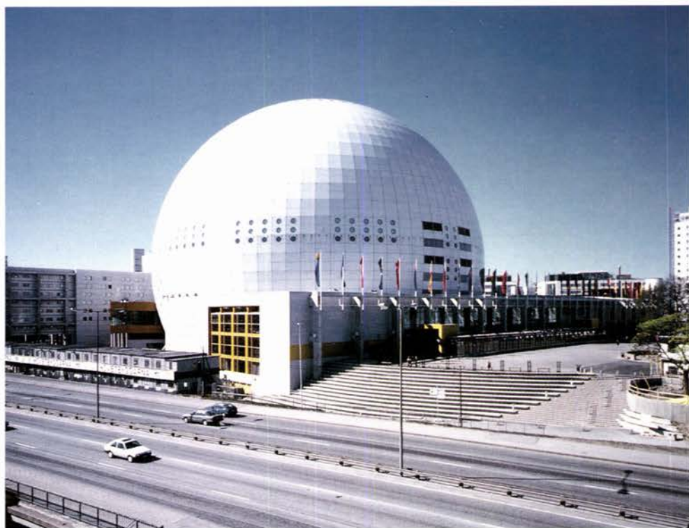
Opposite and above: A spaceframe used as the structure of a building – the dome of the “Sport and Culture Centre”, Stockholm, Sweden
