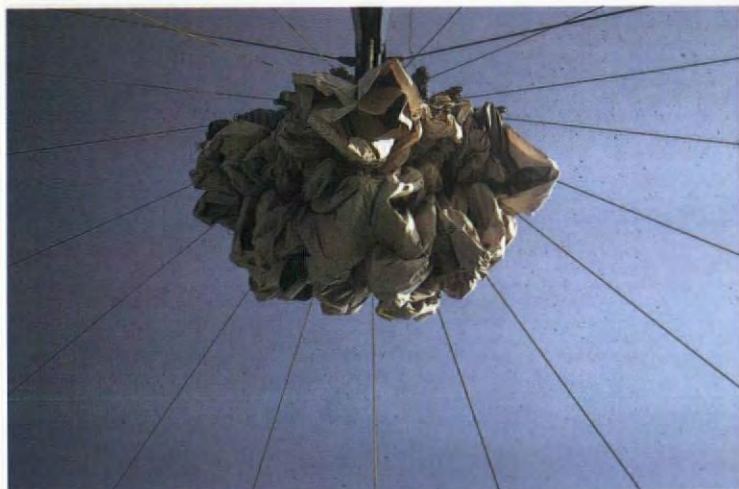
Below and black and white sequence: PVC retractable roofing over a swimming pool, Düsseldorf, West Germany. Architect: Dyckerhoff & Widmann. Consultant engineer and implementation: IPL. Area covered: 1,900 m 2 .
