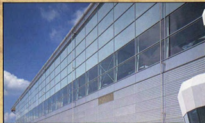
STANSTED AIRPORT - CURTAIN WALLING AND CLADDING BY SCHMIDLIN
