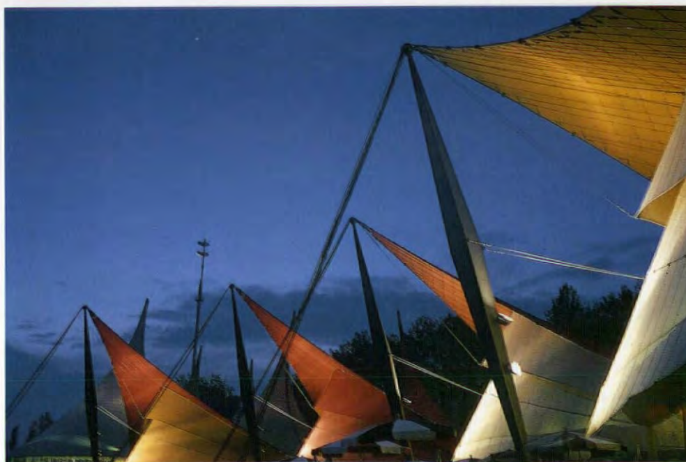
EXPO '64, Lausanne, Switzerland. Mechanically tensioned sails supported by ridge and boundary cables. Architect: Saugey. Consultant engineer and implementation: L. Stromeyer & Co.
