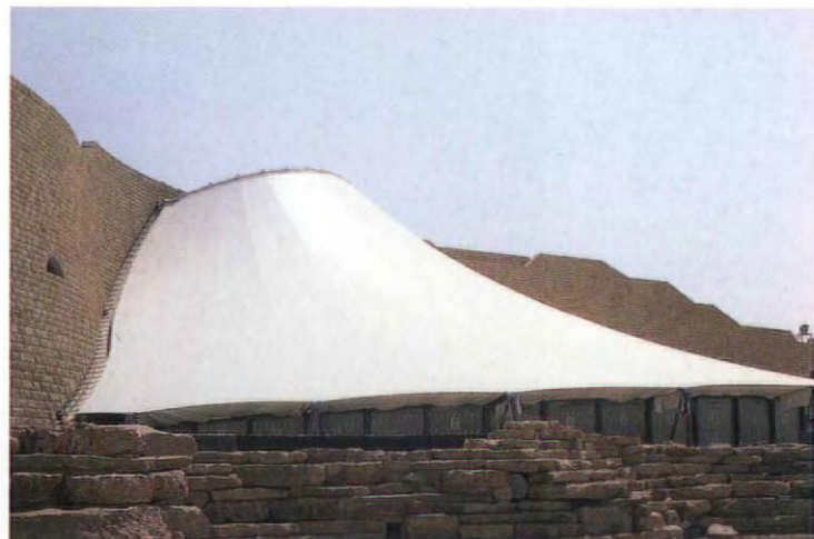
Above and right: Diplomatic Club, Riyadh, Saudi Arabia. Interior and exterior views of double skin PTFE-Fibreglass structure. Architect: Omeria/Otto. Consultant engineer: Happold Bath. Implementation: IPL.
