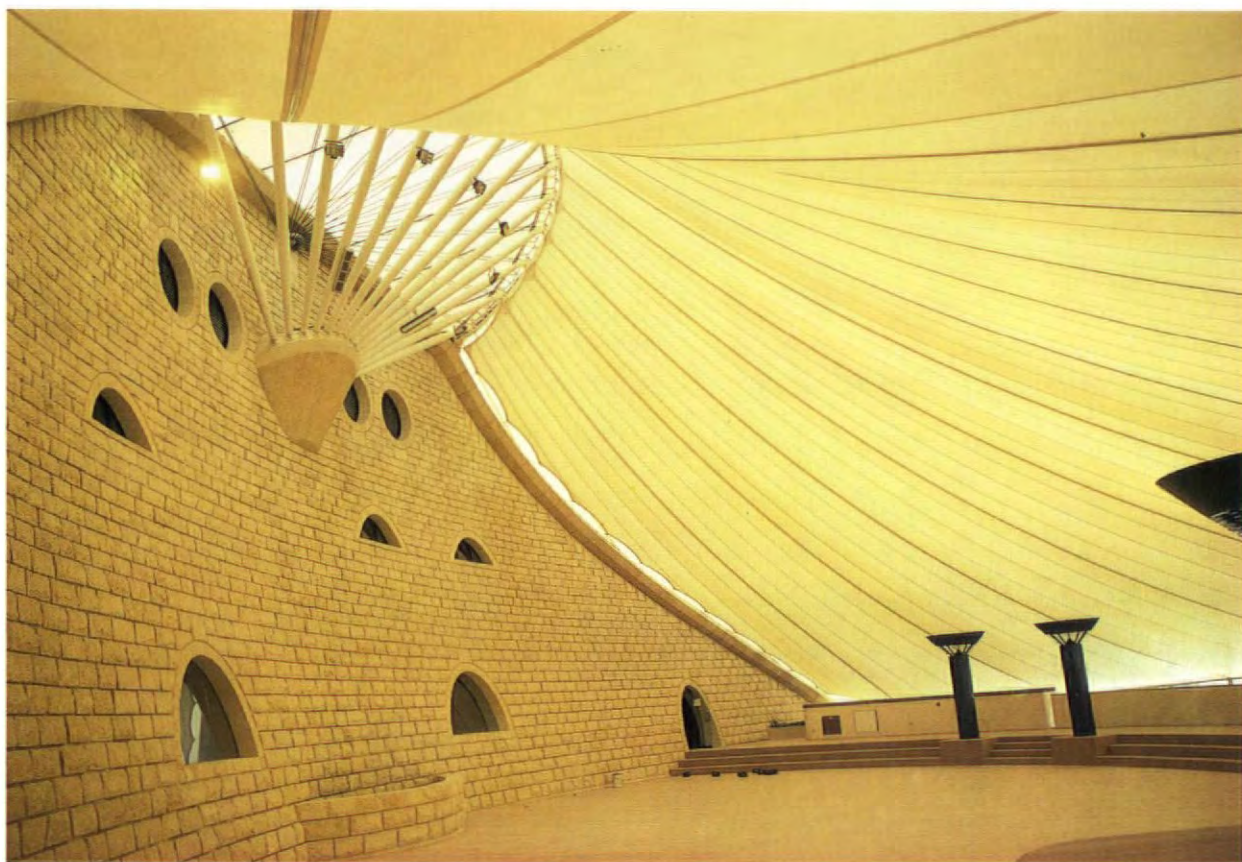
Above and right: Diplomatic Club, Riyadh, Saudi Arabia. Interior and exterior views of double skin PTFE-Fibreglass structure. Architect: Omeria/Otto. Consultant engineer: Happold Bath. Implementation: IPL.
