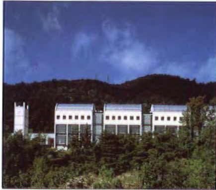
Kobe Institute, Kobe - Arup has worked with architect Troughton McAslan Limited and Takenaka on the design of structures and building services of new and refurbished buildings for the post-graduate college
