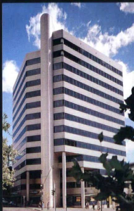
S.T.A. Office Building, Adelaide/Australia
