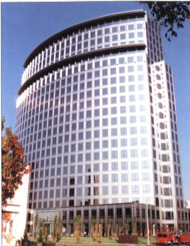
Plaza Tower 600 Anton Boulevard Costa Mesa, California
