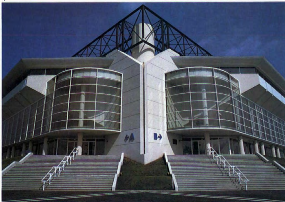
1 and 2 Esso House corporate headquarters at Leatherhead, Surrey, UK. Architects Percy Thomas Partnership specified Formawall 1000 flat insulate composite panels for the curtain wall system. The crisp, silver-grey cladding panels have a solar reflective finish. Supplier: H H Robertson (UK), Cromwell Road,
