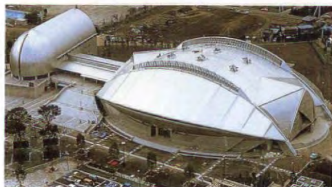
Fujisawa municipal gymnasium
