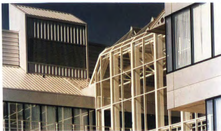
Esso building, near Leatherhead, UK, designed by Percy Thomas Partnership: creative use of composite metal panels on a prestige building.
