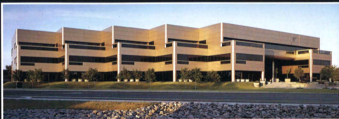
Biltmore Commerce Centre, Phoenix, Arizona/USA
