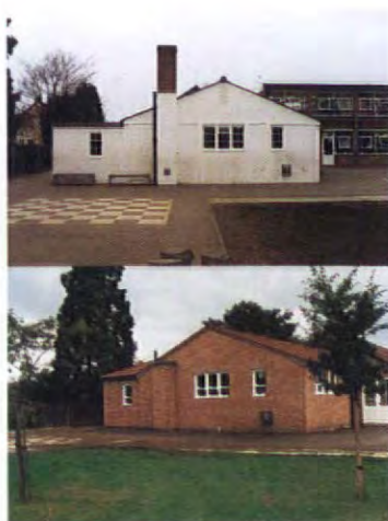
An example of over-cladding using an insulated brick cladding system from Eurobrick (above) at Ashford School, Middlesex. Circle #76.
