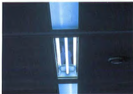
3M Silverlux™ reflectors (right) are a new concept in lighting which contain a silver reflective film which assures 95% reflectivity. Through replacement of 'TL' luminaire with a 'Silverlux' model containing only half the original number of lamps, it is possible to achieve the same level of light output using half the electricity. Circle #73.
