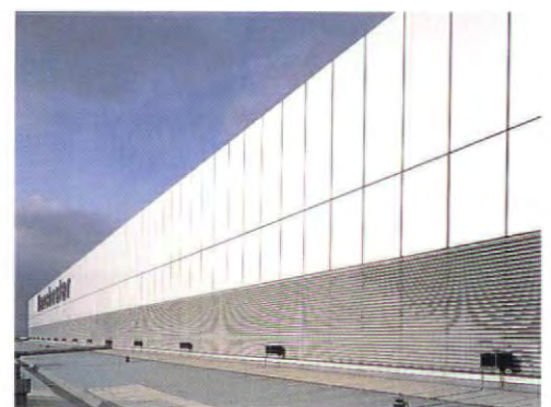
Manchester Airport's Terminal 2 features cladding from Felix Constructions SA, specified for its high level of noise reduction, thermal performance and optimum protection for the comfort of those inside the terminal
