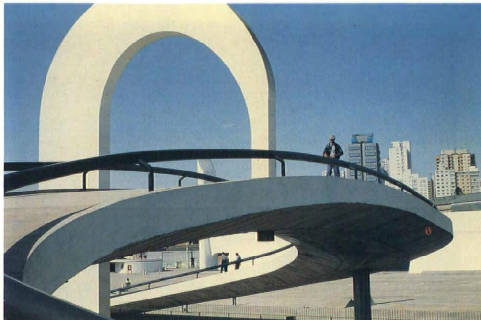
The concrete pedestrian bridge (above) crossing the motorway with its expressive curving support
