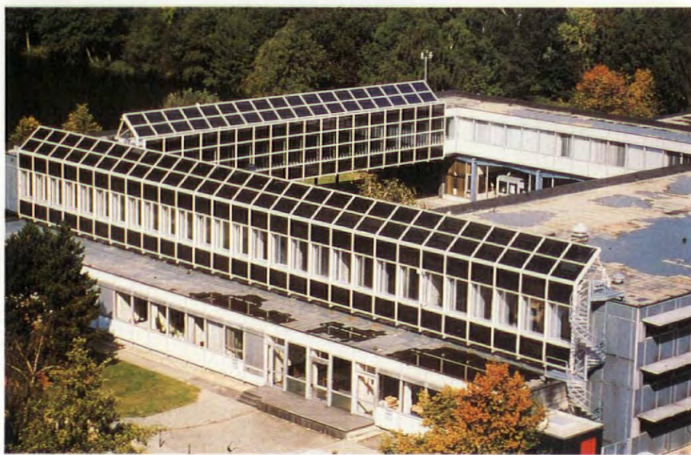
Central library of the research centre KFA Jülich: The solar modules have been integrated into the curtain wall.
