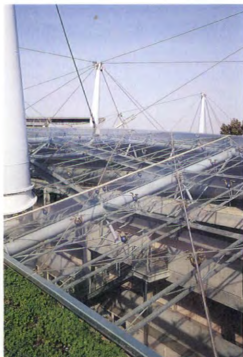
Junction of undulating grass roof and rooflights
