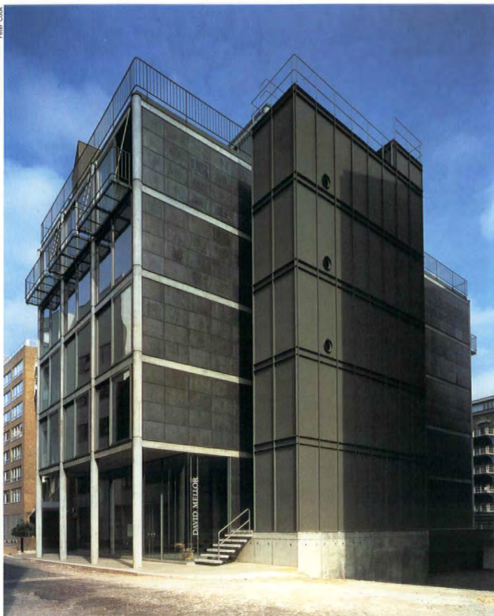
Building is set next to River Thames (left). Plans (above) show rational concrete framing and out-rigged lift tower
