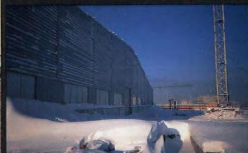
A sawmill built in Russian Siberia in collaboration with a Japanese company. 20,000 m 2 of Kvatro panels were used in the building which was designed to withstand temperatures down to -56°C.
