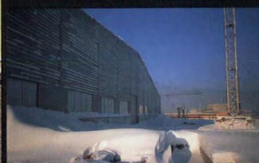
A sawmill built in Russian Siberia in collaboration with a Japanese company. 20,000 m 2 of Kvatro panels were used in the building which was designed to withstand temperatures down to -56°C.
