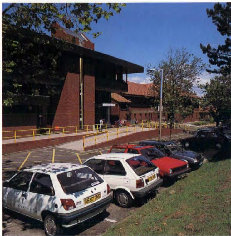
The short stay unit, Liverpool Cardiothoracic Centre (below left and right), mental illness unit Fazakerley Hospital, Liverpool (middle) and Park Lane Hospital, Liverpool (bottom)
